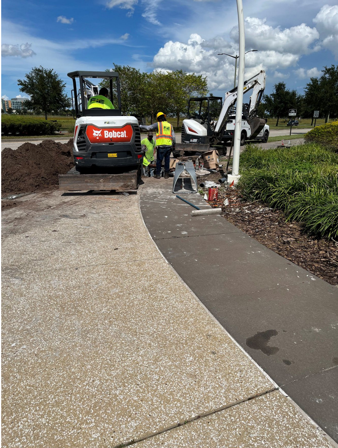
Photo 67 - Construction in Entrance at VA Hospital Intersection
