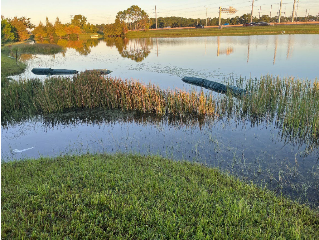
Photo 80 – Broken Floating Turbidity Barrier
