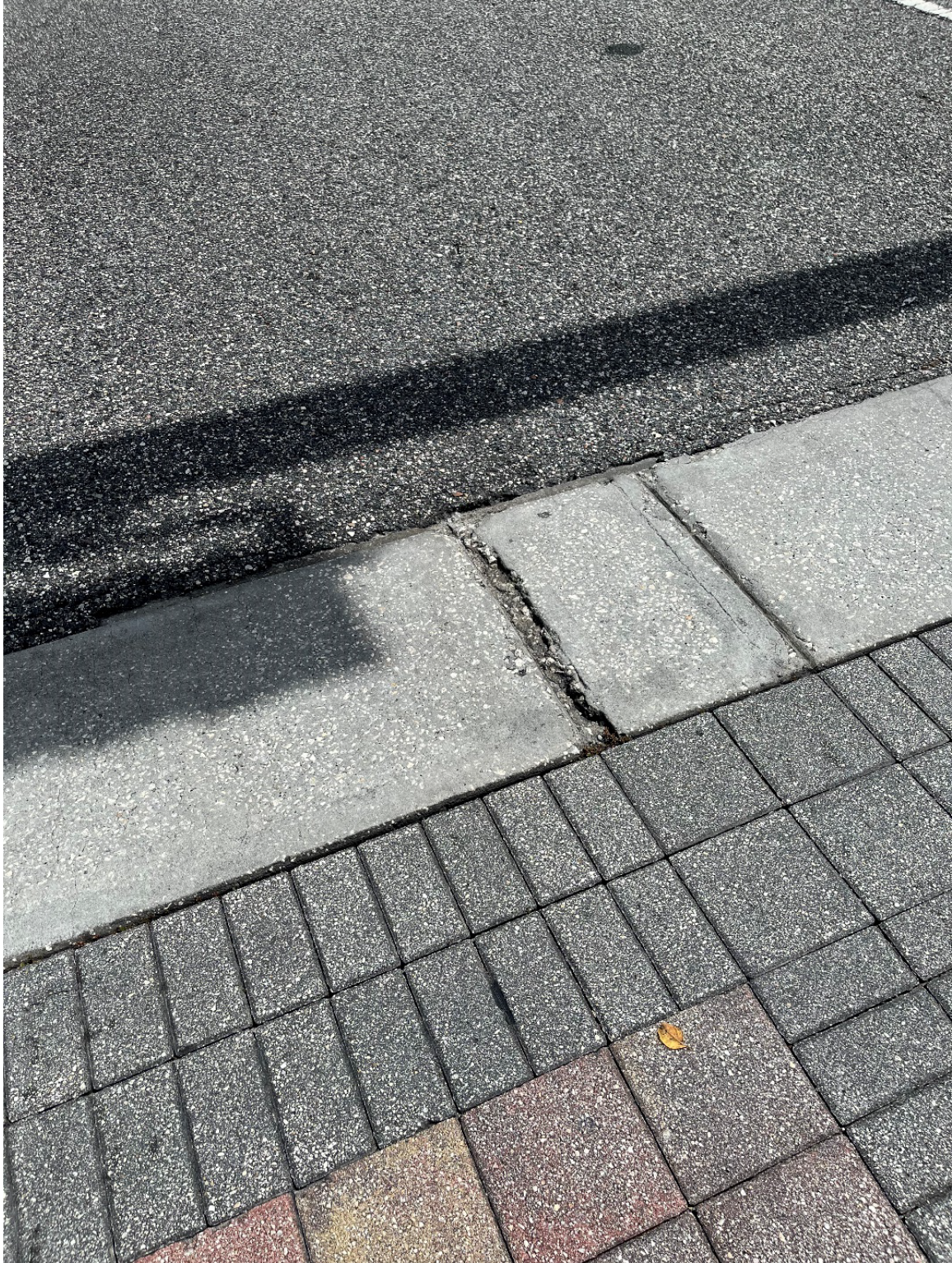
Photo 94 – Cracked Concrete - Minor Settling
