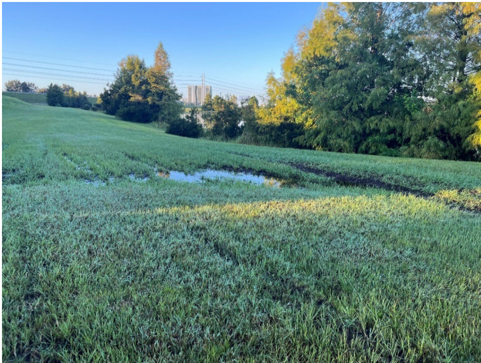
Photo 81 – Poor Drainage in NE Corner Berm
