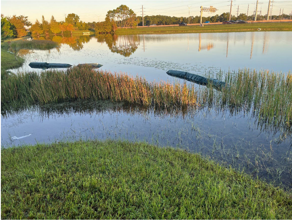
Photo 80 – Broken Floating Turbidity Barrier
