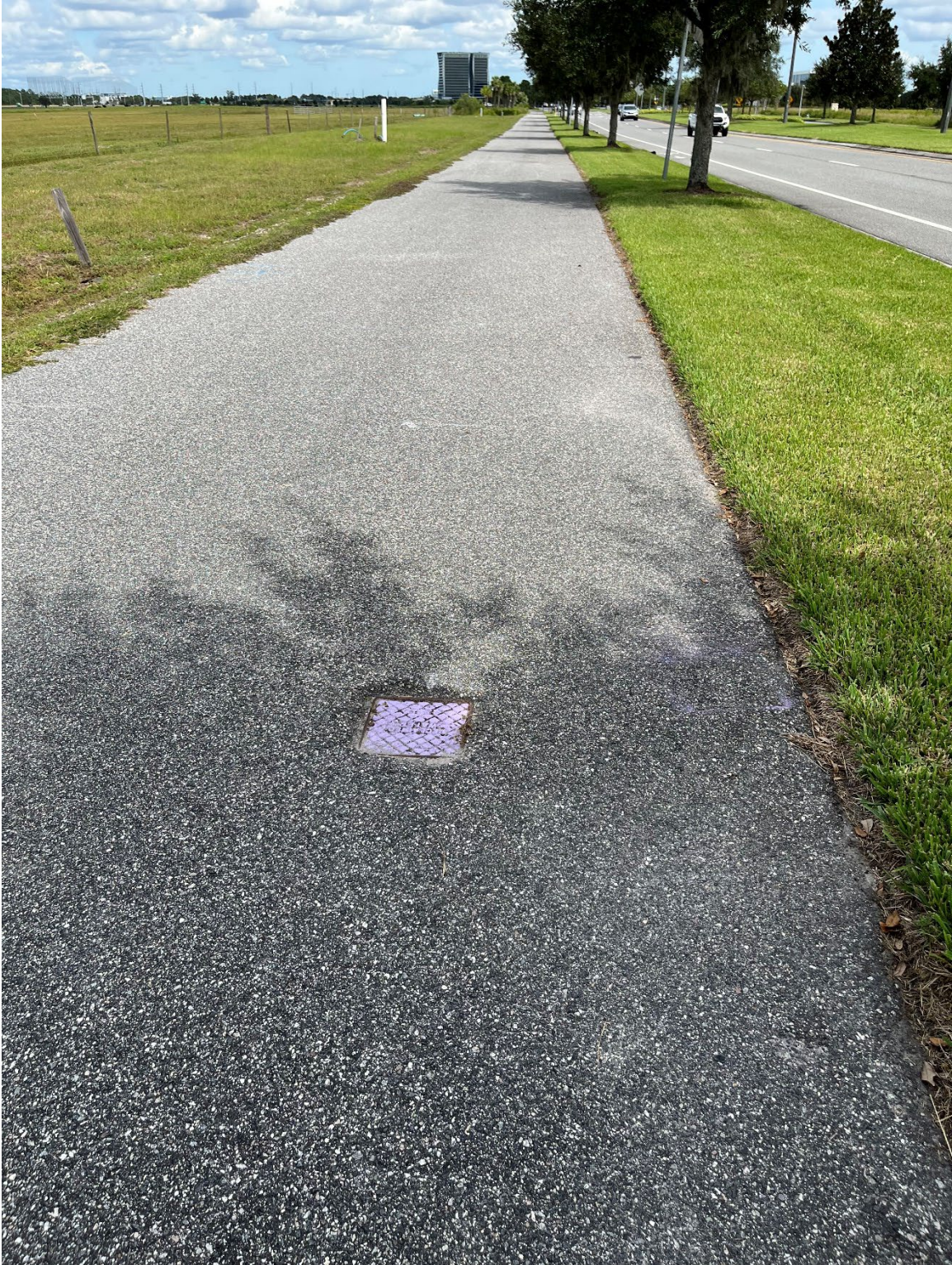
Photo 12 – Sunken Reclaim Water Meter
