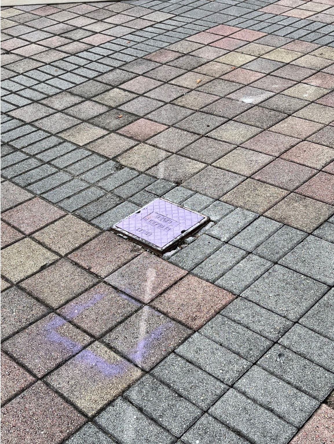
Photo 42 - Raised Reclaim Meter (Approximately 1/2 inch)
