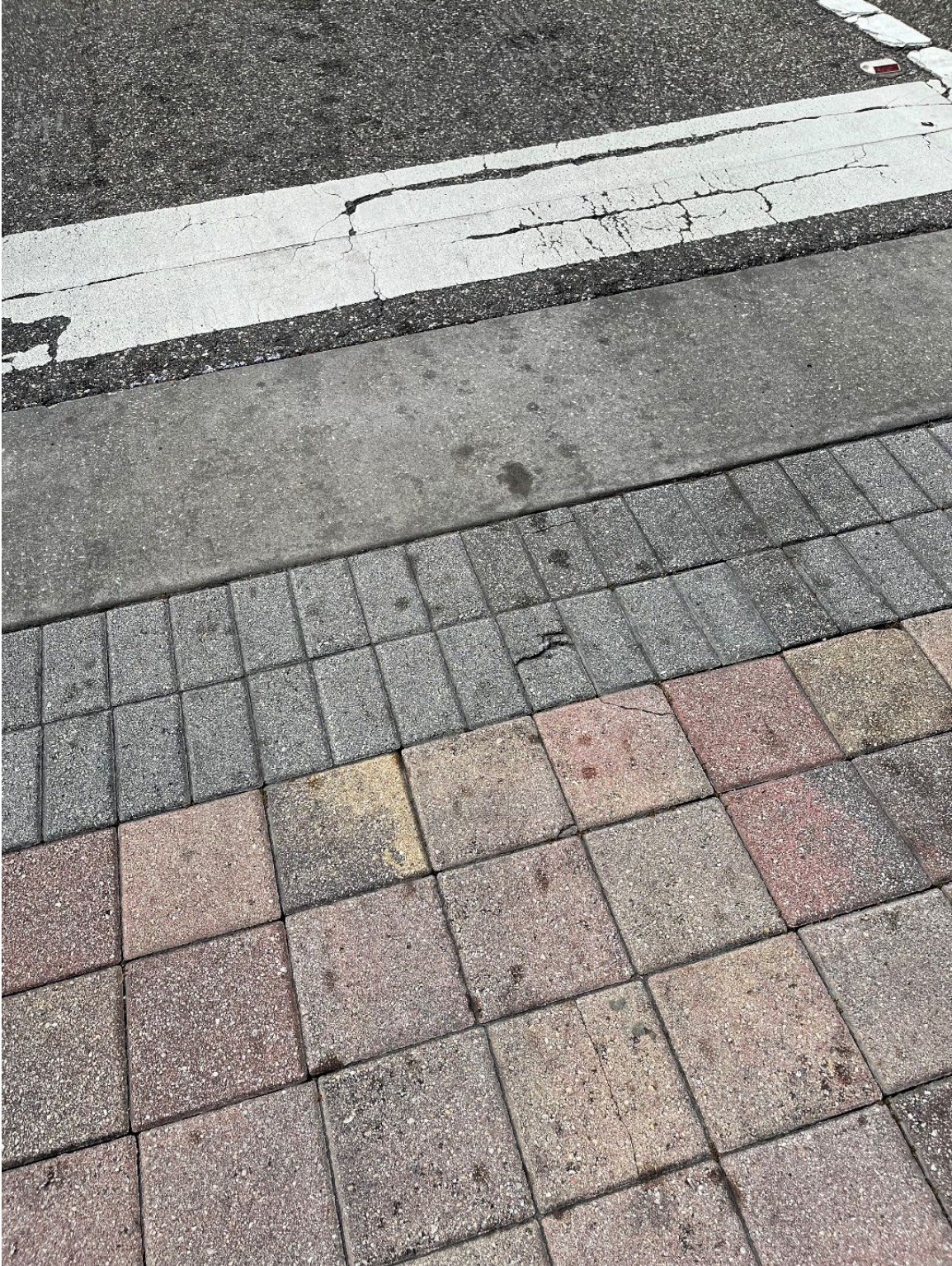
Photo 110 – Cracked Pavers – Some Settling
