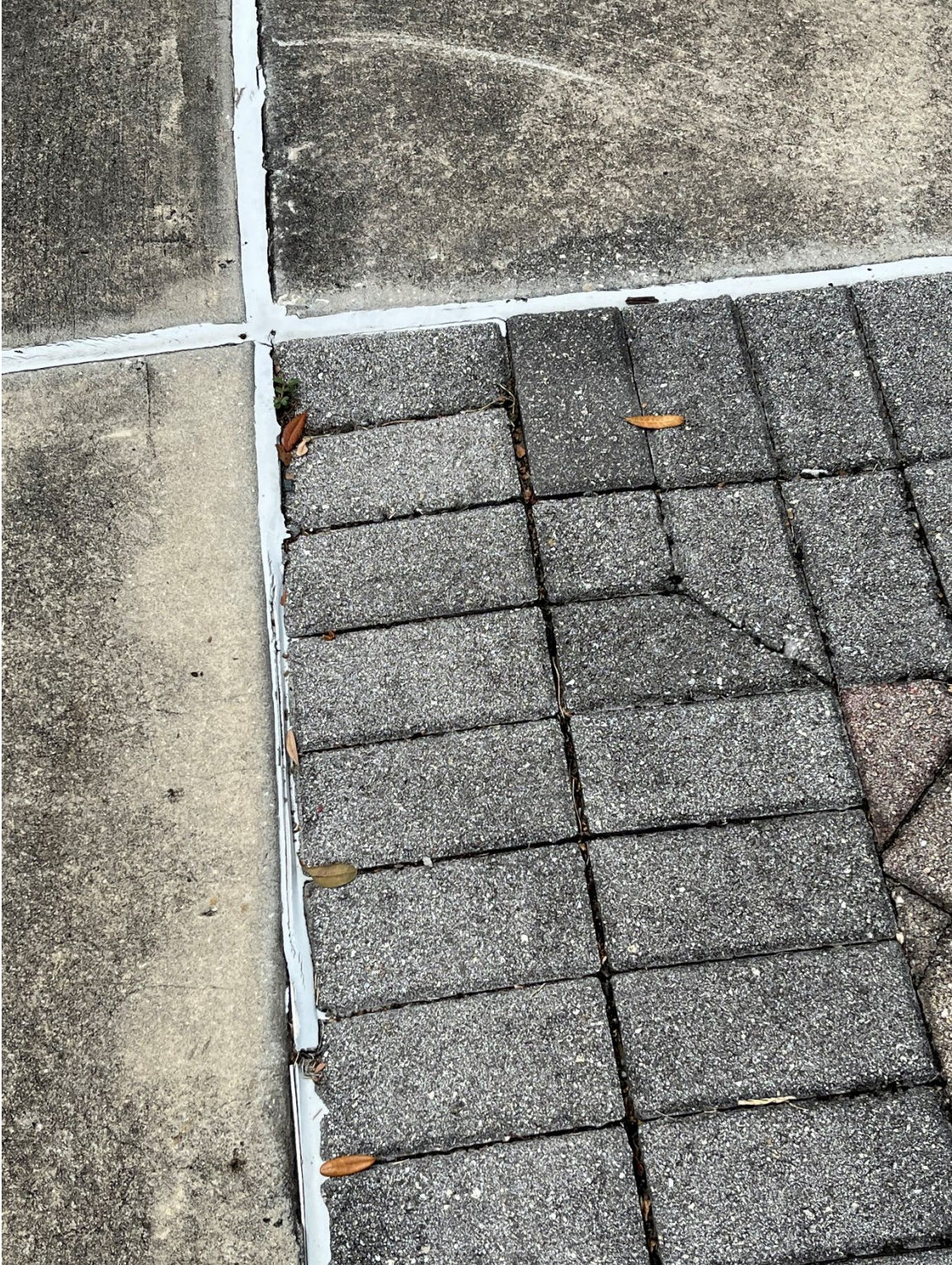
Photo 34 - Paver Base Failure
