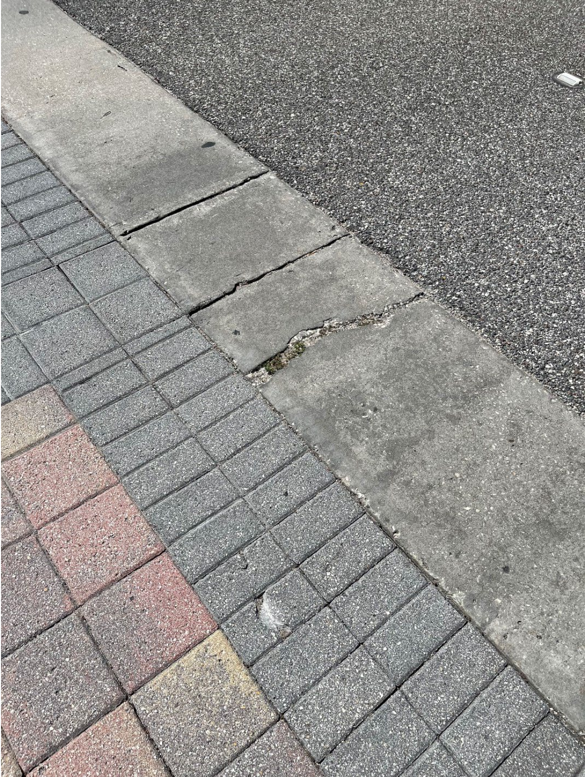
Photo 119 – Construction Entrance – Broken Concrete in Flush Curb
