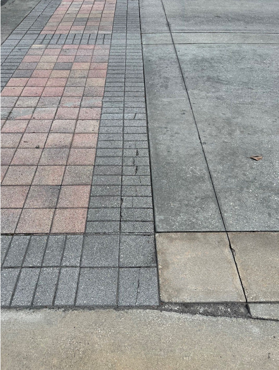
Photo 91 – Cracked Pavers - Minor Settling
