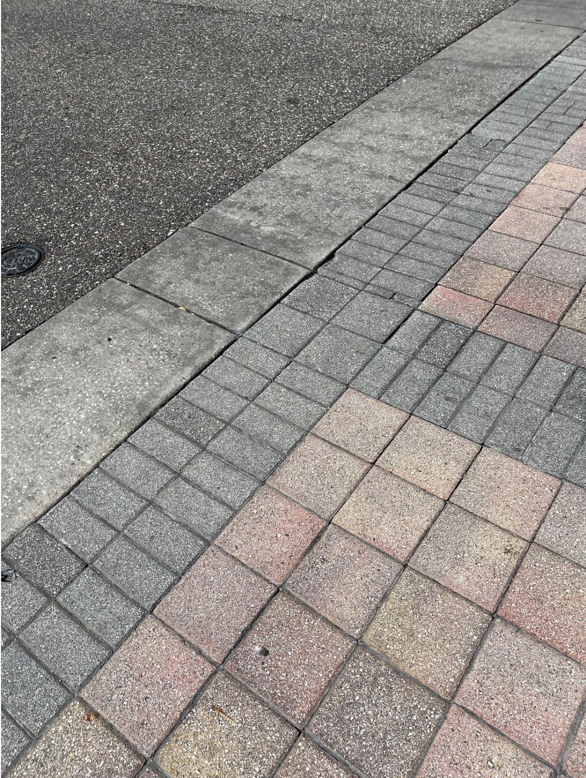
Photo 106 – Cracked Pavers – Settling Pavers
