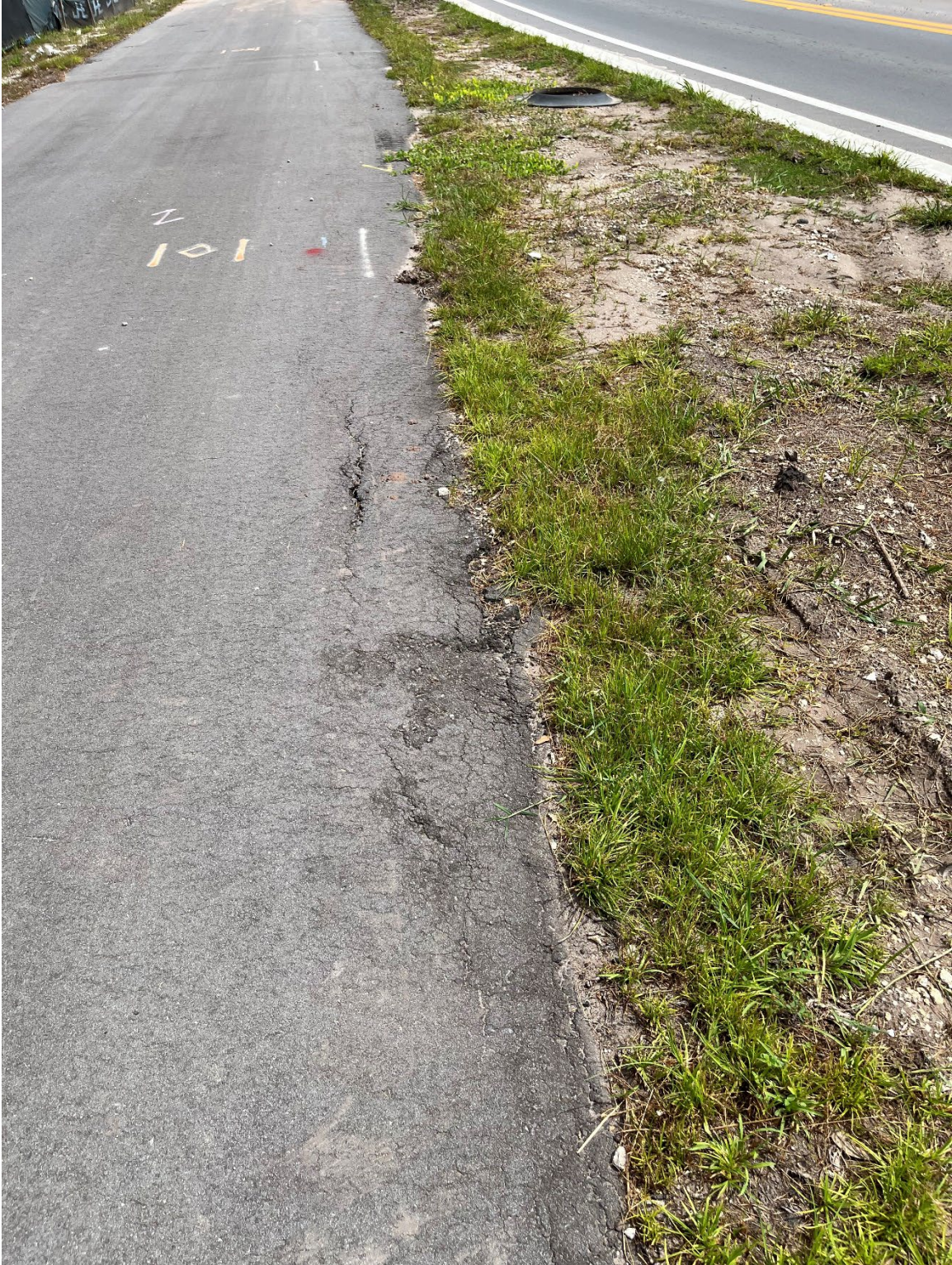
Photo 7 – Raveling Asphalt and Base Failure
