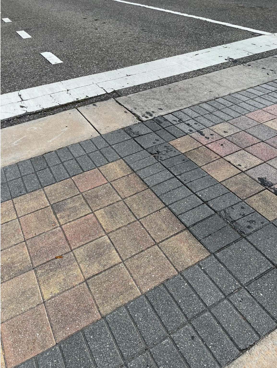
Photo 111 – Broken Concrete Flush Curb
