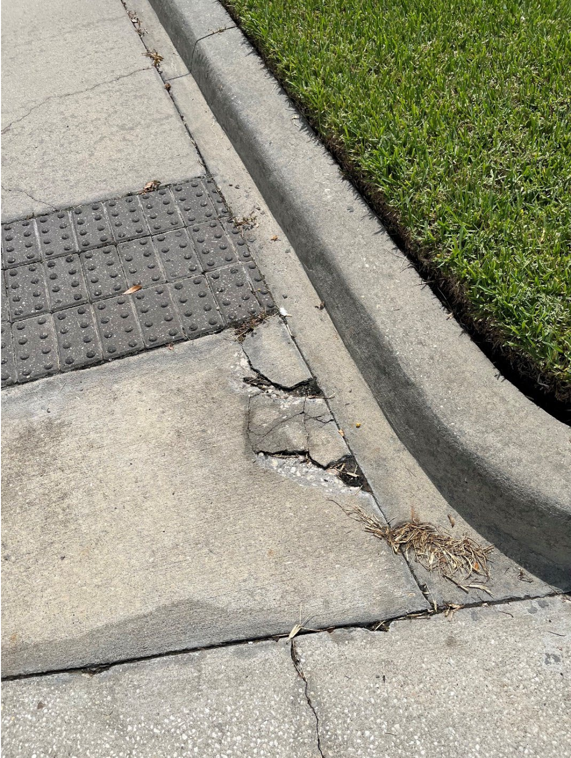
Photo 104 – Cracked Concrete – Some Settling
