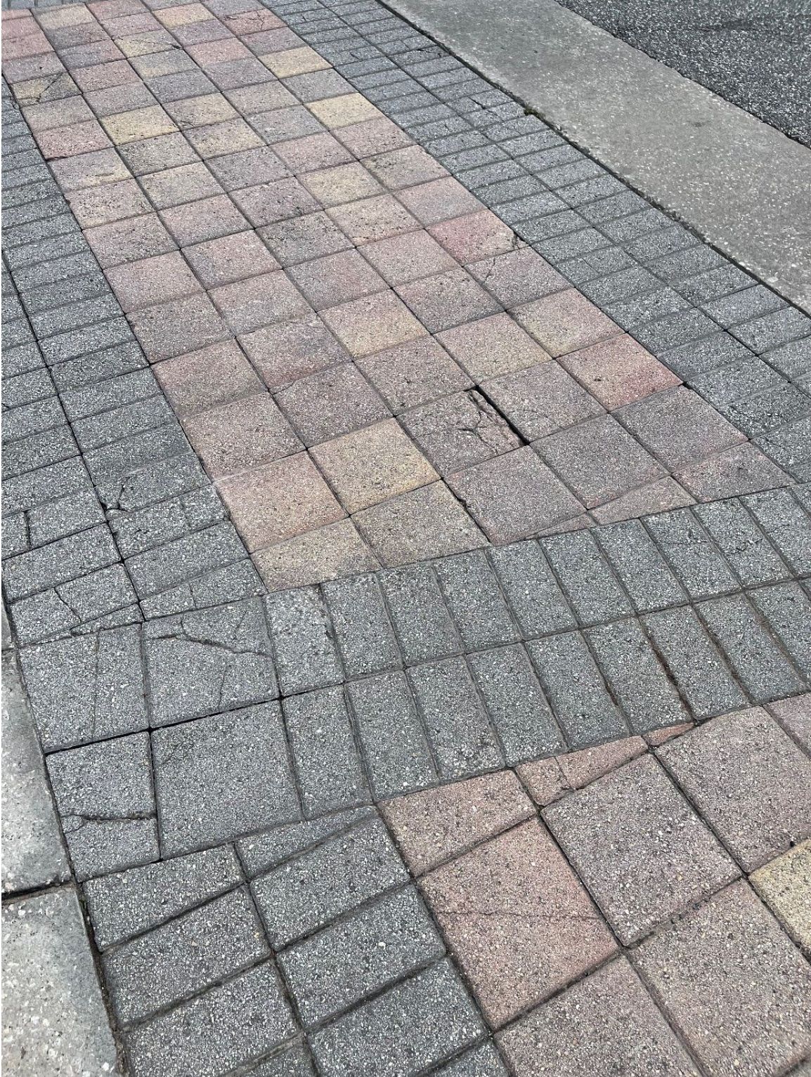
Photo 112 – Cracked Concrete – Pavers Settling
