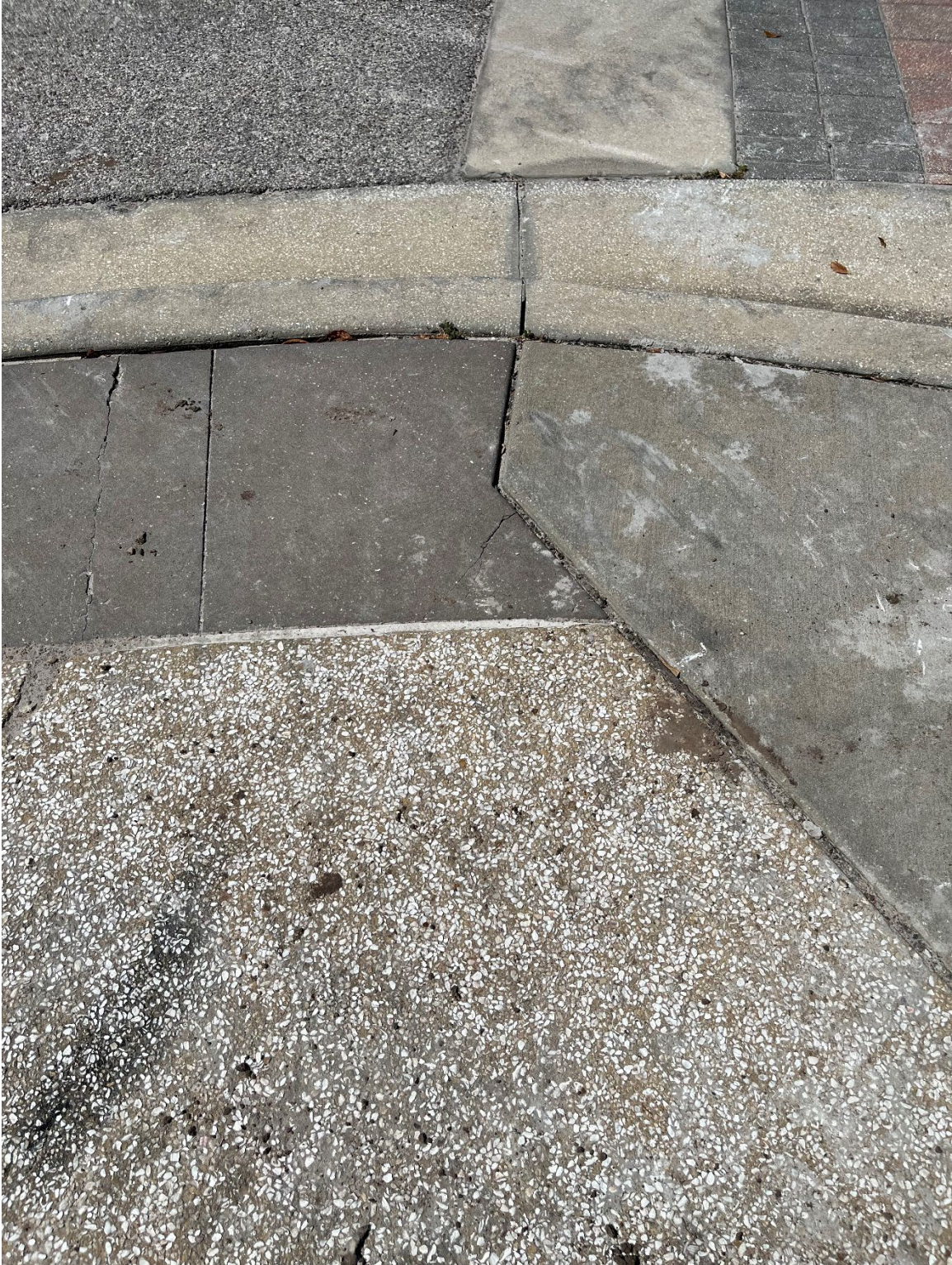
Photo 65 – Concrete Crack in Ribbon Curb (construction ongoing)
