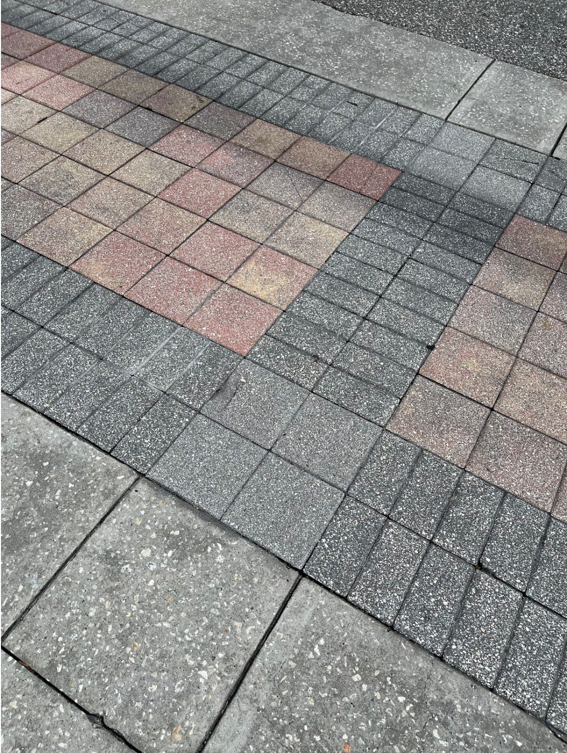
Photo 102– Cracked Pavers – Minor Settling
