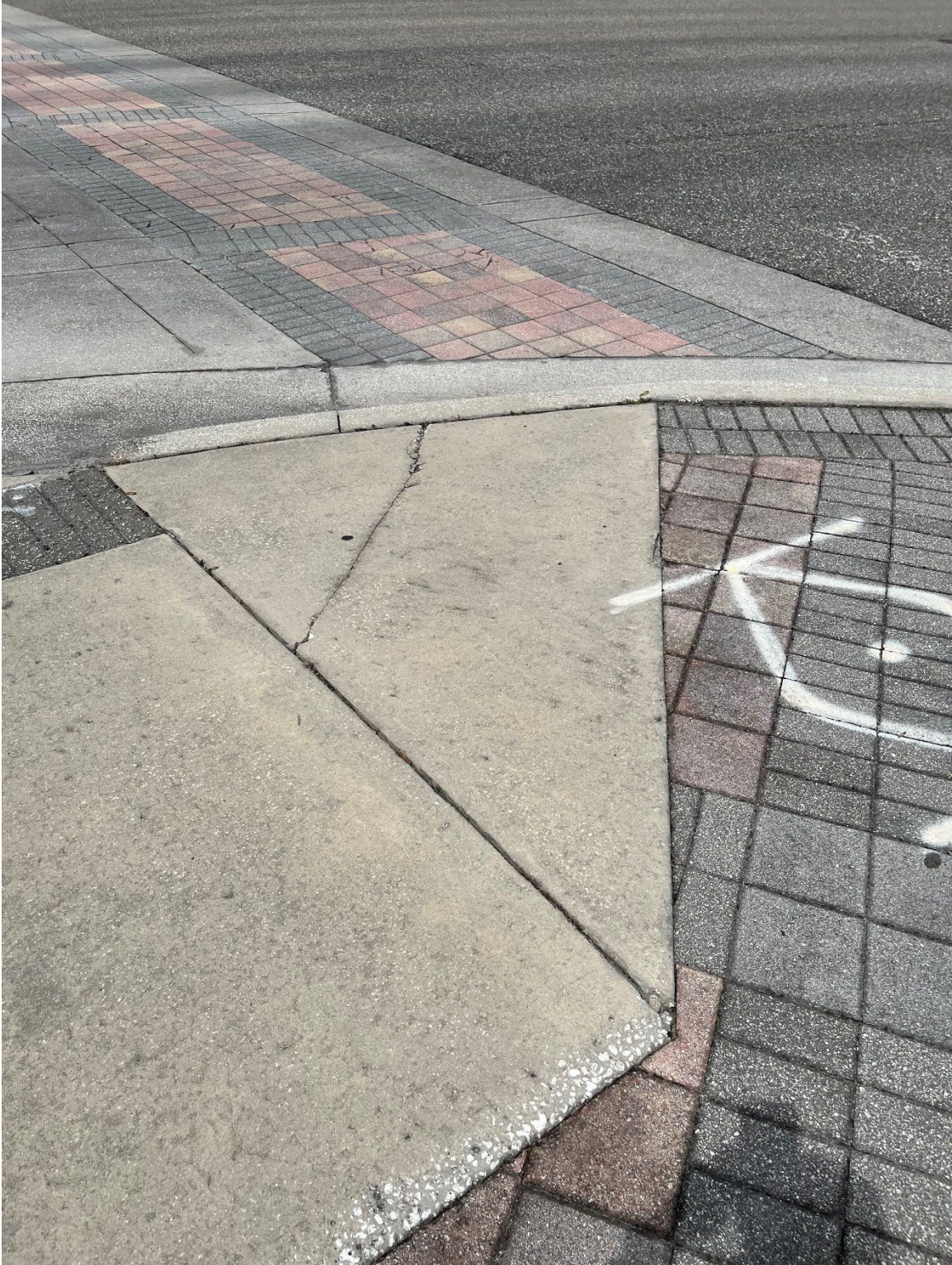
Photo 15 – Surficial Concrete Crack in Handicap Ramp
