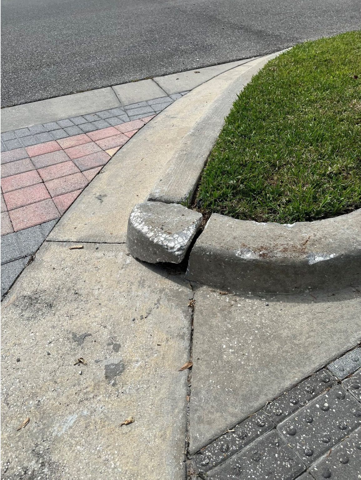
Photo 116 – Broken Concrete Curb
