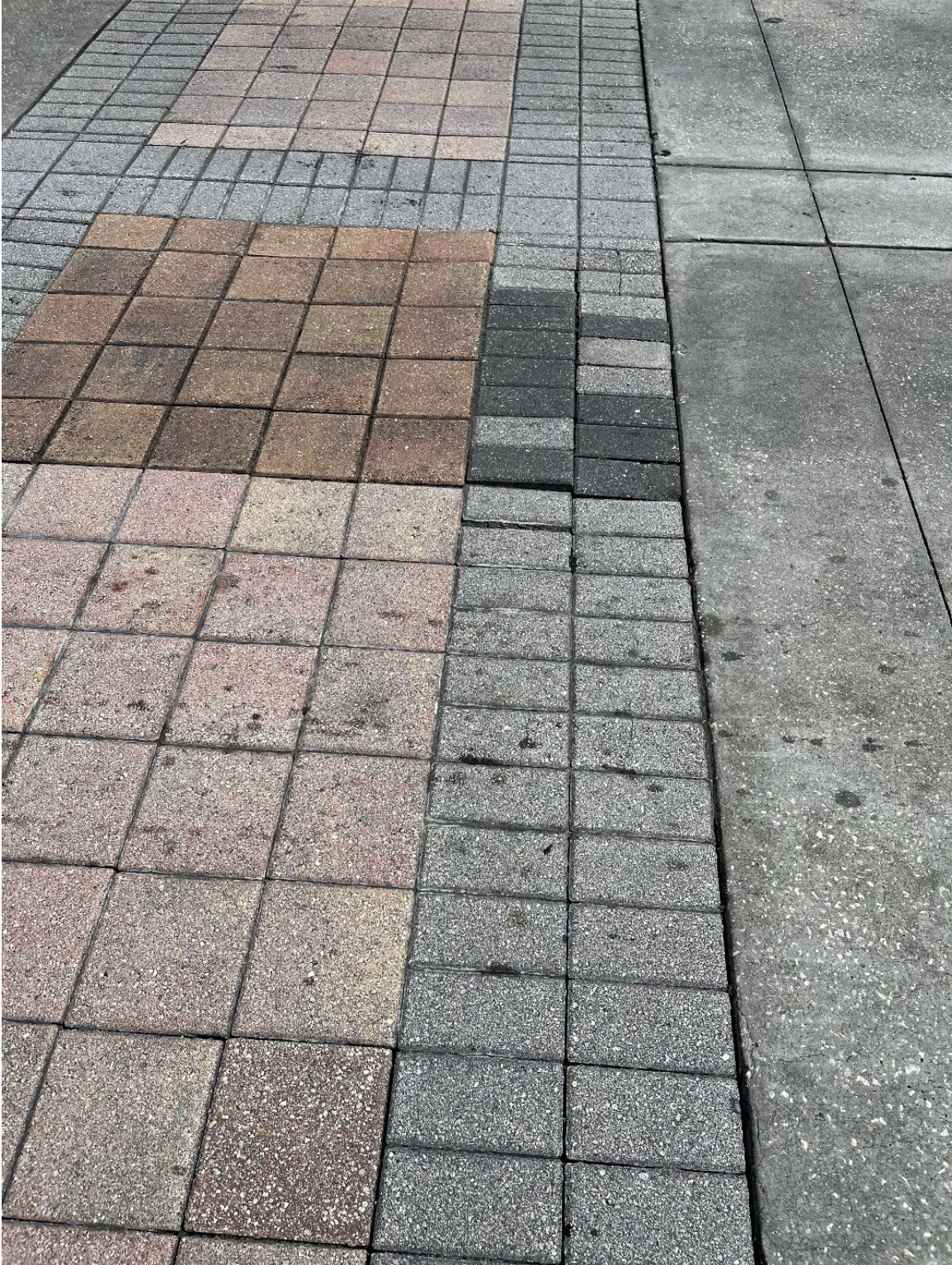
Photo 92 – Surficial Paver Cracks- Minor Settling
