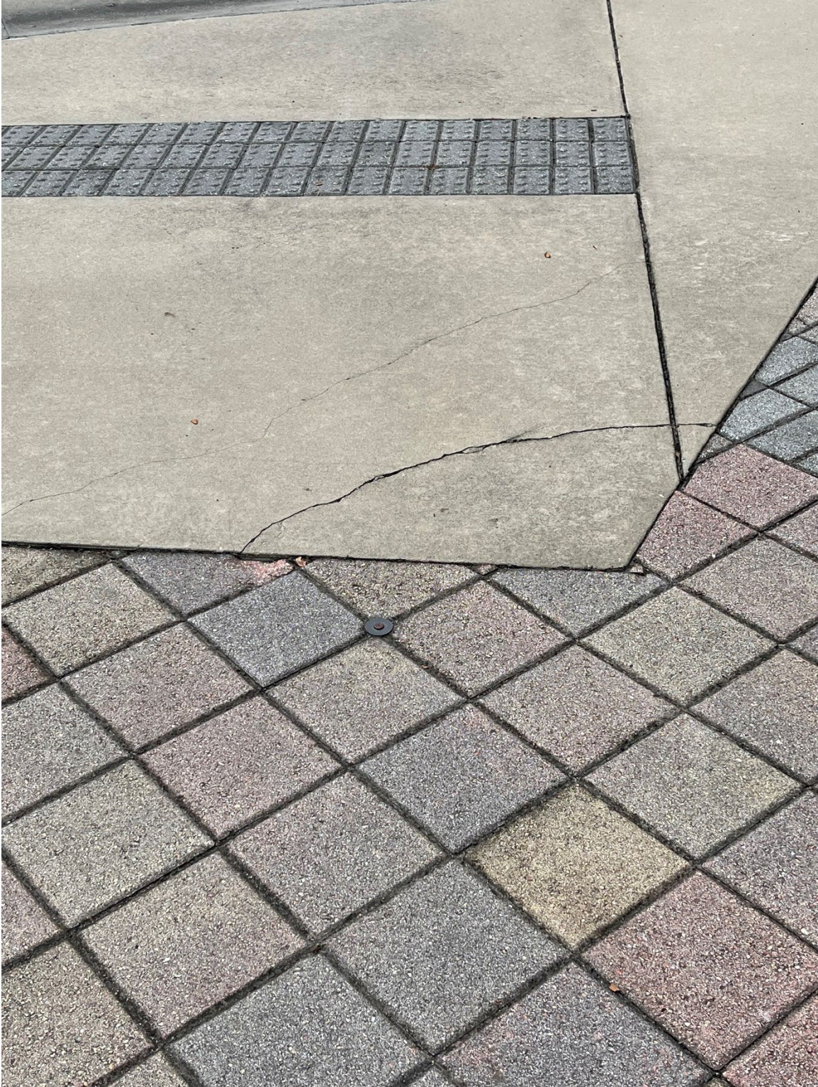
Photo 40 - Surficial Concrete Cracks in Handicap Ramp
