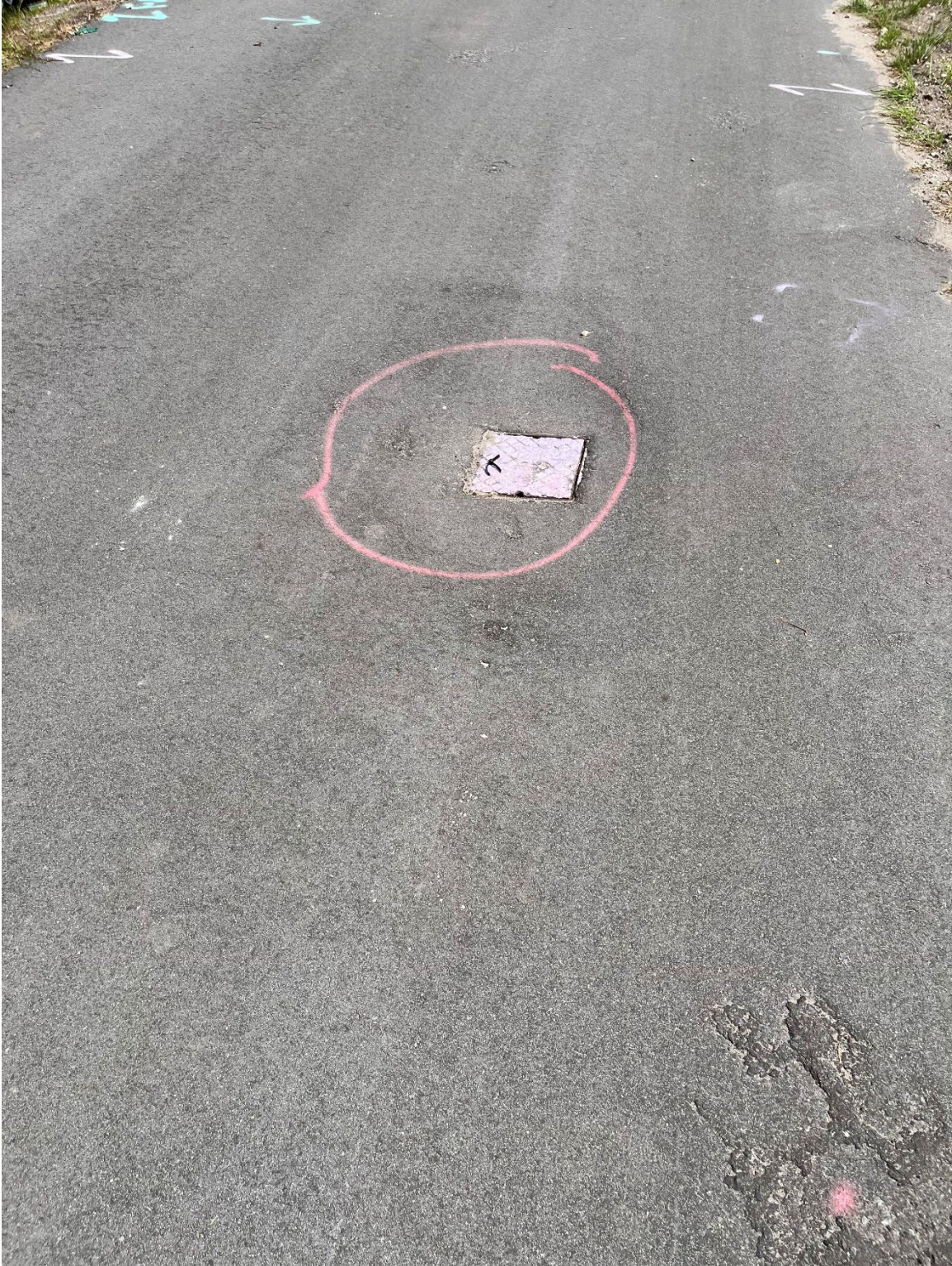
Photo 8 – Sunken Reclaim Water Meter
