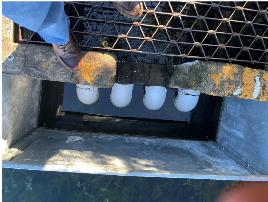
Photo 89 – Drawdown Pipe Inside of Outfall Structure
