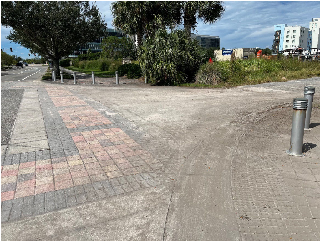
Photo 118 – Construction Entrance – Broken Concrete in Flush Curb
