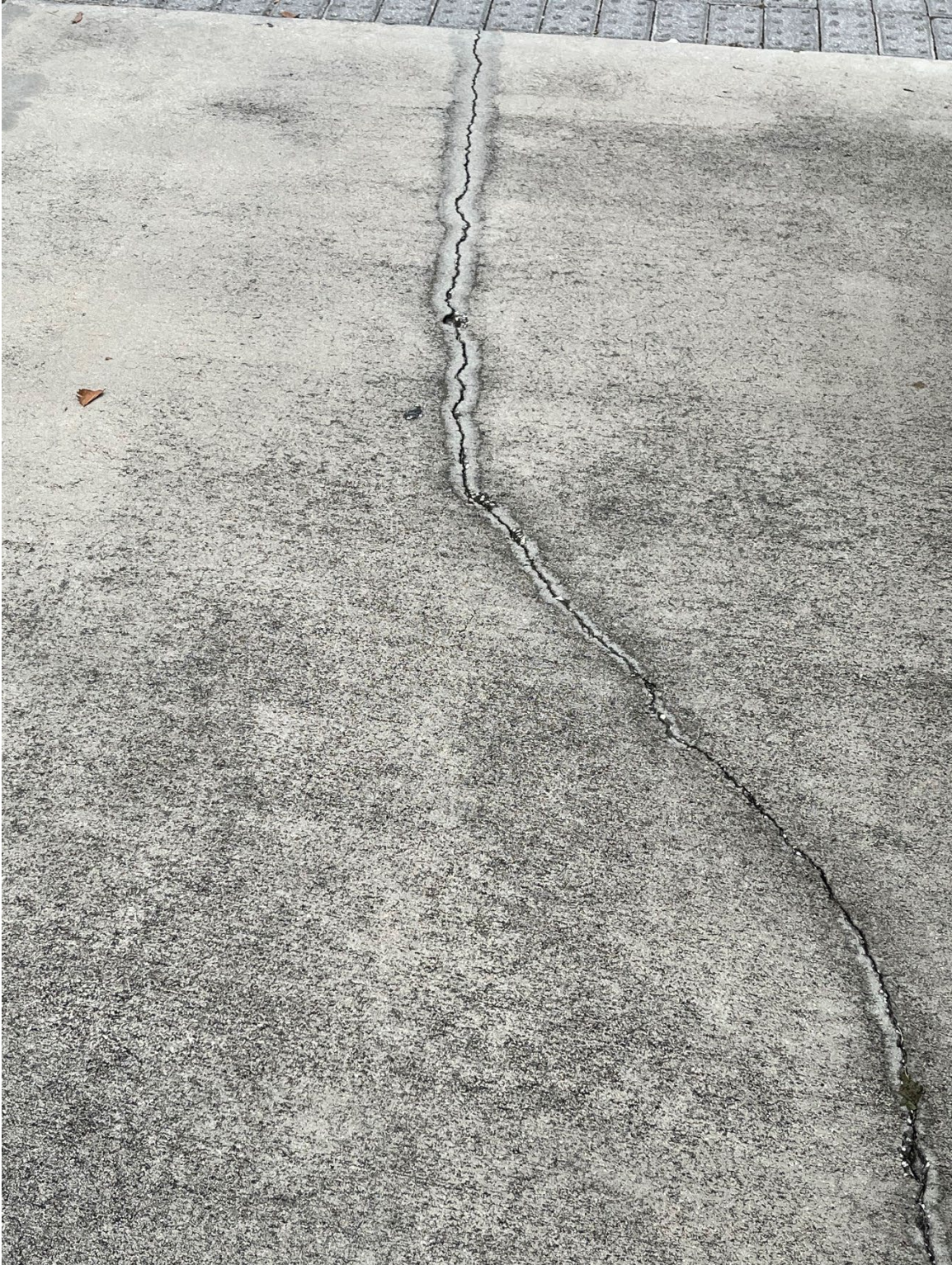
Photo 39 – Surficial Concrete Cracks in Median Strip
