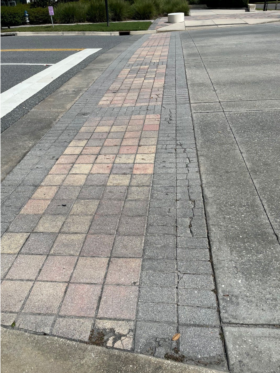
Photo 108 – Cracked and Broken Pavers – Some Settling
