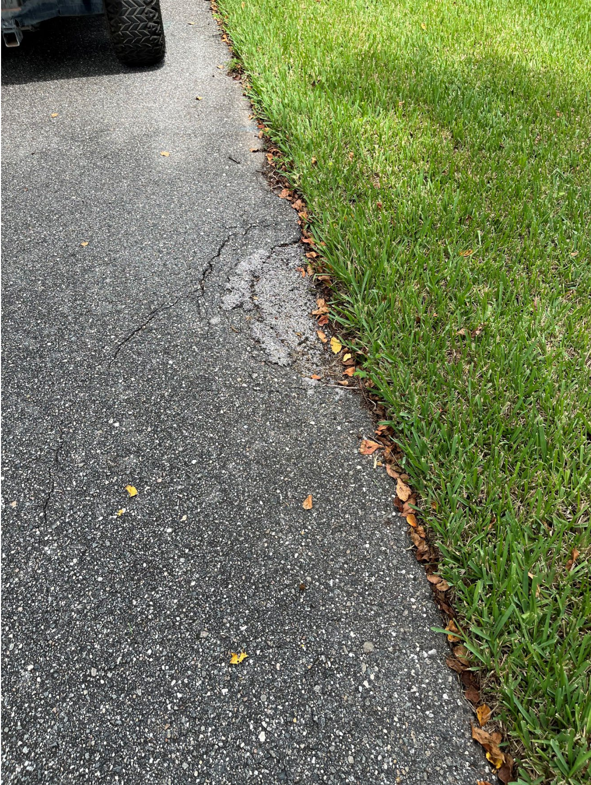
Photo 43 – Raveling Asphalt and Base Failure
