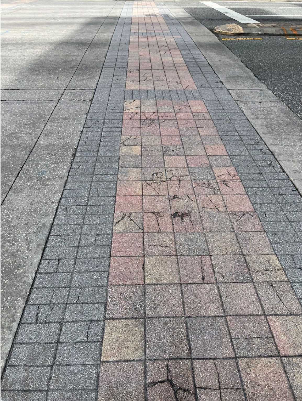
Photo 97 – Cracked Pavers
