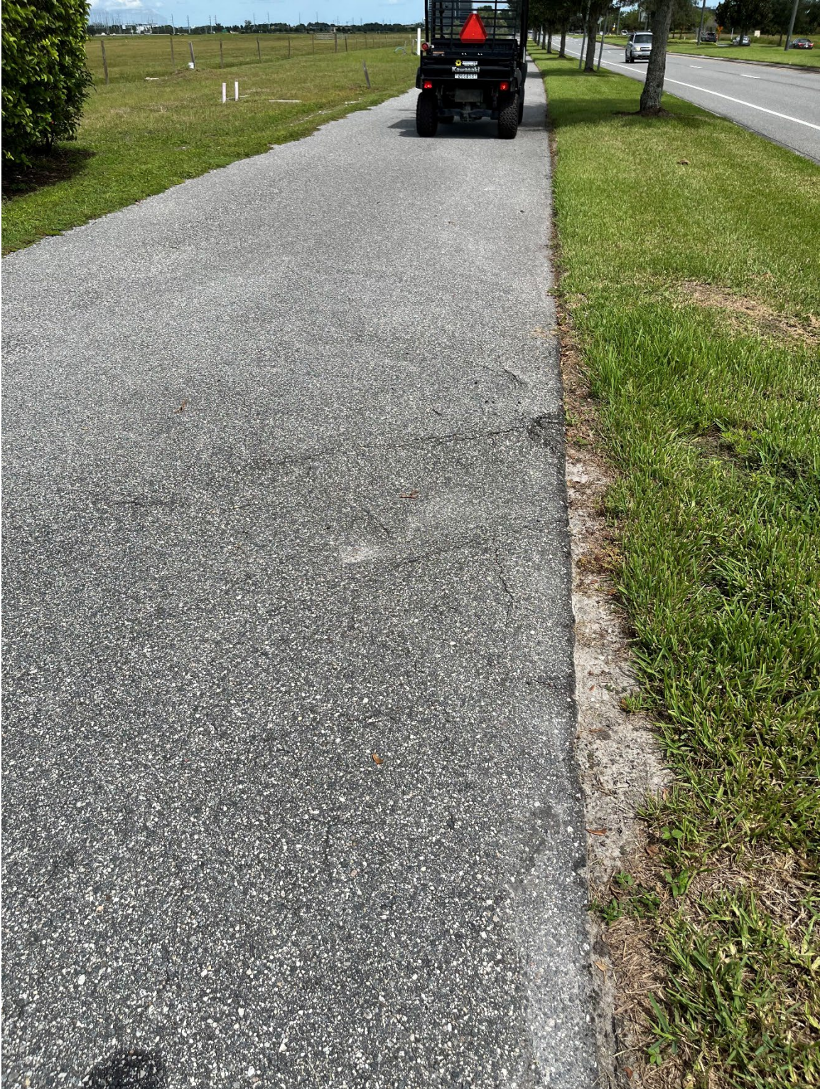
Photo 11 – Raveling Asphalt with Depression and Base Failure
