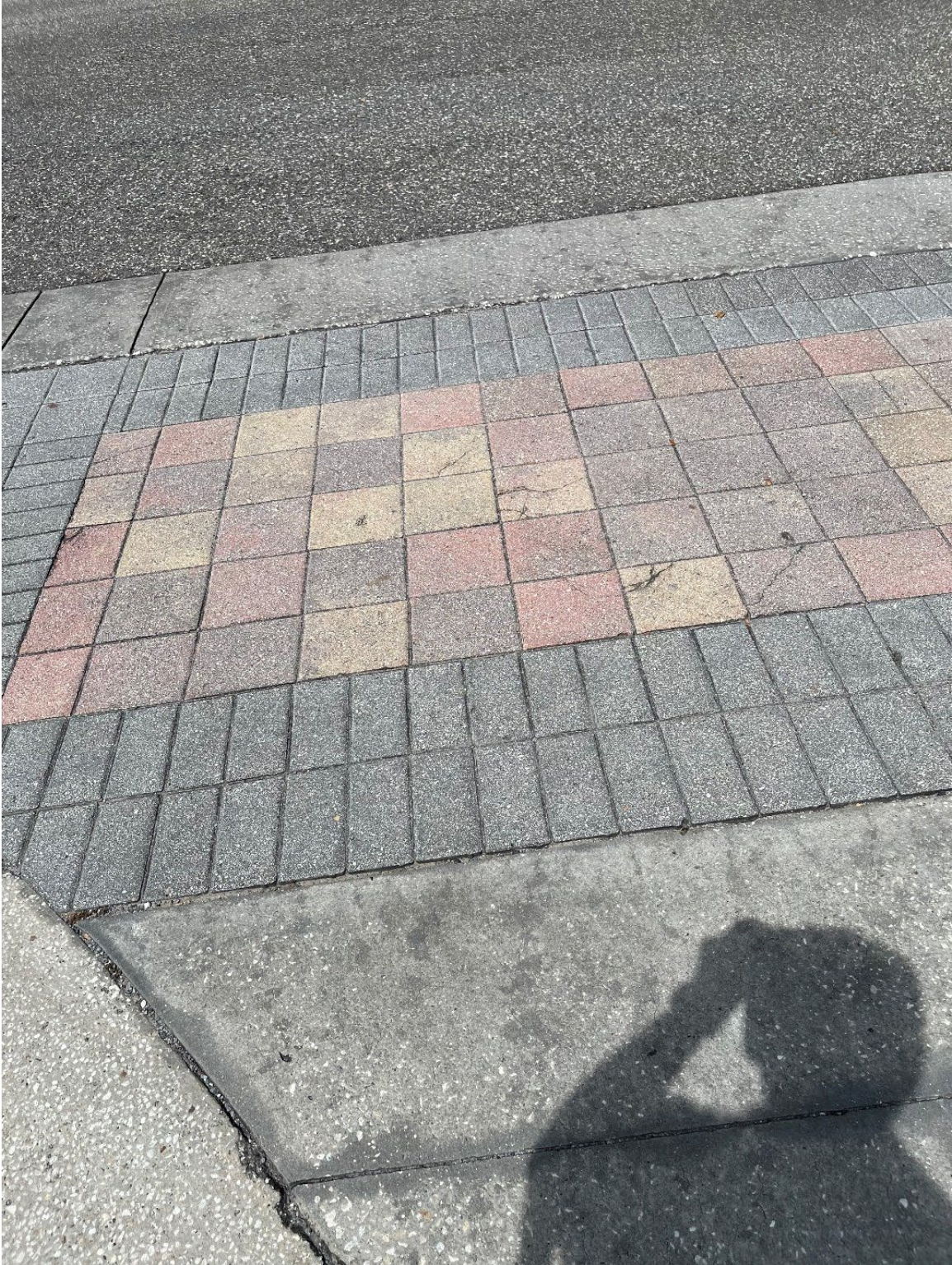
Photo 105 – Cracked Pavers – Some Settling
