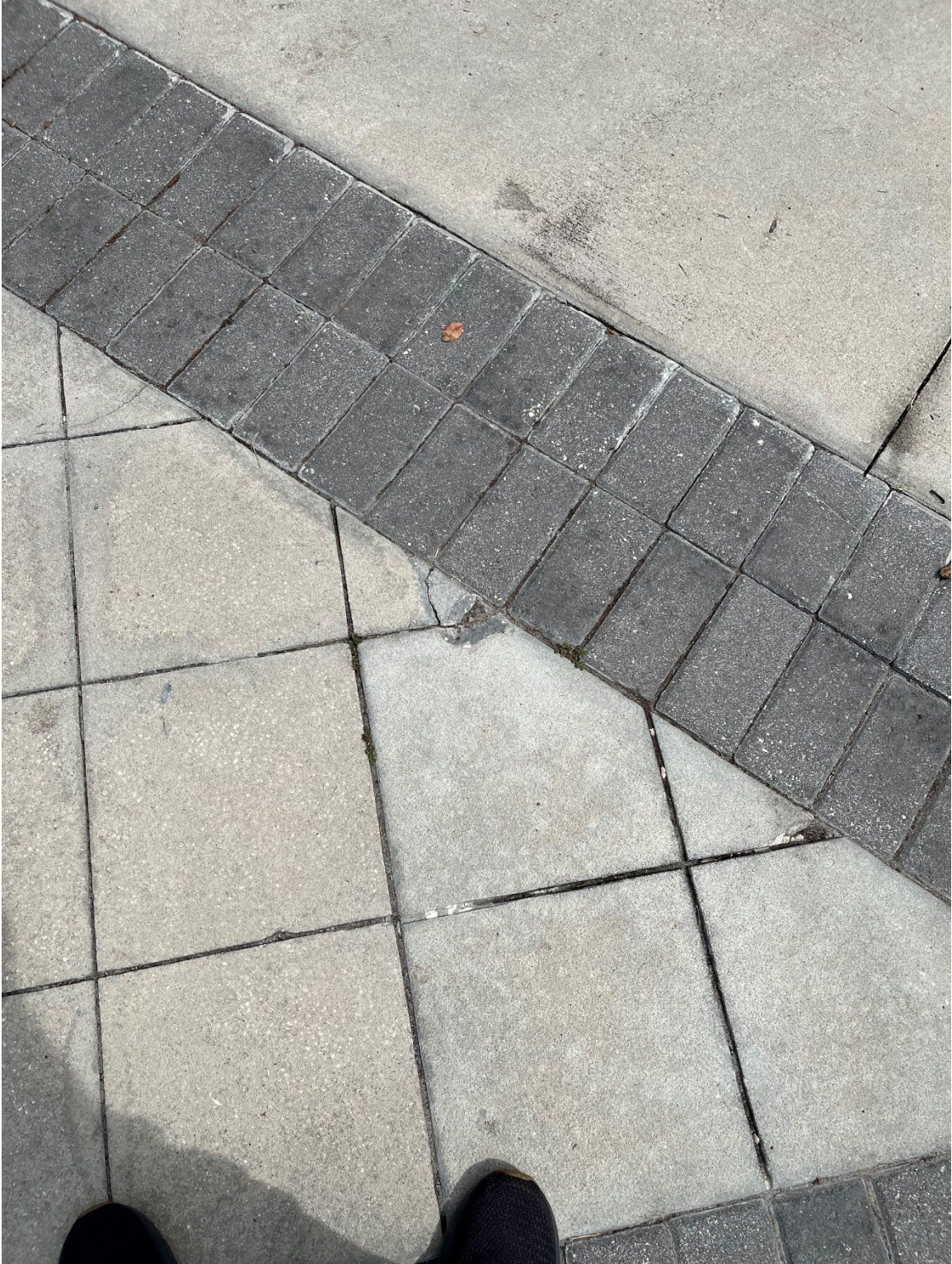
Photo 46 – Multiple Chipped Pavers
