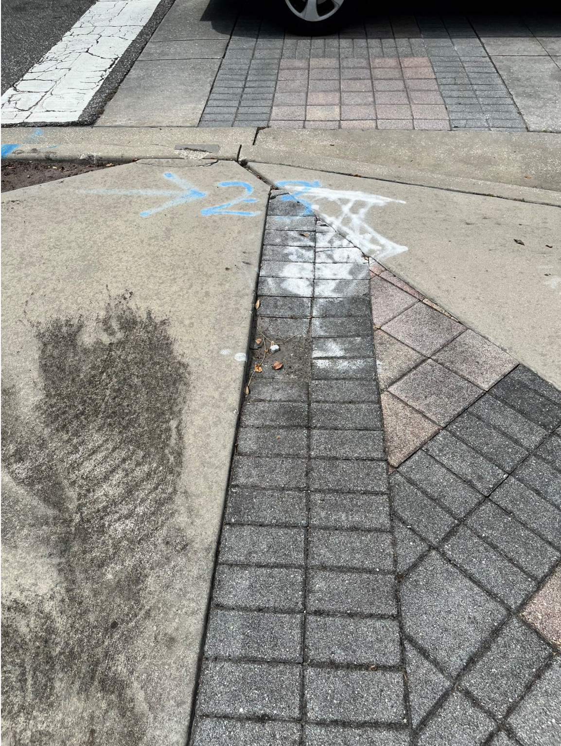
Photo 50 - Cracks in Handicap Ramp, Paver Base Failure
