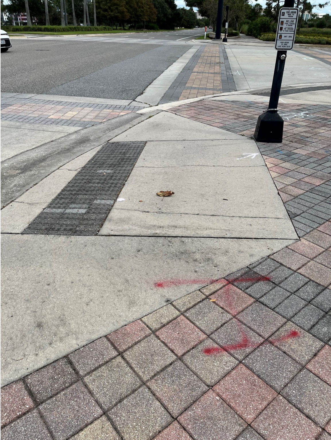
Photo 18 – Surficial Concrete Cracks in Handicap Ramp
