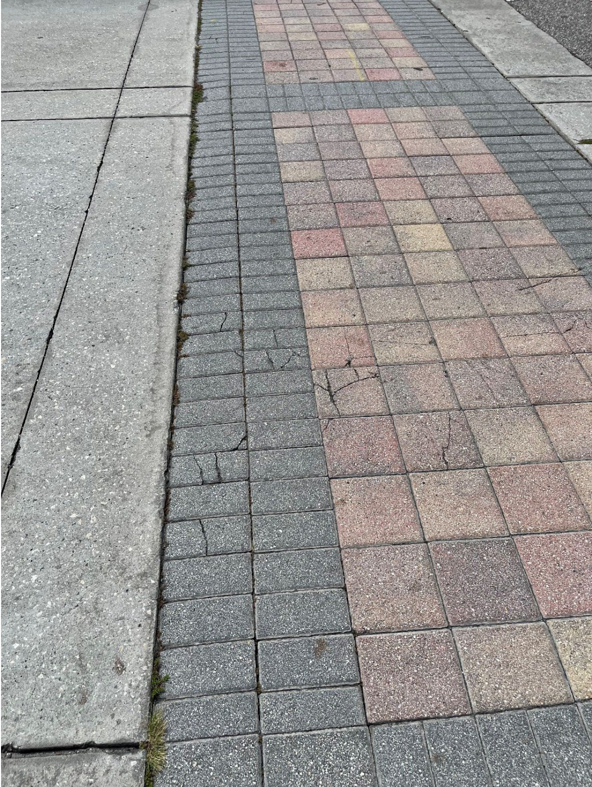
Photo 100 – Cracked Pavers - Sinking Pavers (Approximately ½")
