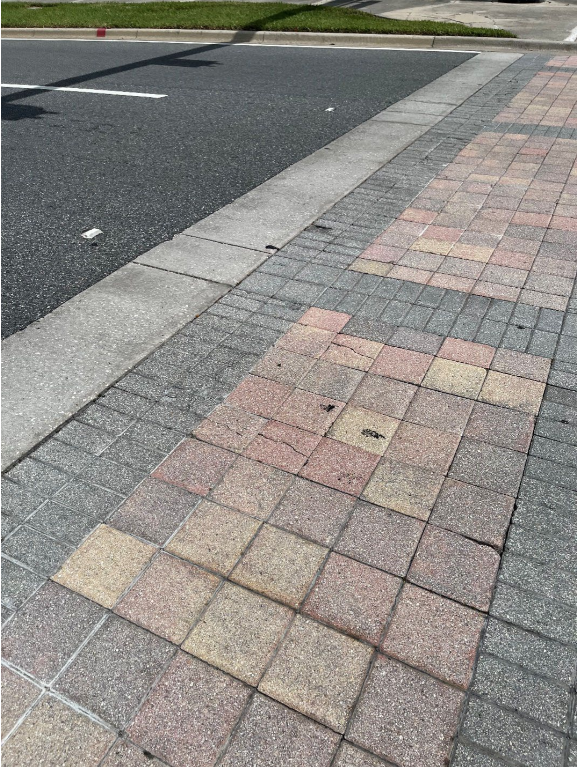
Photo 93 – Surficial Paver Cracks - Minor Settling
