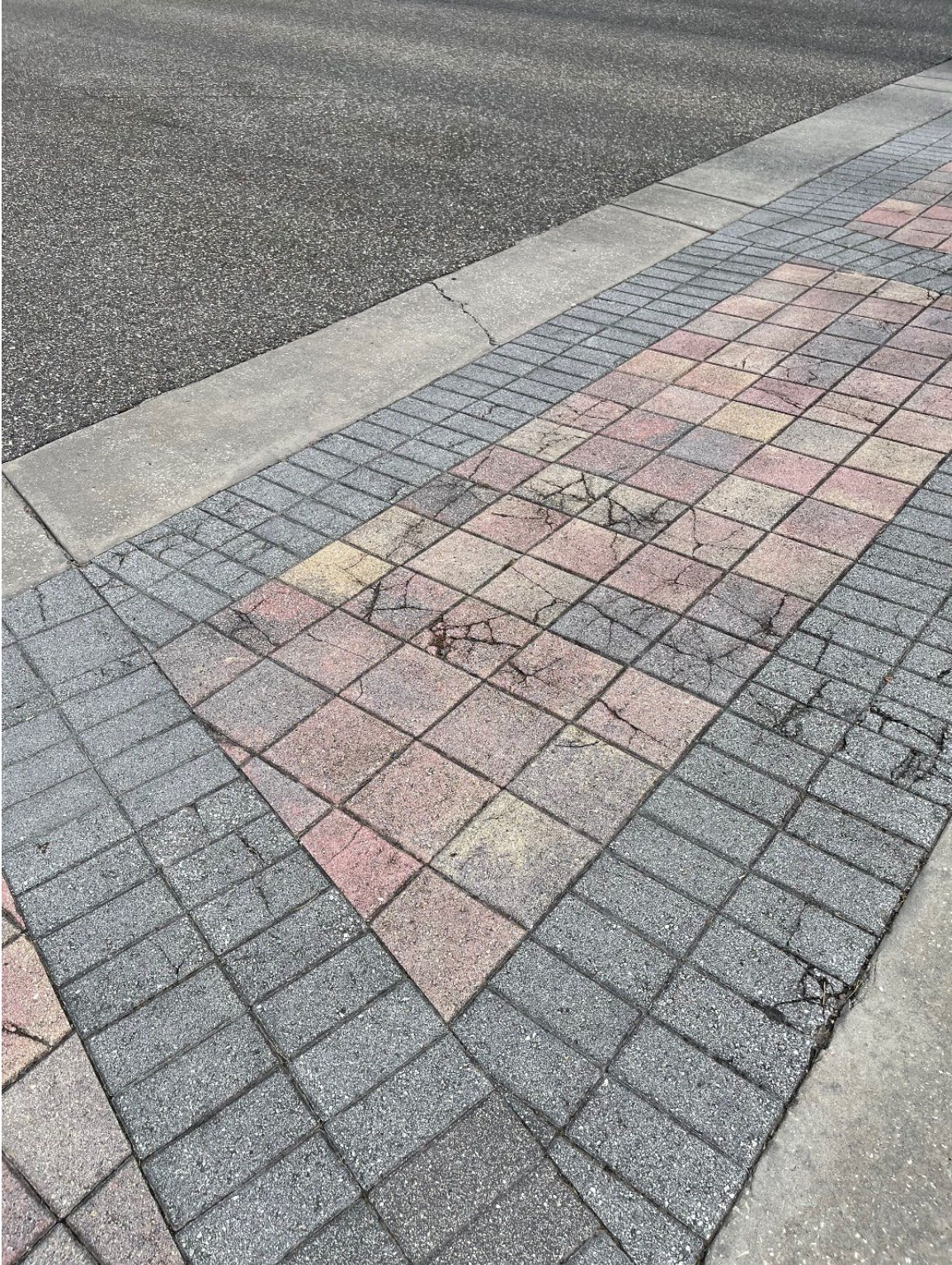
Photo 114 – Multiple Cracked Concrete – Pavers Settling – Broken Curb
