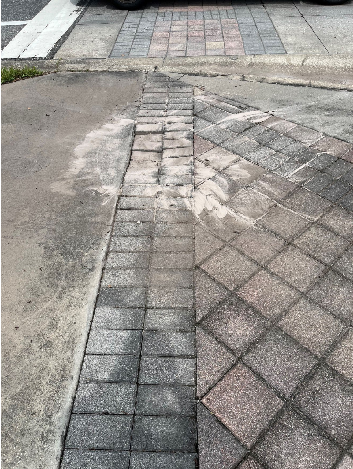
Photo 25 - Paver Base Failure
