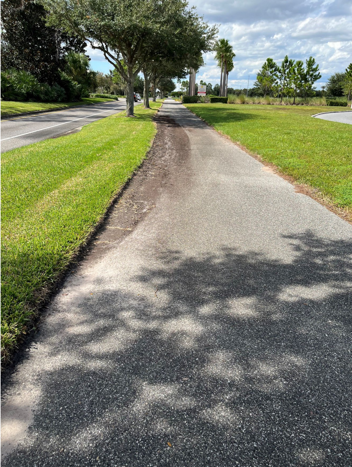
Photo 71 – Poor Drainage
