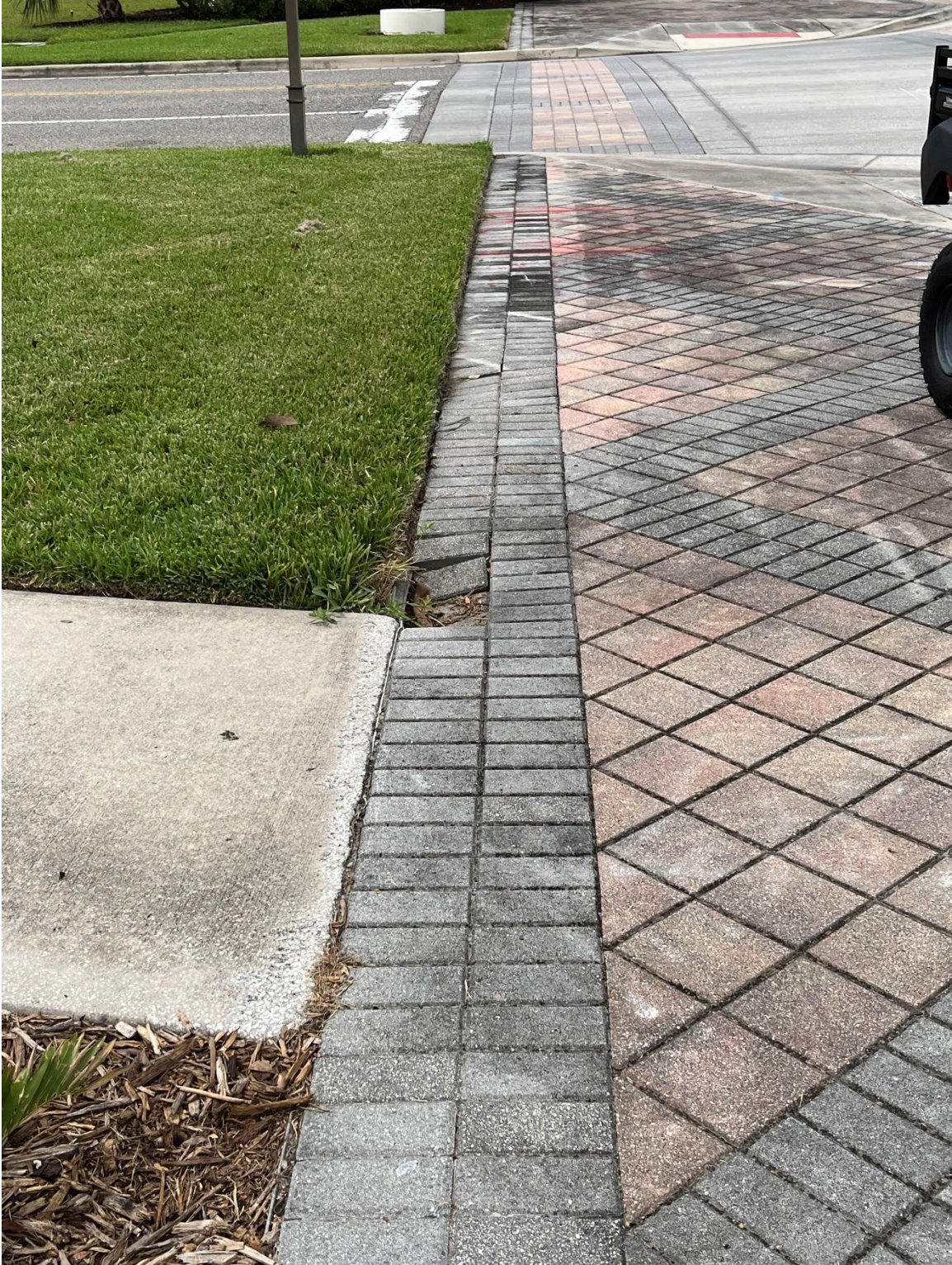
Photo 28 - Paver Base Failure
