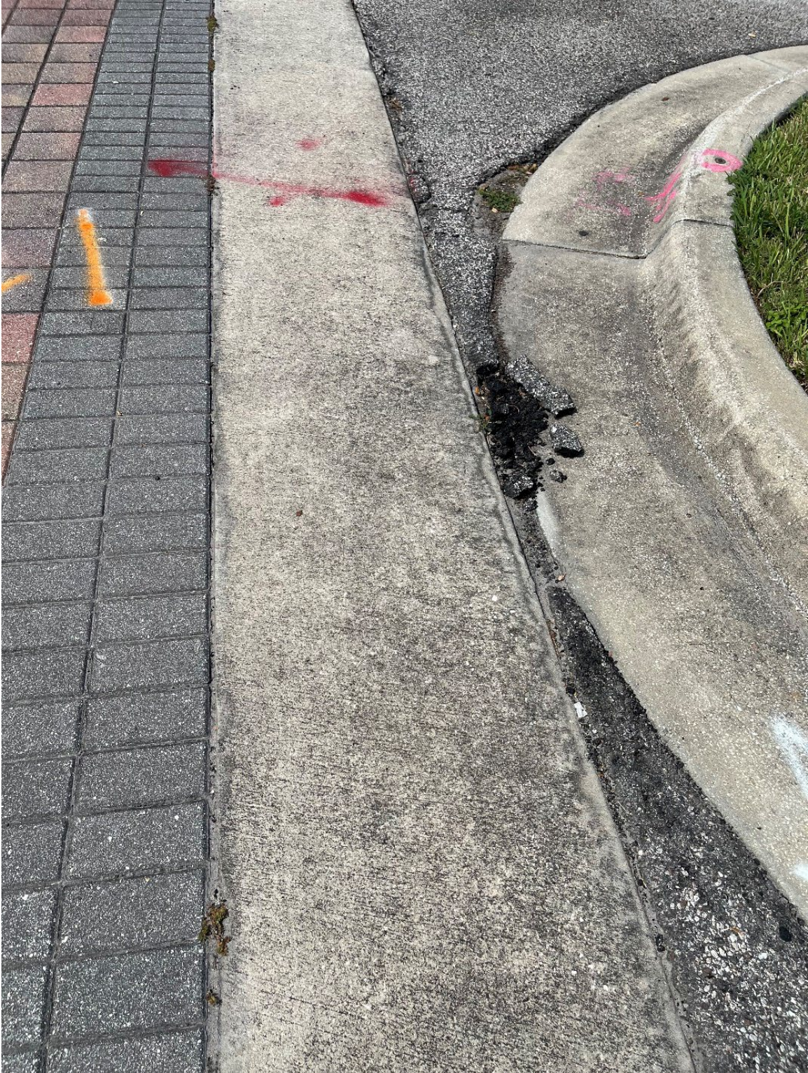
Photo 121 – Broken Concrete
