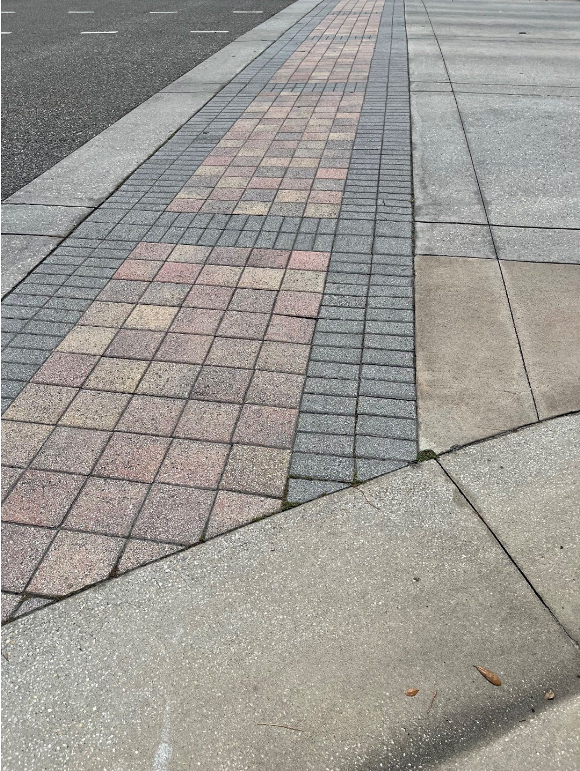
Photo 99 – Cracked Pavers – Paver Settling
