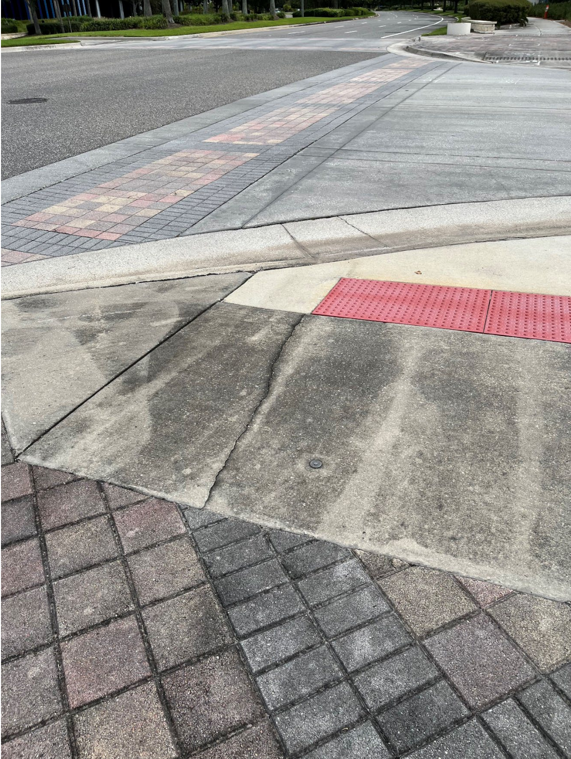
Photo 26 – Surficial Concrete Cracks in Handicap Ramp
