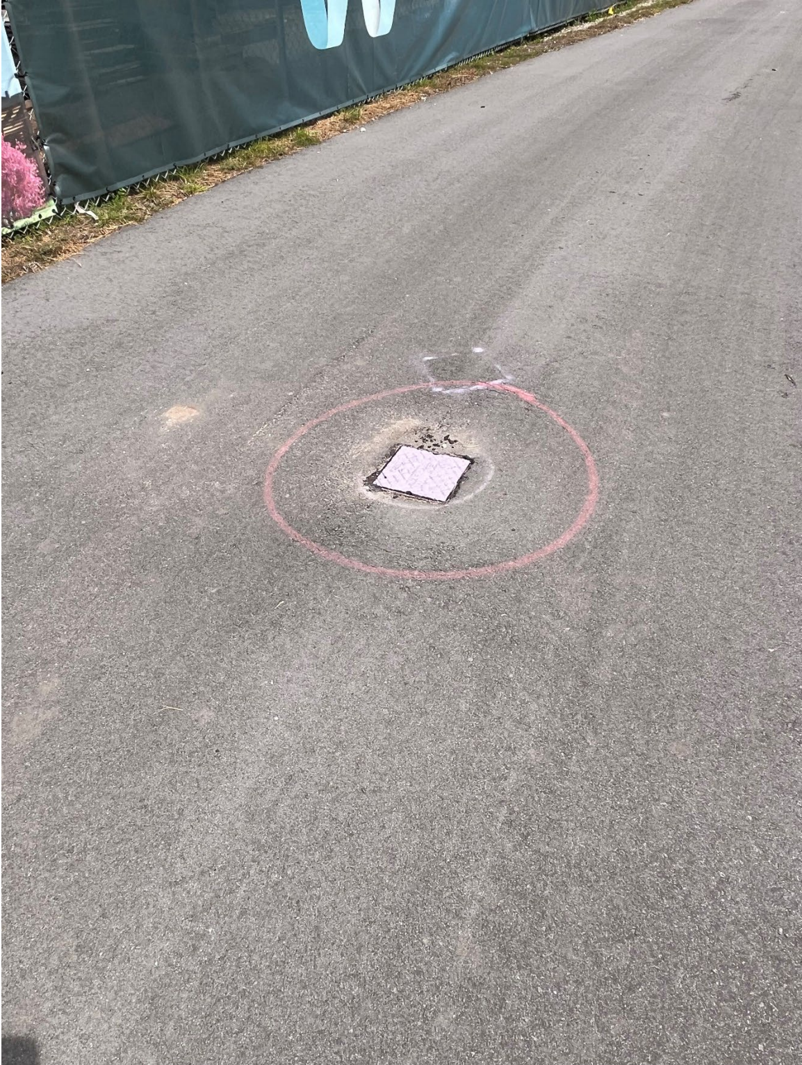
Photo 6 – Sunken Reclaim Water Meter
