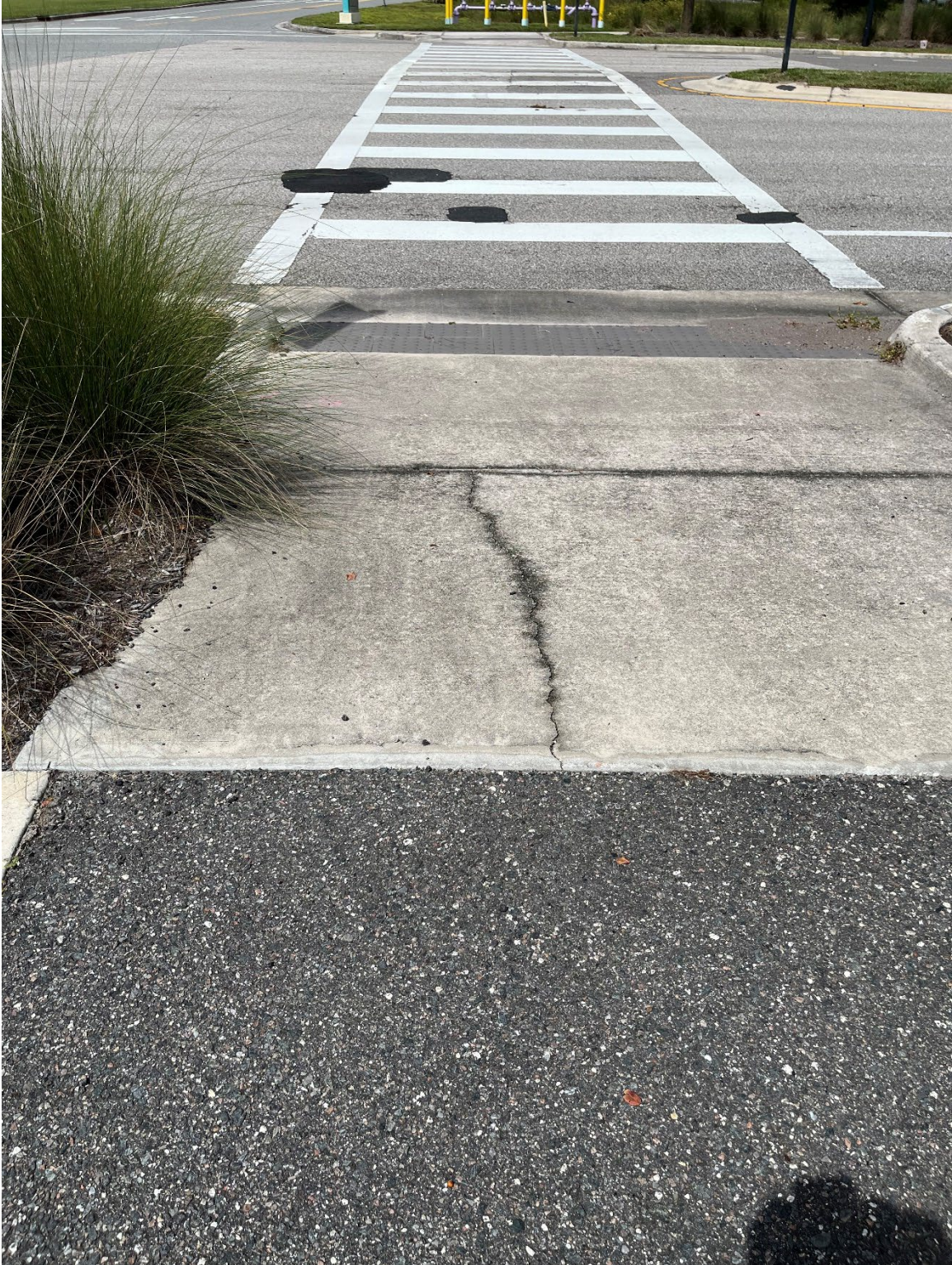
Photo 63 – Surficial Concrete Crack in Handicap Ramp
