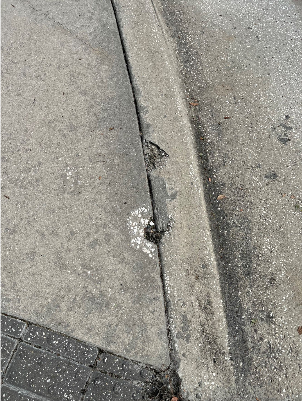
Photo 24 - Cracked Concrete in Handicap Ramp
