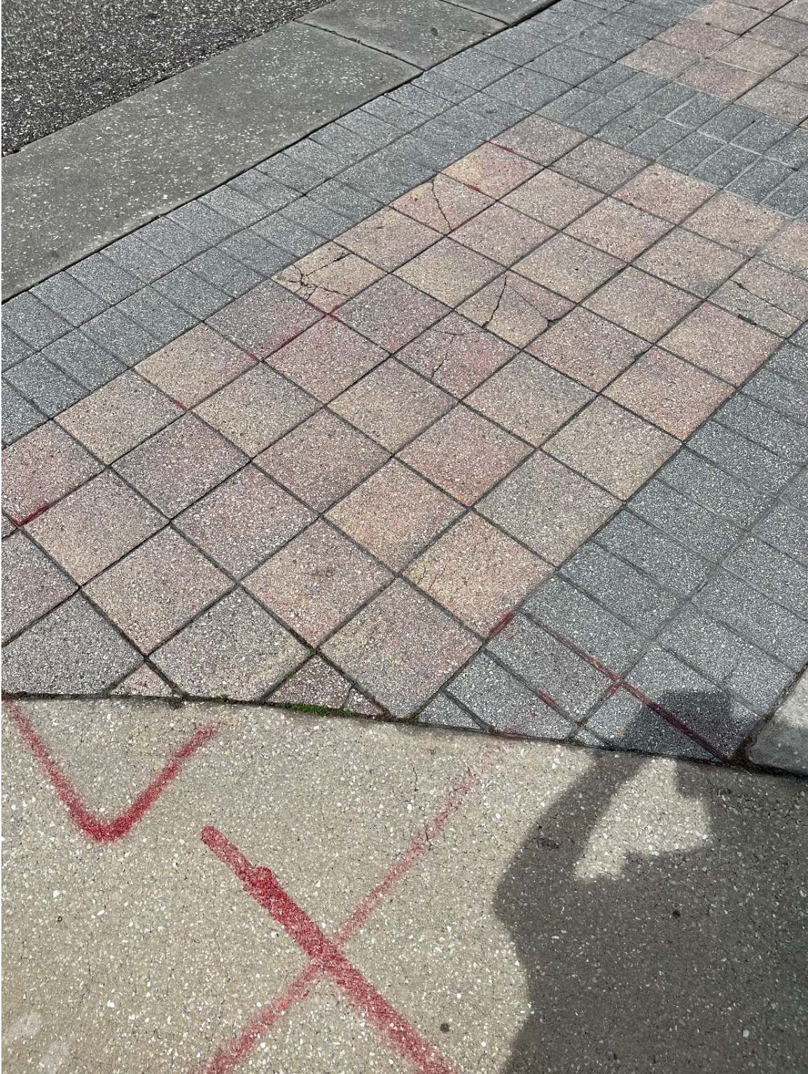
Photo 96 – Cracked Pavers
