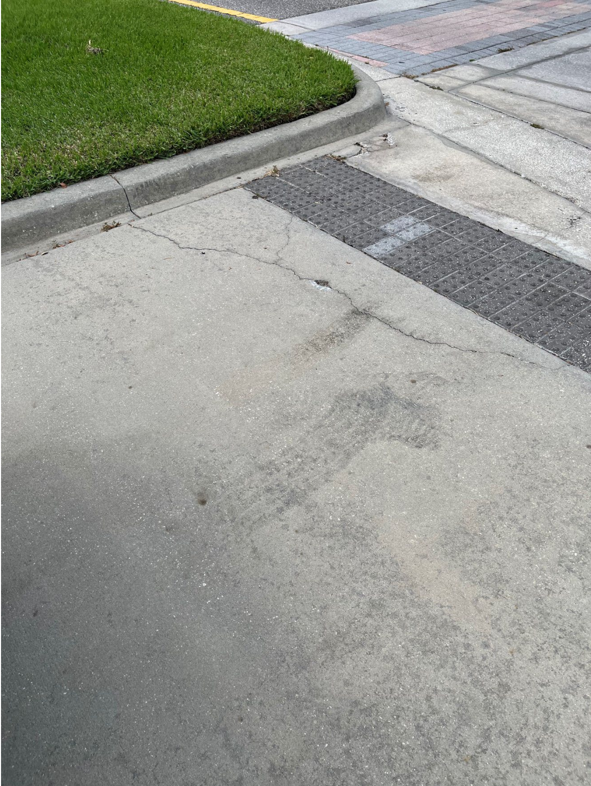
Photo 21 - Surficial Concrete Cracks in Handicap Ramp
