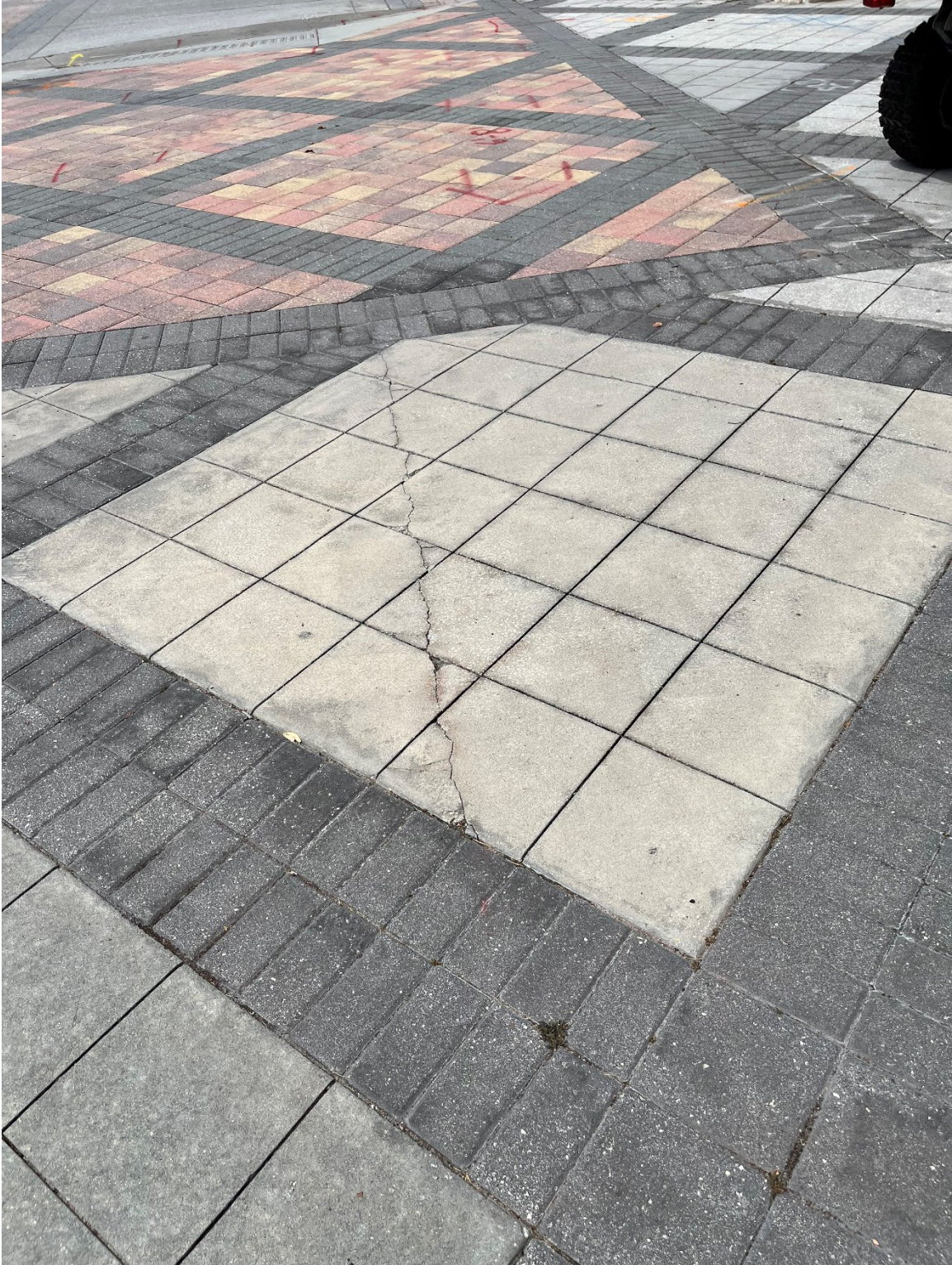
Photo 47 - Broken Pavers
