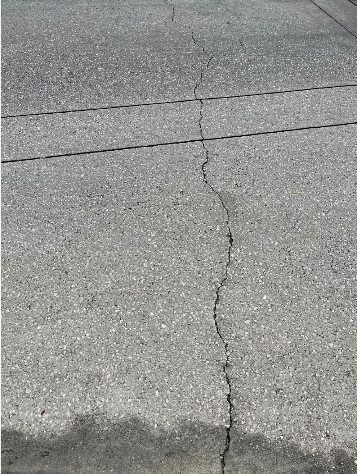
Photo 125 – Surficial Concrete Cracks
