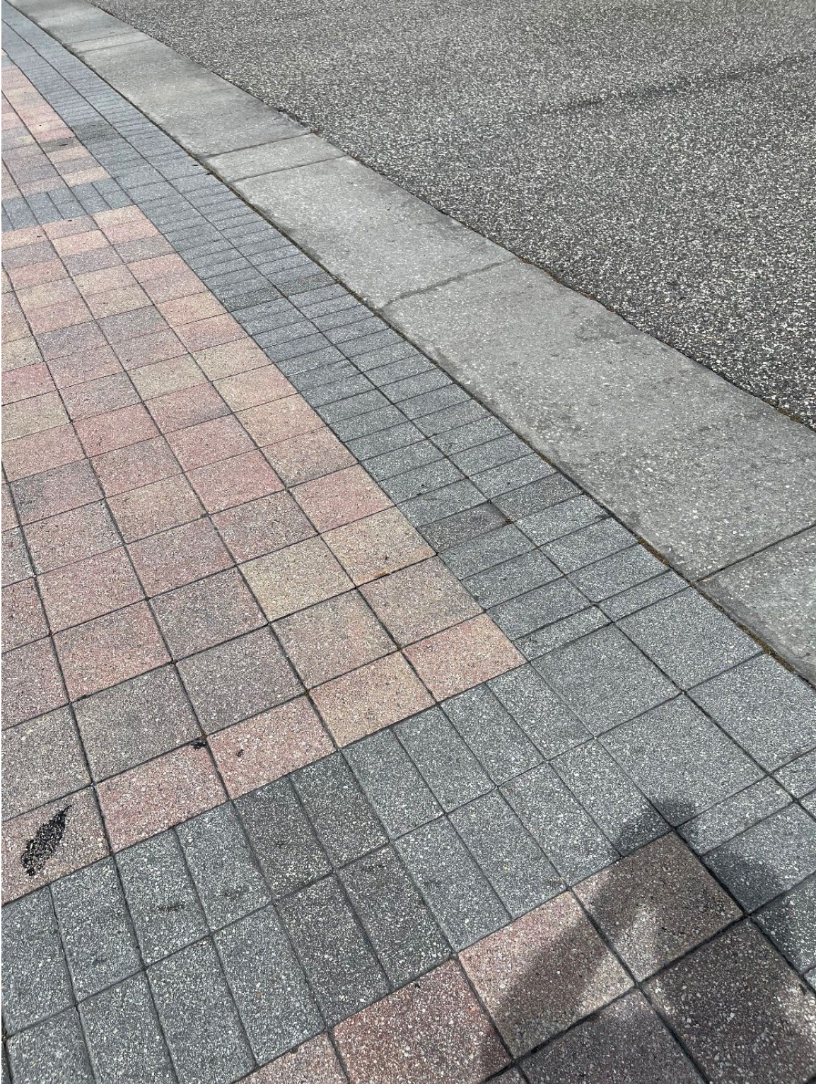
Photo 101 – Cracked Pavers – Minor Settling
