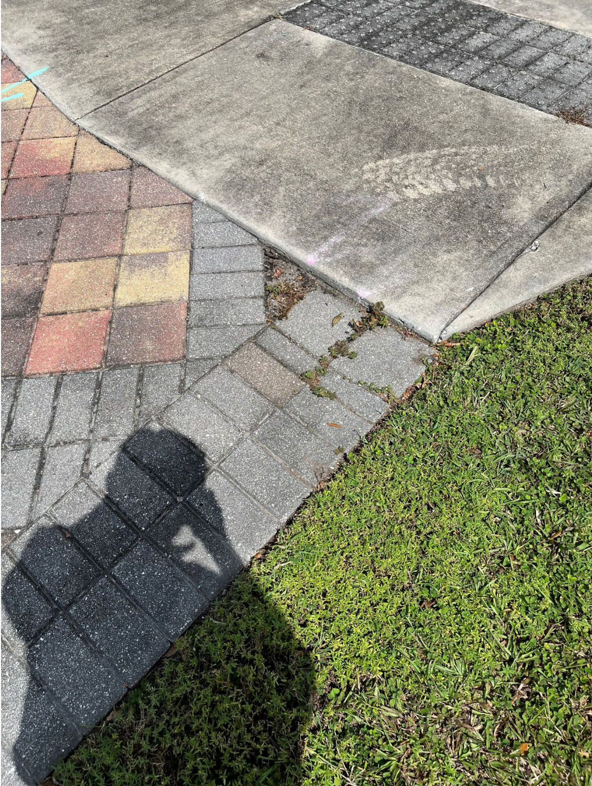
Photo 59 - Paver Base Failure
