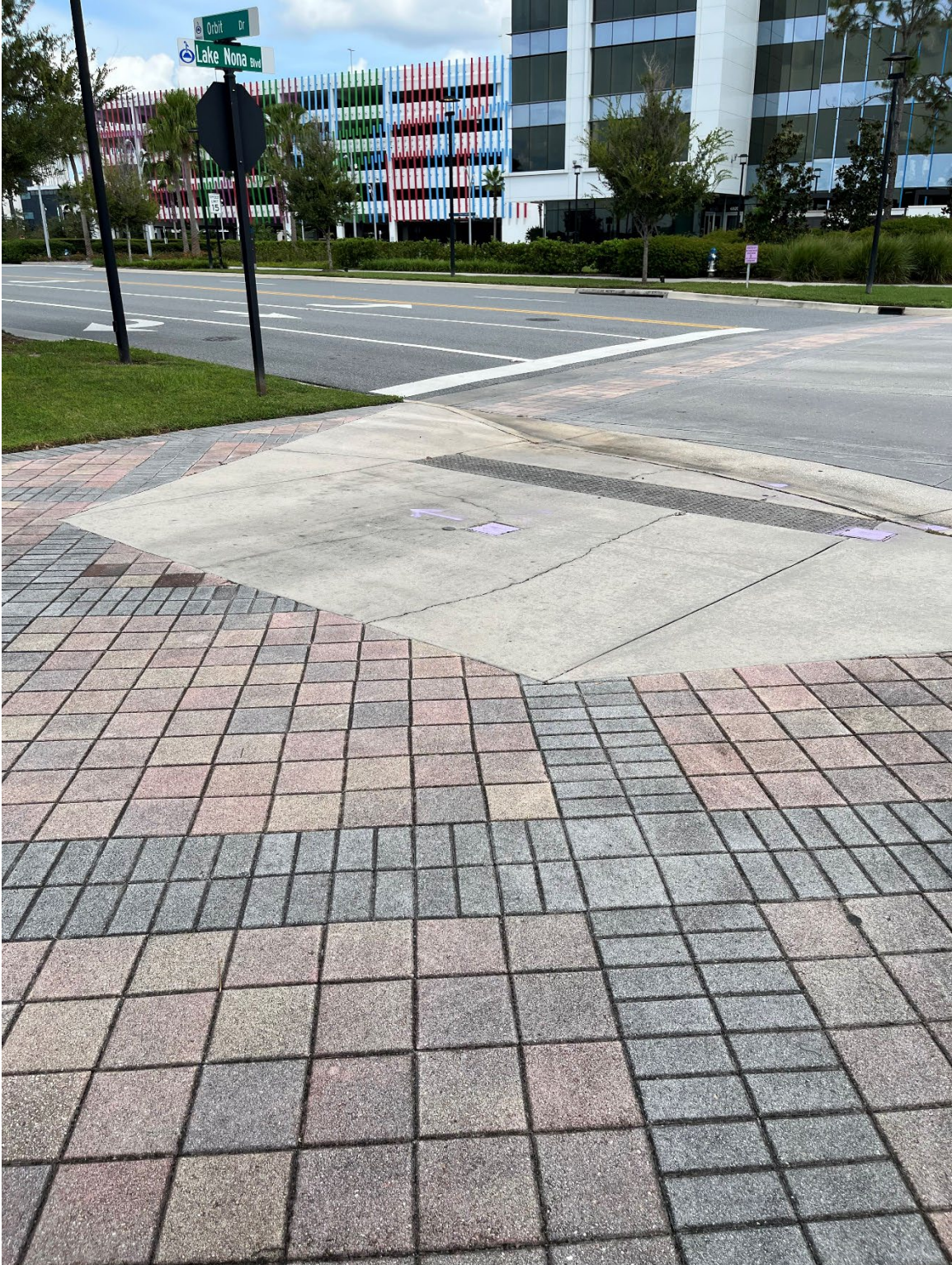
Photo 20 – Surficial Concrete Cracks in Handicap Ramp
