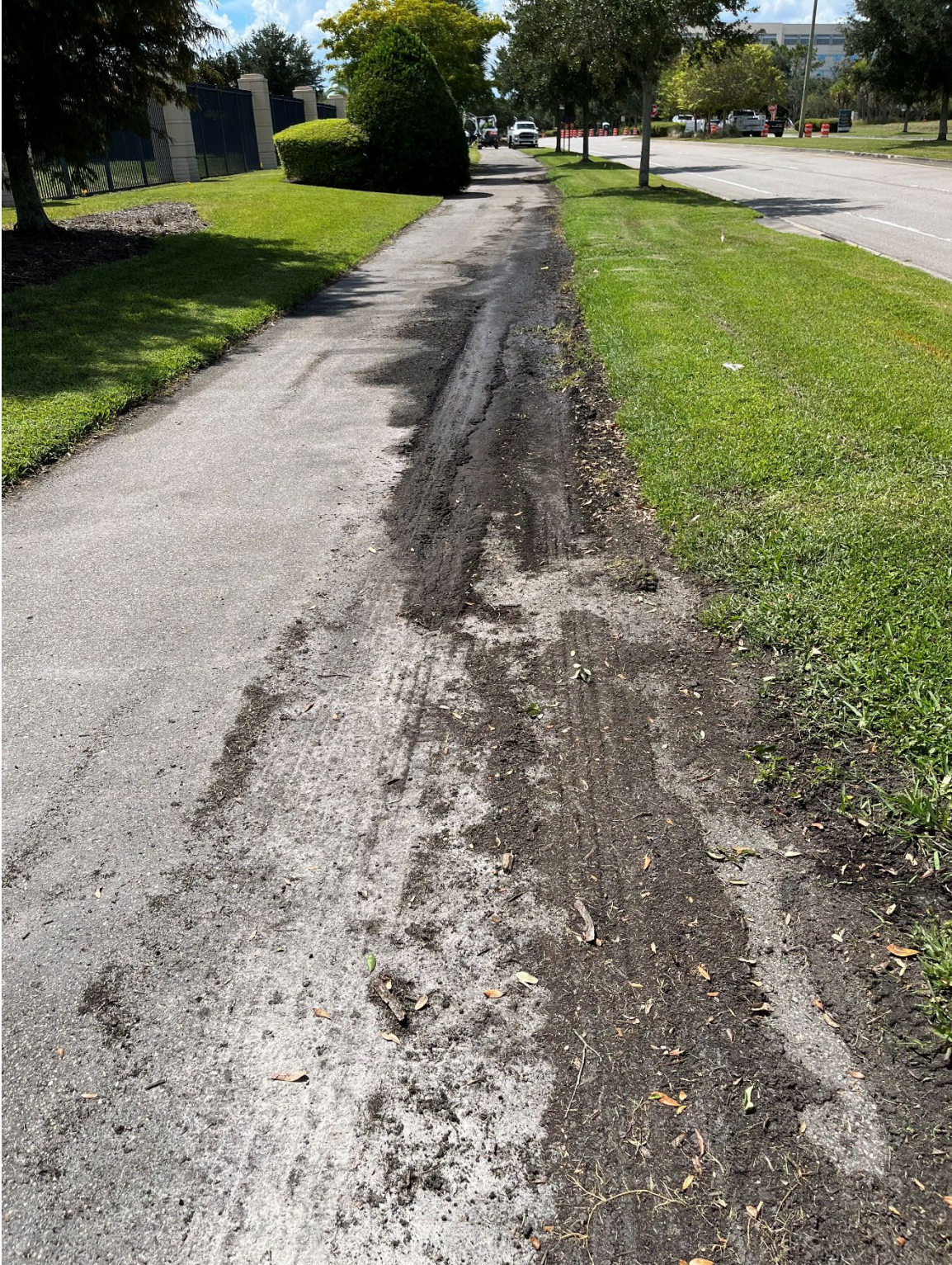
Photo 64 - Poor Drainage Area
