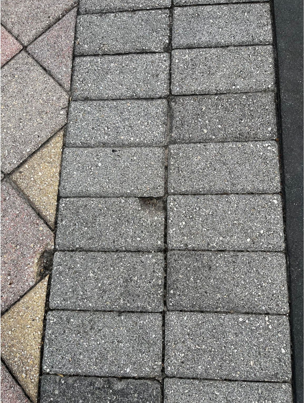
Photo 45 - Multiple Chipped Pavers
