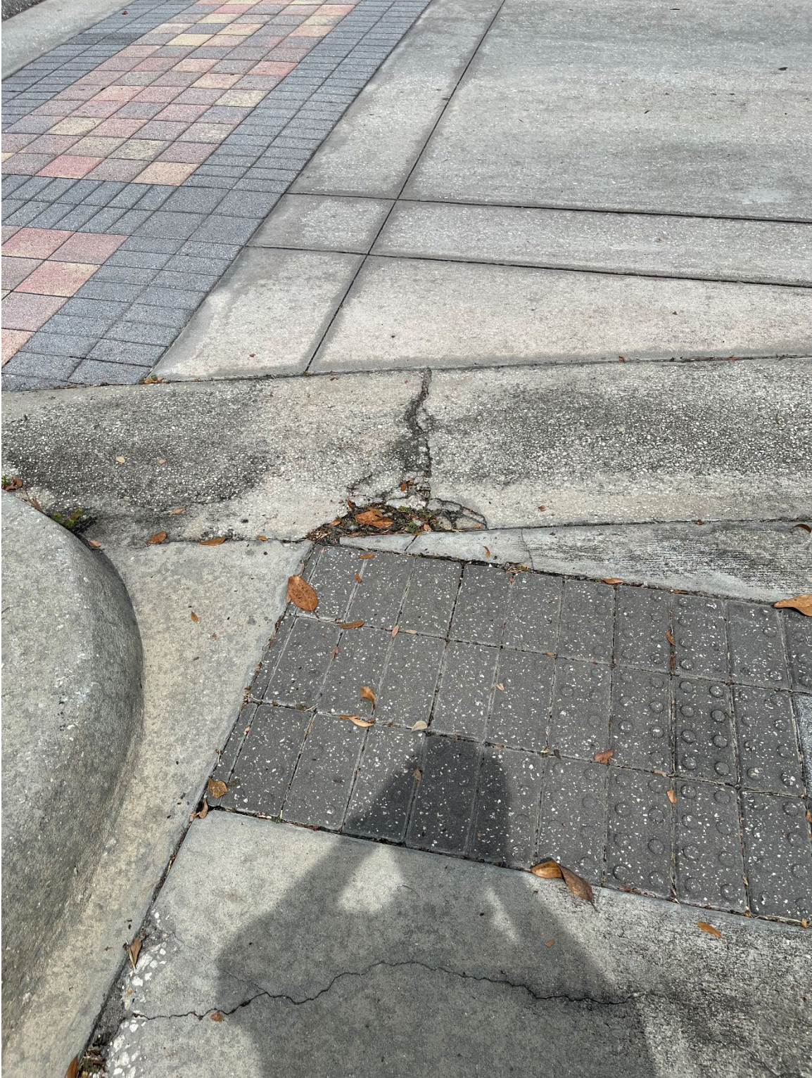
Photo 30 - Cracked Concrete in East Median
