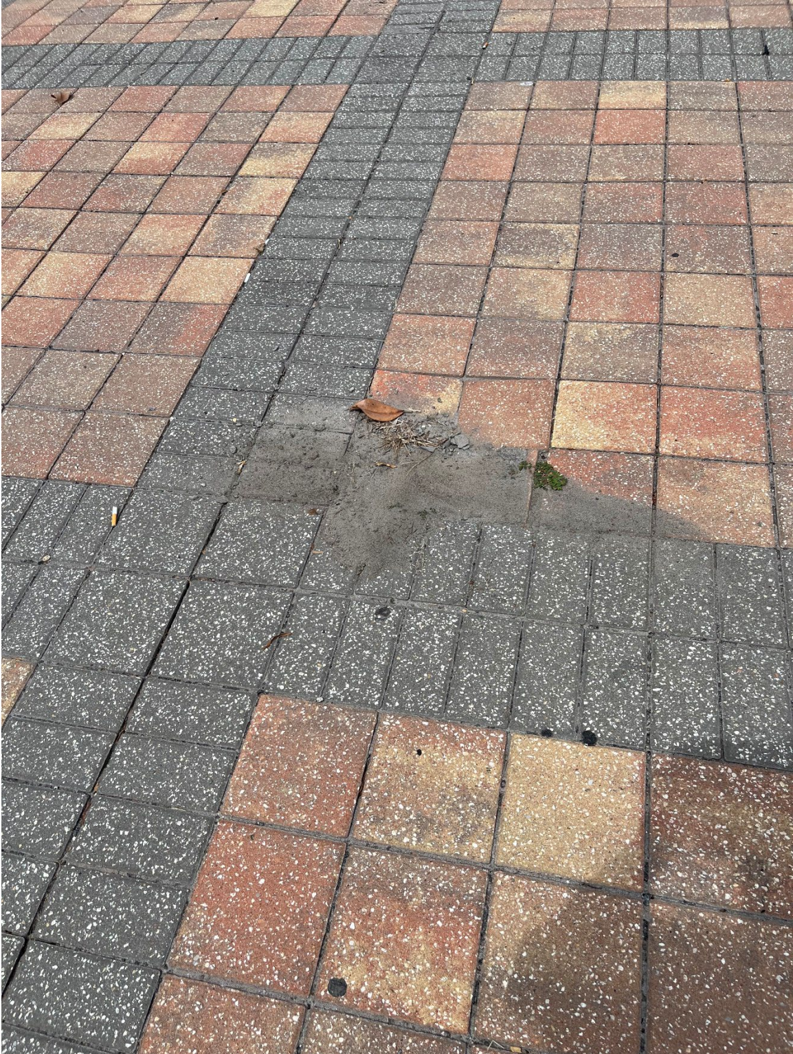
Photo 54 - Paver Base Failure in Median
