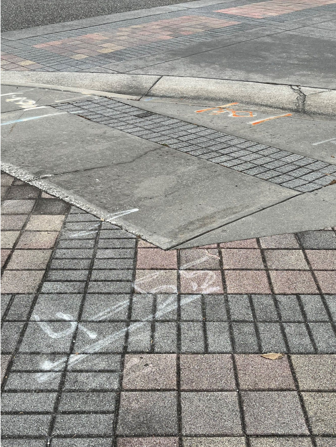
Photo 35 – Surficial Concrete Cracks in Handicap Ramp
