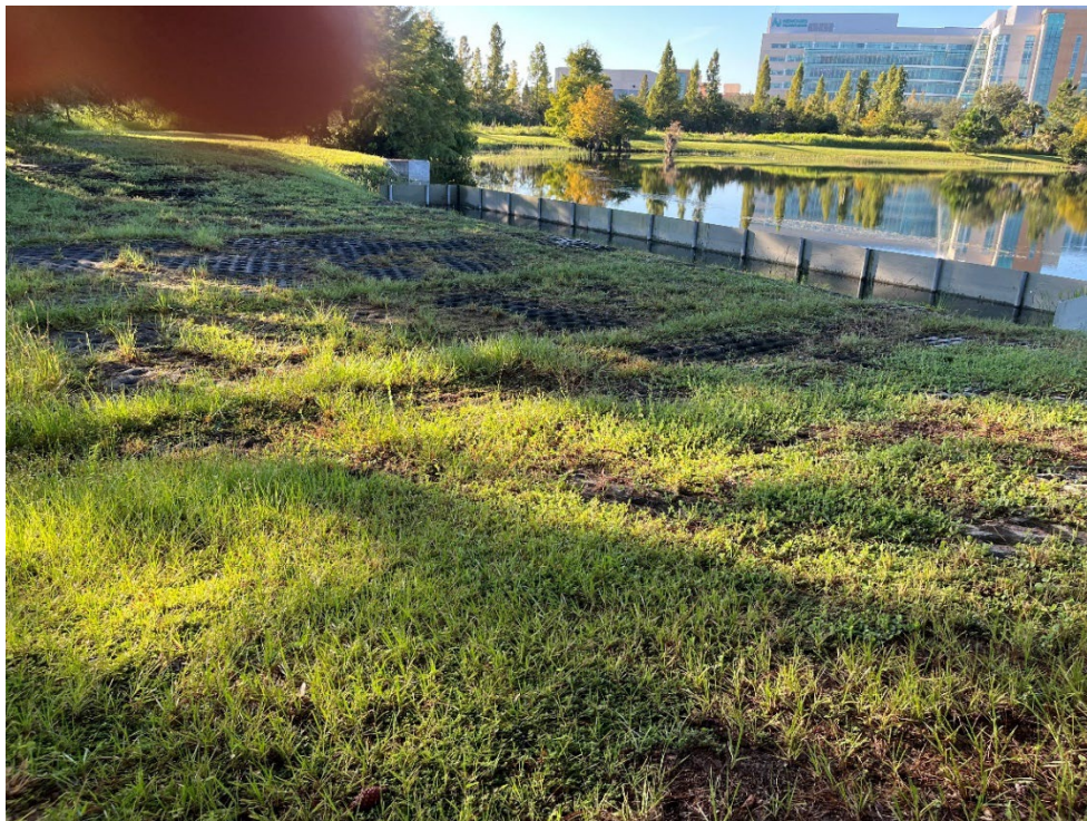
Photo 87 –Weir on NE Corner in Good Condition
