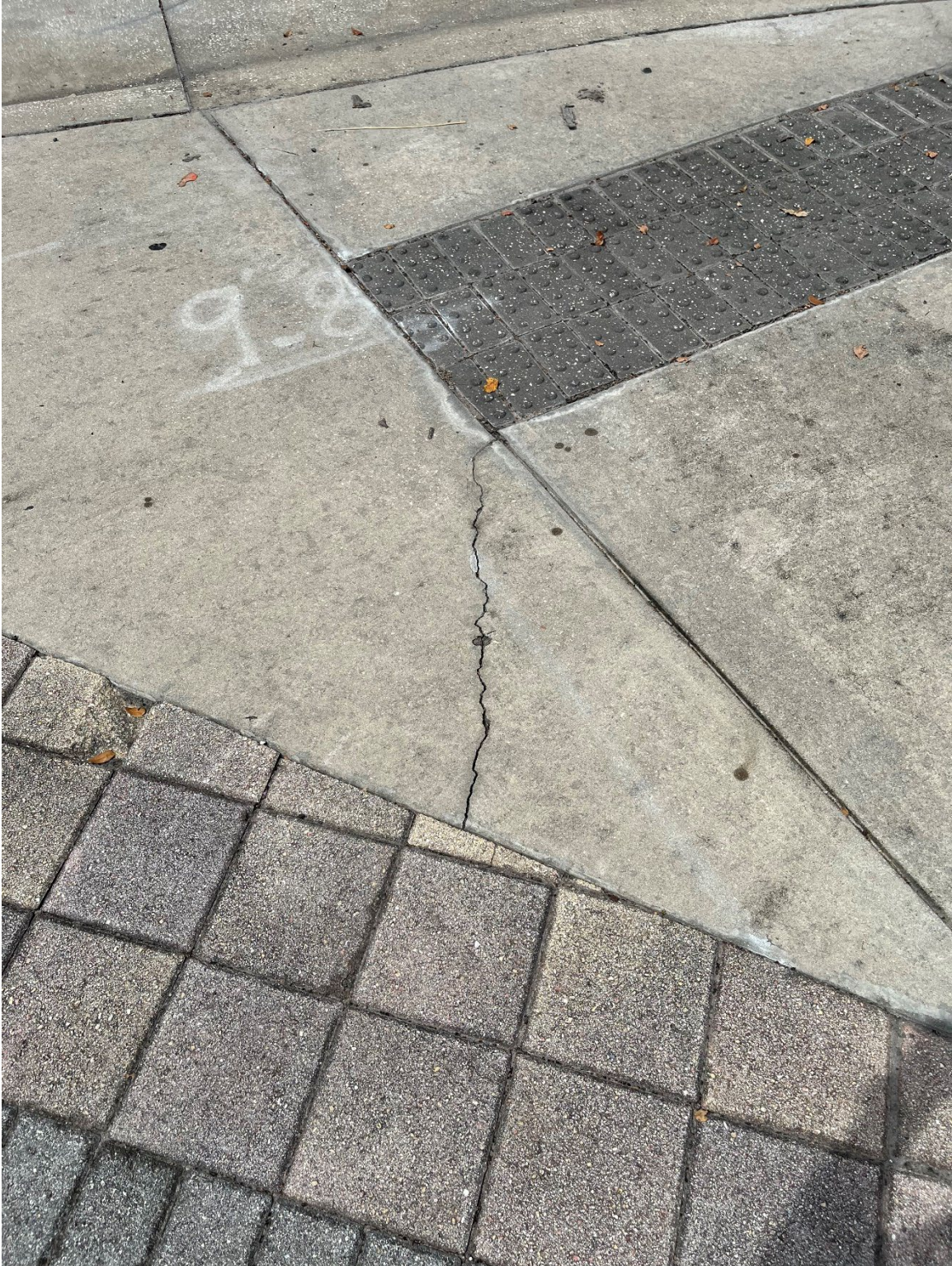
Photo 49 - Surficial Concrete Crack in Handicap Ramp
