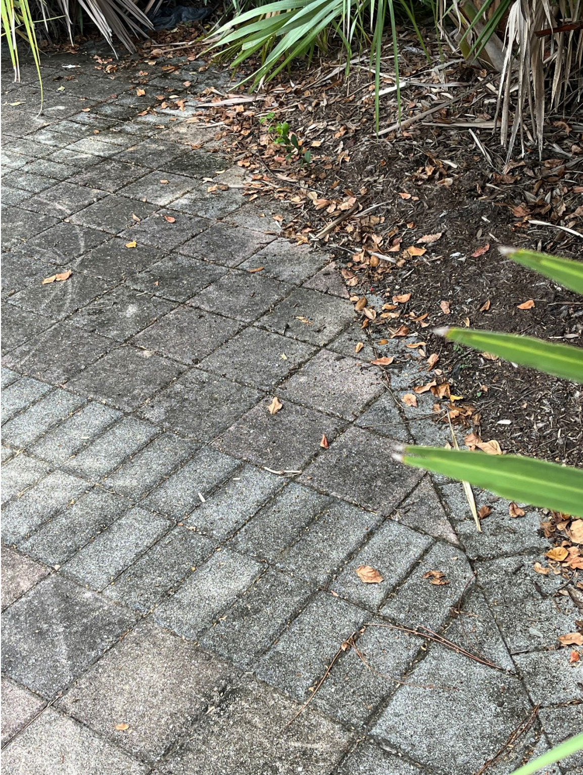
Photo 36 - Soil Covering Pavers
