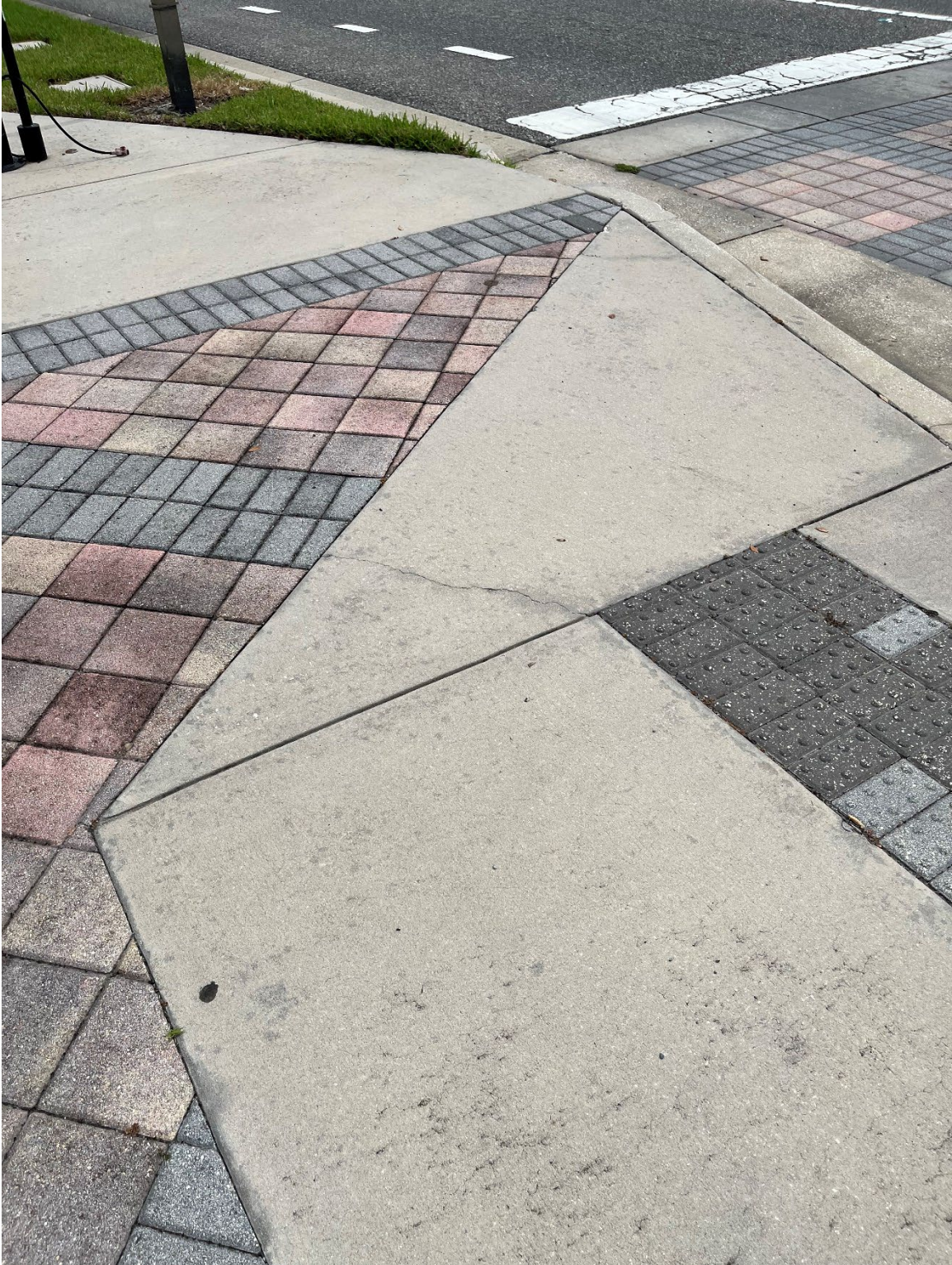
Photo 32 - Surficial Concrete Crack in Handicap Ramp
