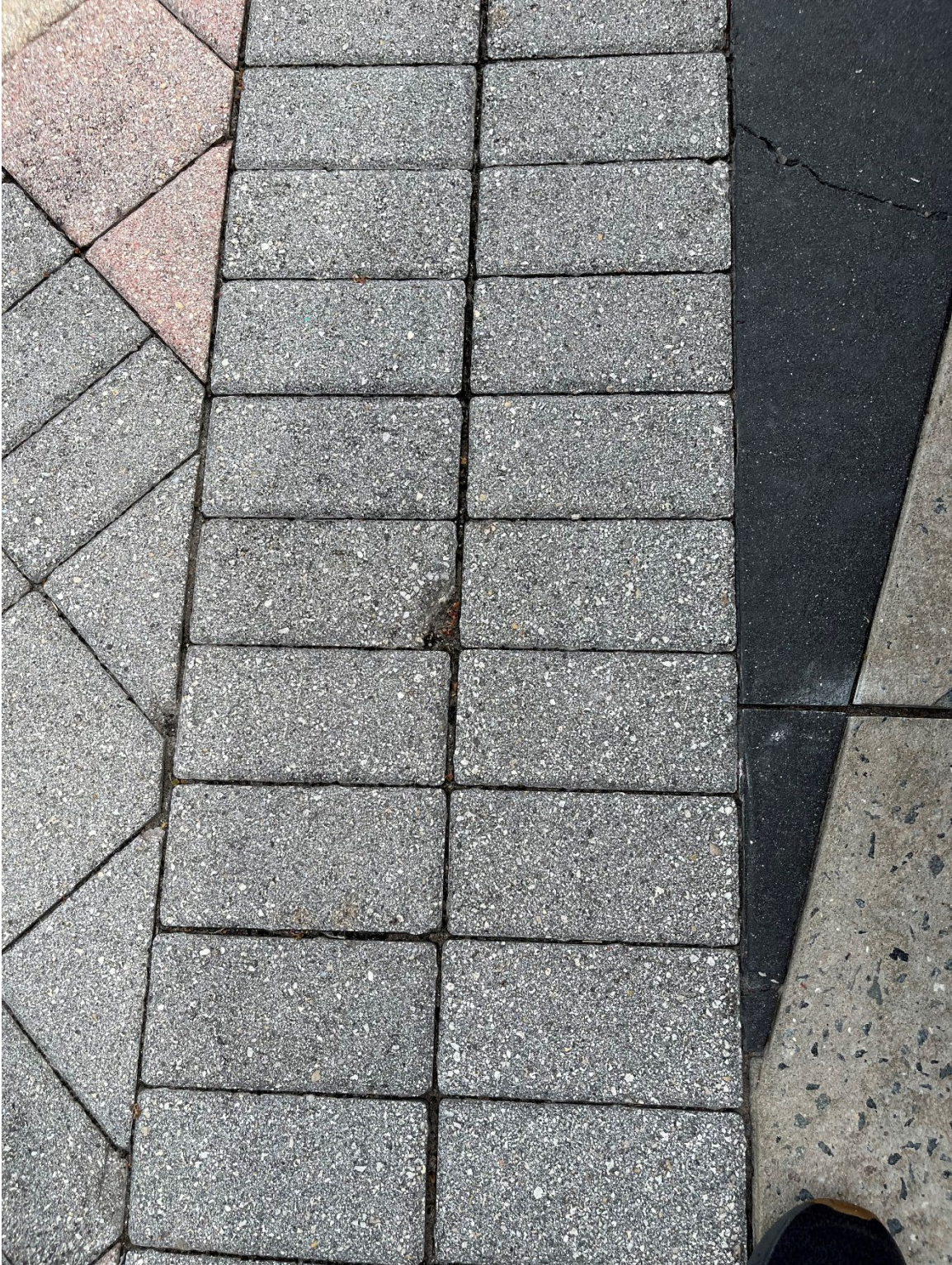
Photo 44 - Multiple Chipped Pavers
