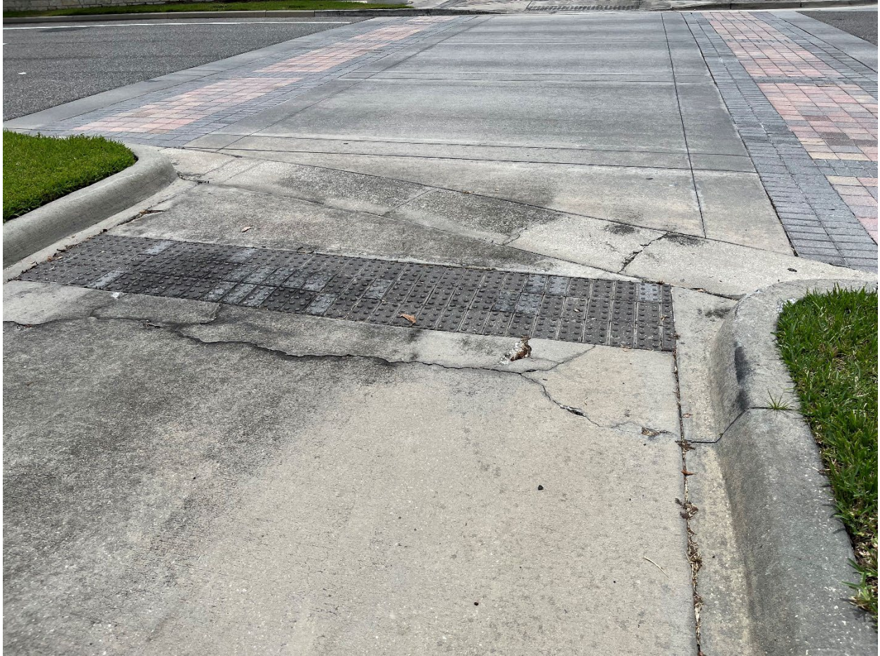
Photo 29 - Surficial Concrete Cracks
