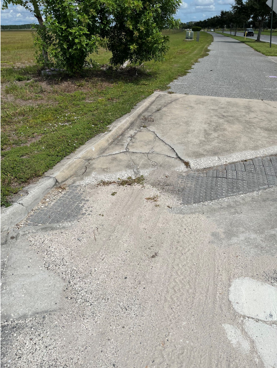
Photo 10 – Surficial Concrete Cracks in Handicap Ramp on East and West Side of Driveway Apron
