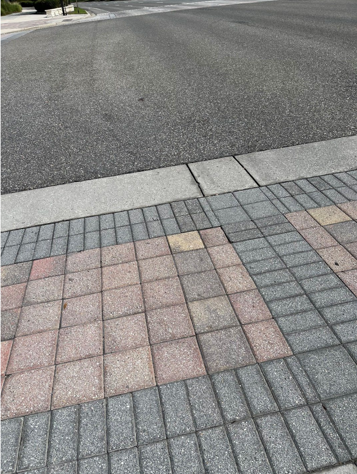
Photo 103 – Minor Settling
