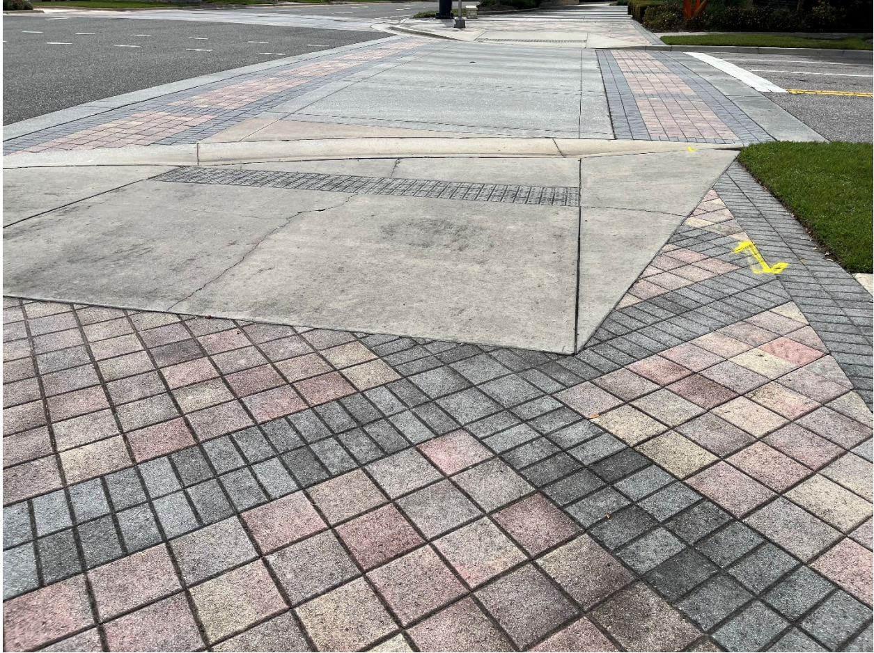
Photo 48 - Surficial Concrete Cracks in Handicap Ramp
