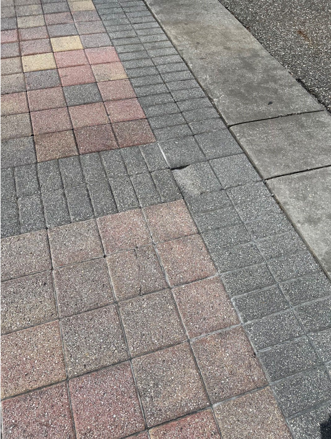
Photo 95 – Cracked Pavers - Minor Settling
