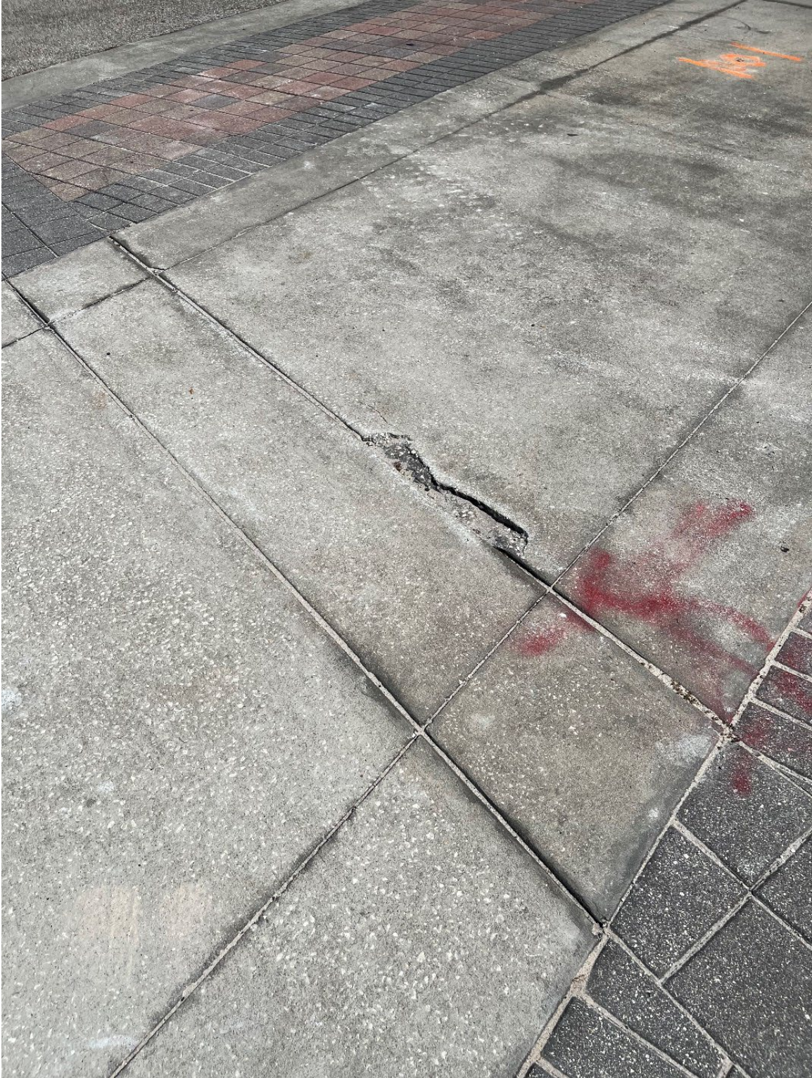
Photo 124 – Broken Concrete
