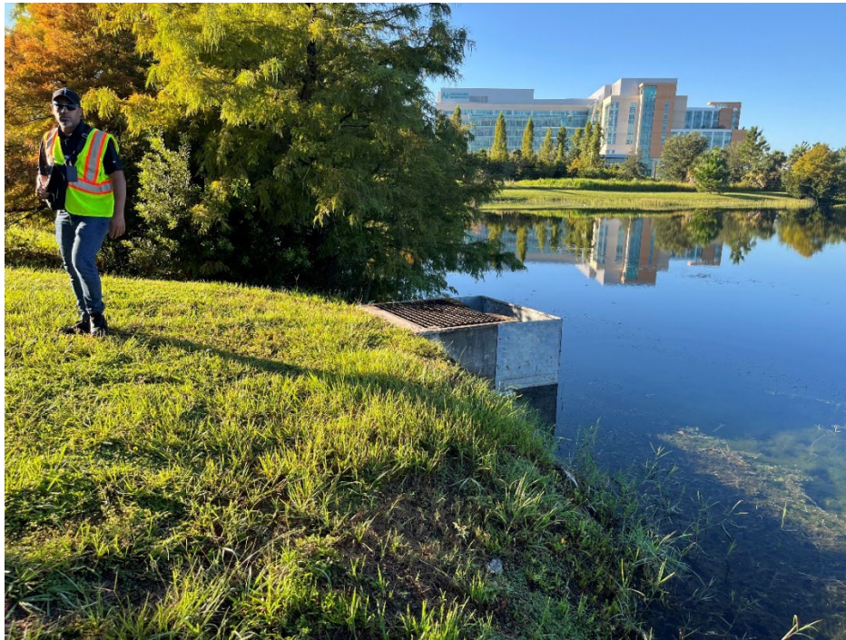
Photo 88 – Outfall Structure in Good Condition
