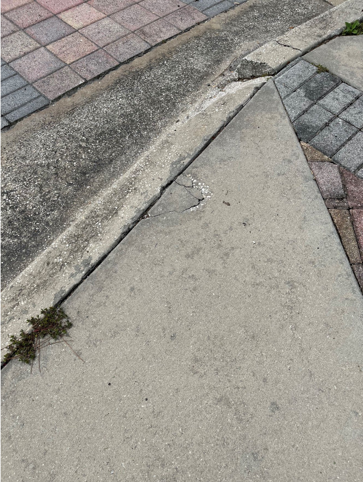
Photo 23 - Cracked Concrete in Handicap Ramp
