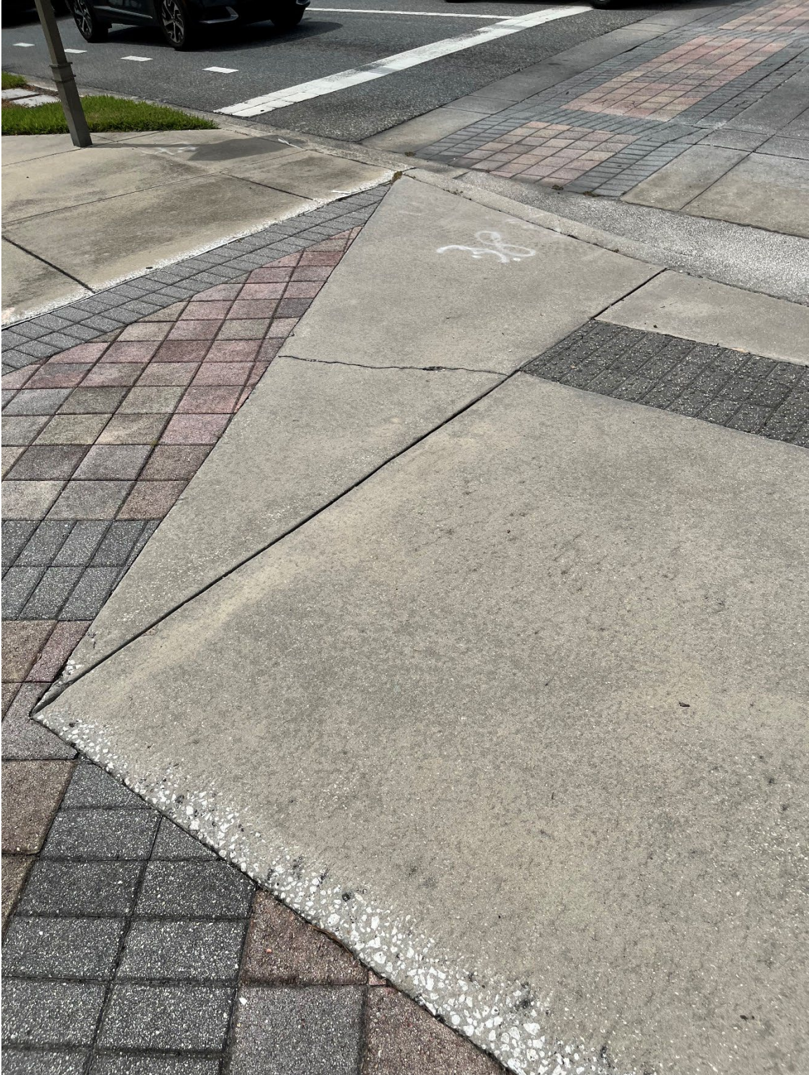
Photo 14 – Surficial Concrete Crack in Handicap Ramp
