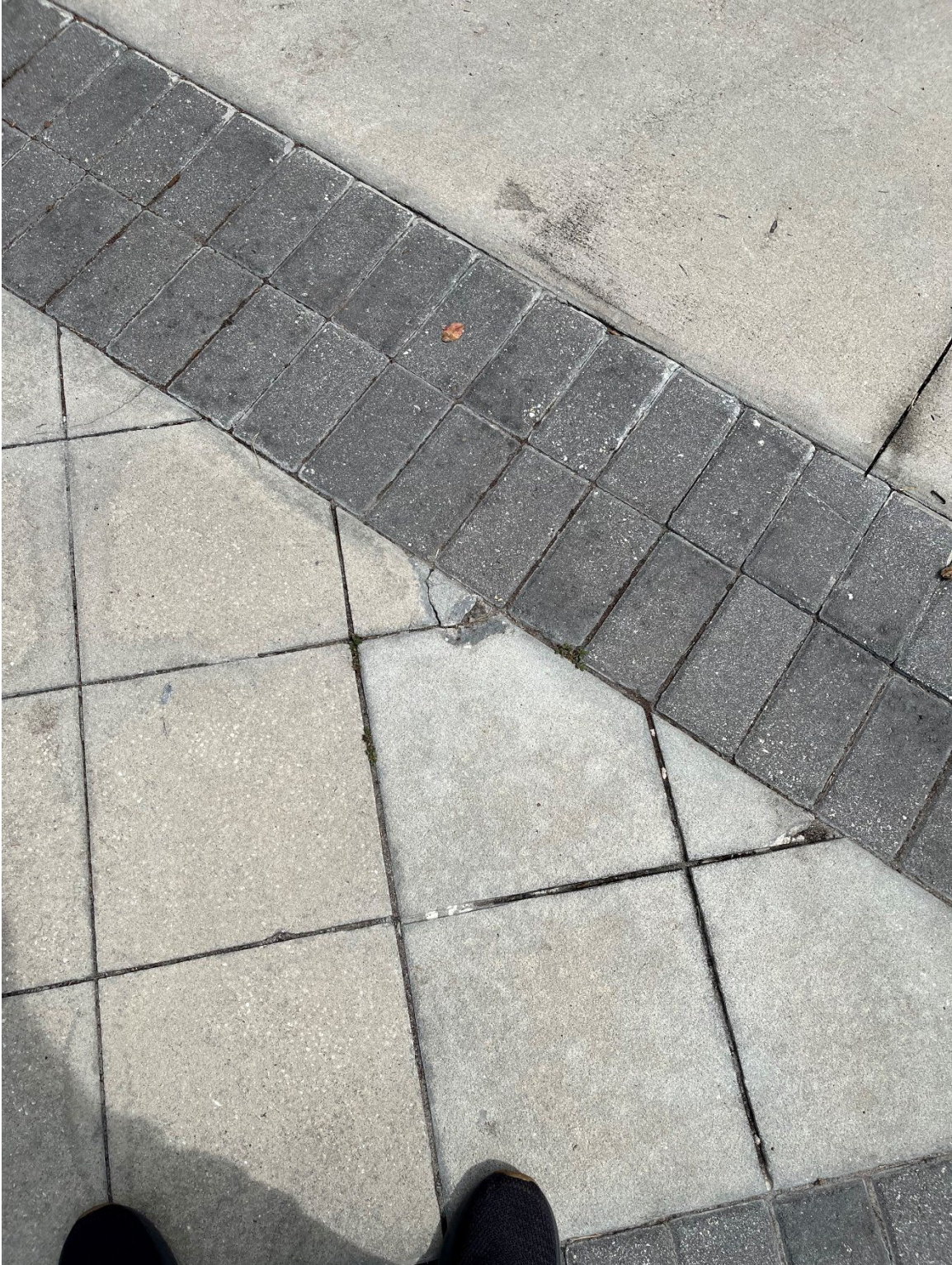
Photo 46 – Multiple Chipped Pavers
