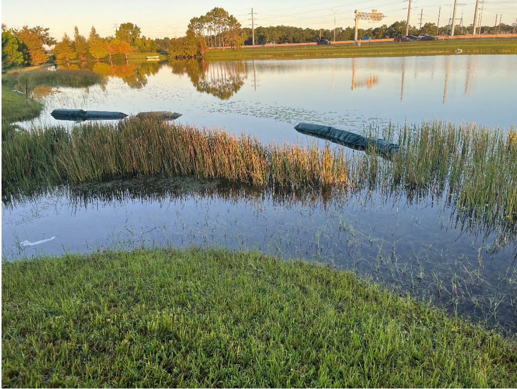
Photo 80 – Broken Floating Turbidity Barrier
