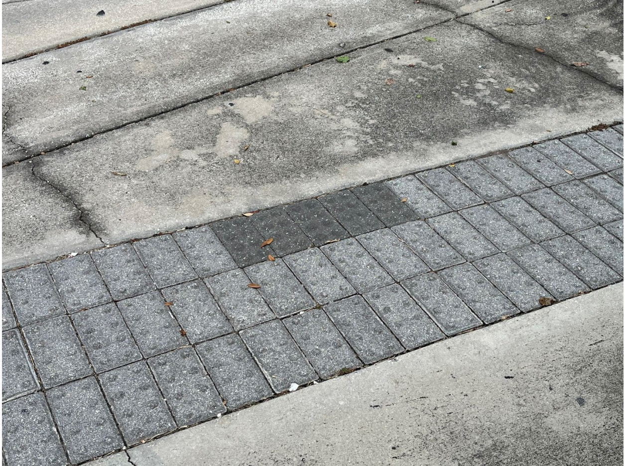
Photo 37 – Surficial Concrete Cracks in Median Strip
