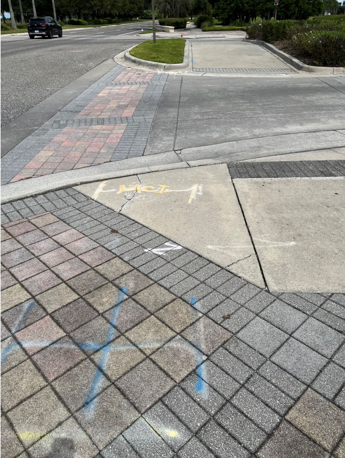
Photo 16 – Surficial Concrete Cracks in Handicap Ramp
