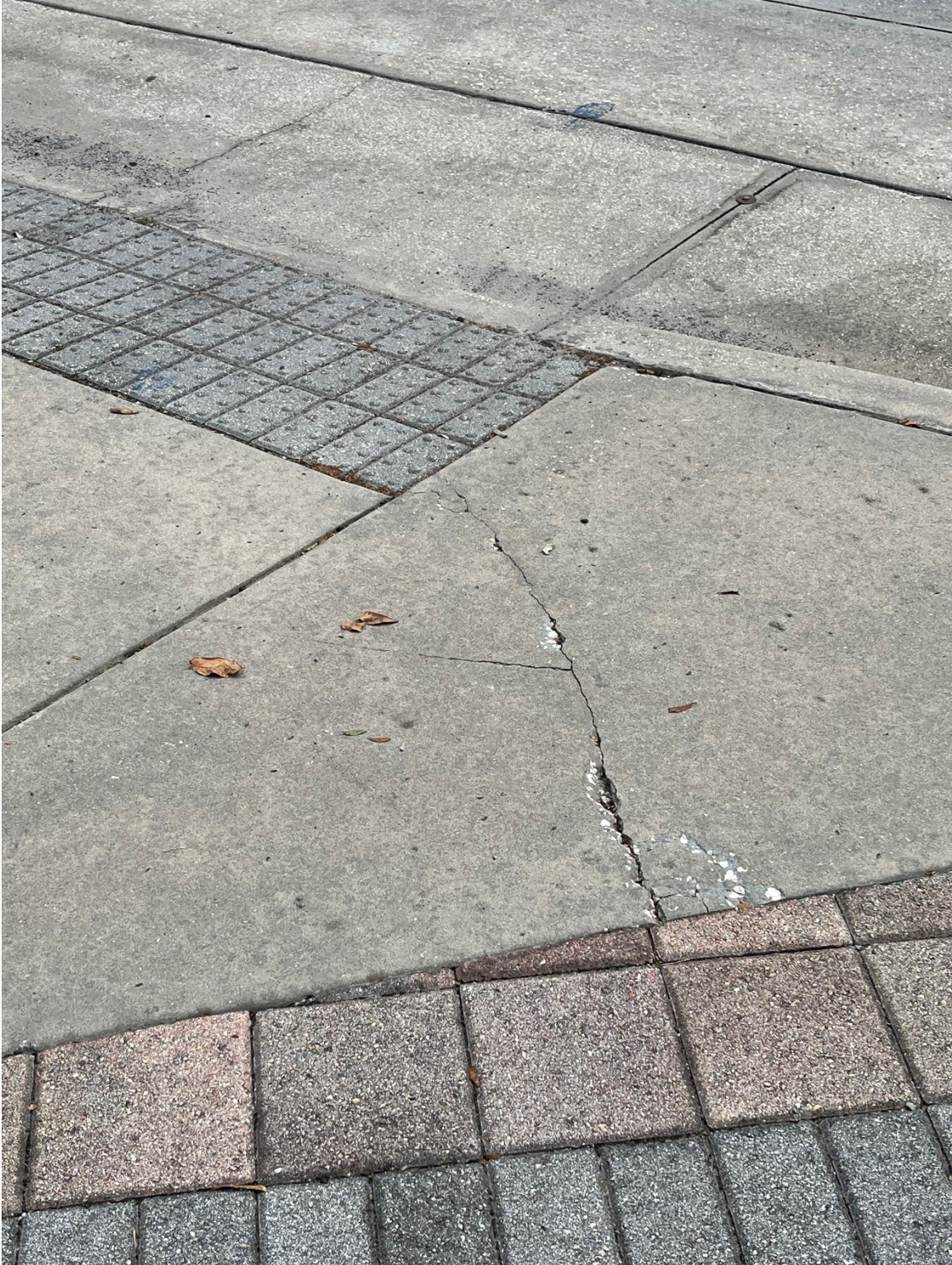
Photo 41 - Surficial Concrete Cracks in Handicap Ramp
