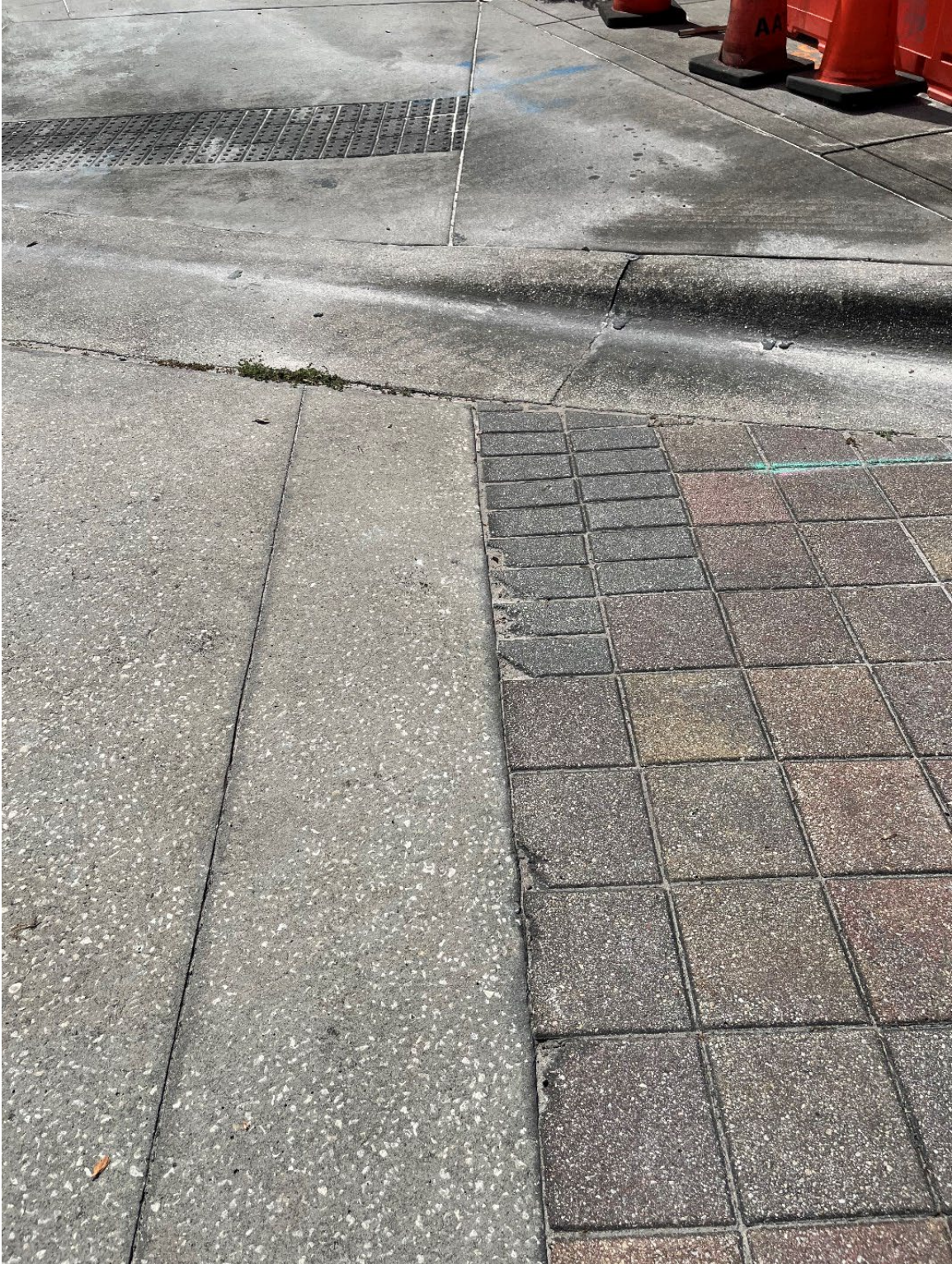
Photo 123 – Cracked Pavers
