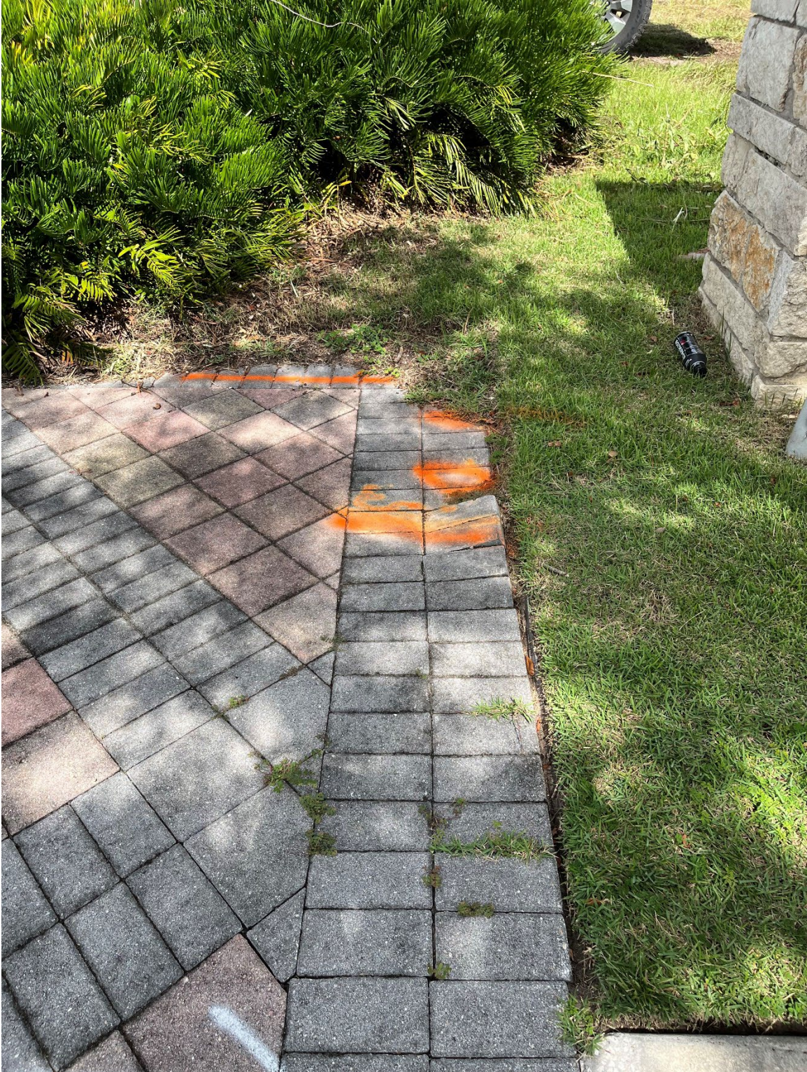
Photo 69 - Paver Base Failure
