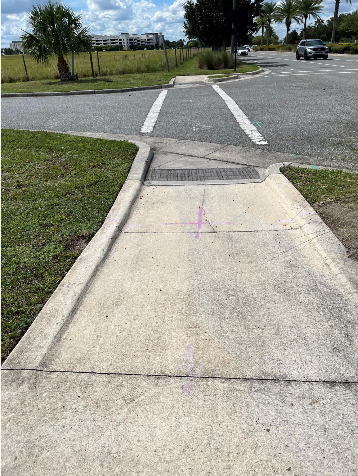
Photo 61 – Surficial Concrete Cracks in Handicap Ramp
