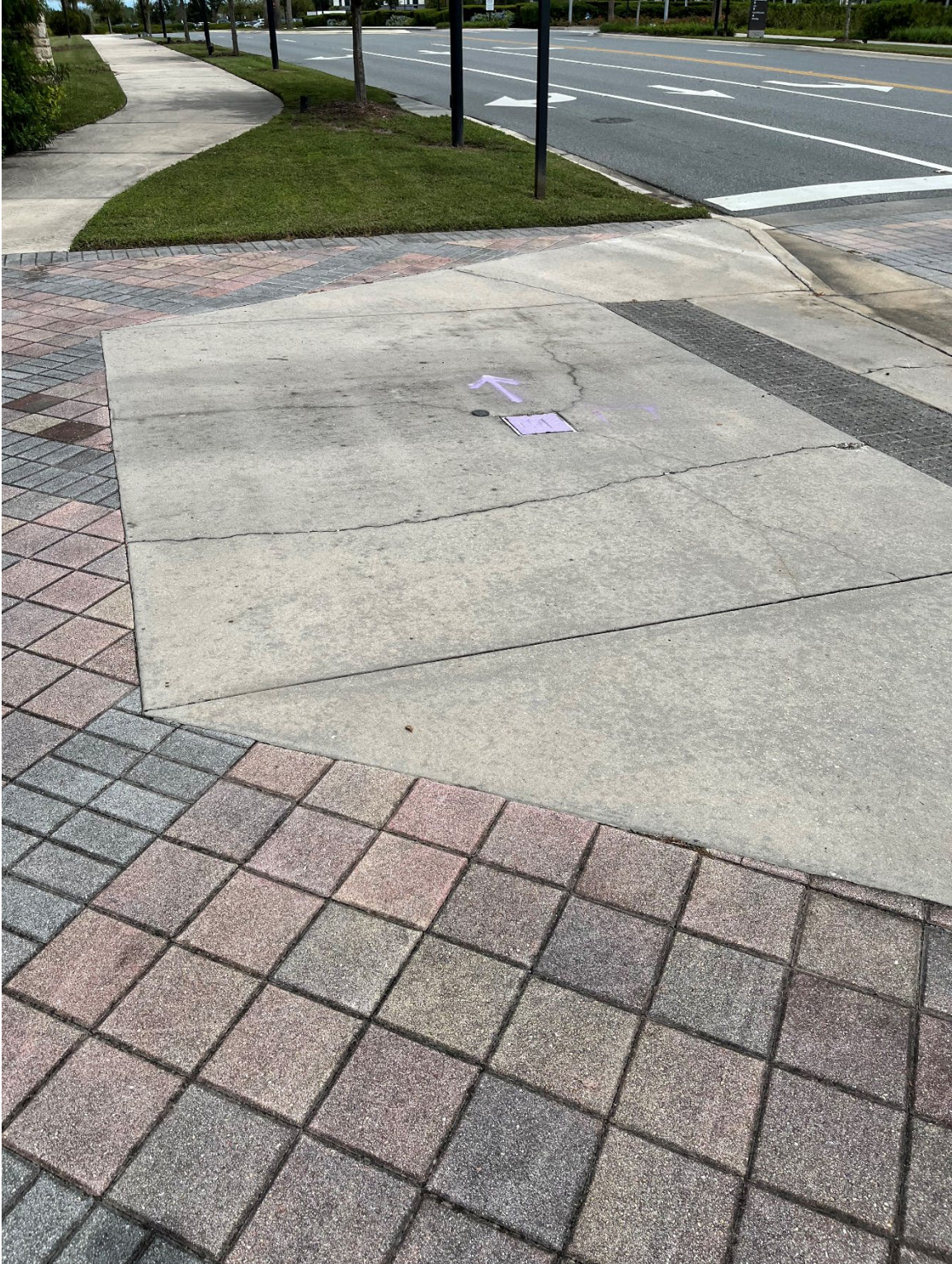
Photo 22 – Surficial Concrete Cracks in Handicap Ramp
