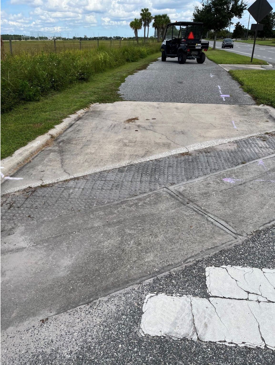
Photo 13 – Surficial Concrete Cracks in Handicap Ramp on East and West Side of Driveway Apron
