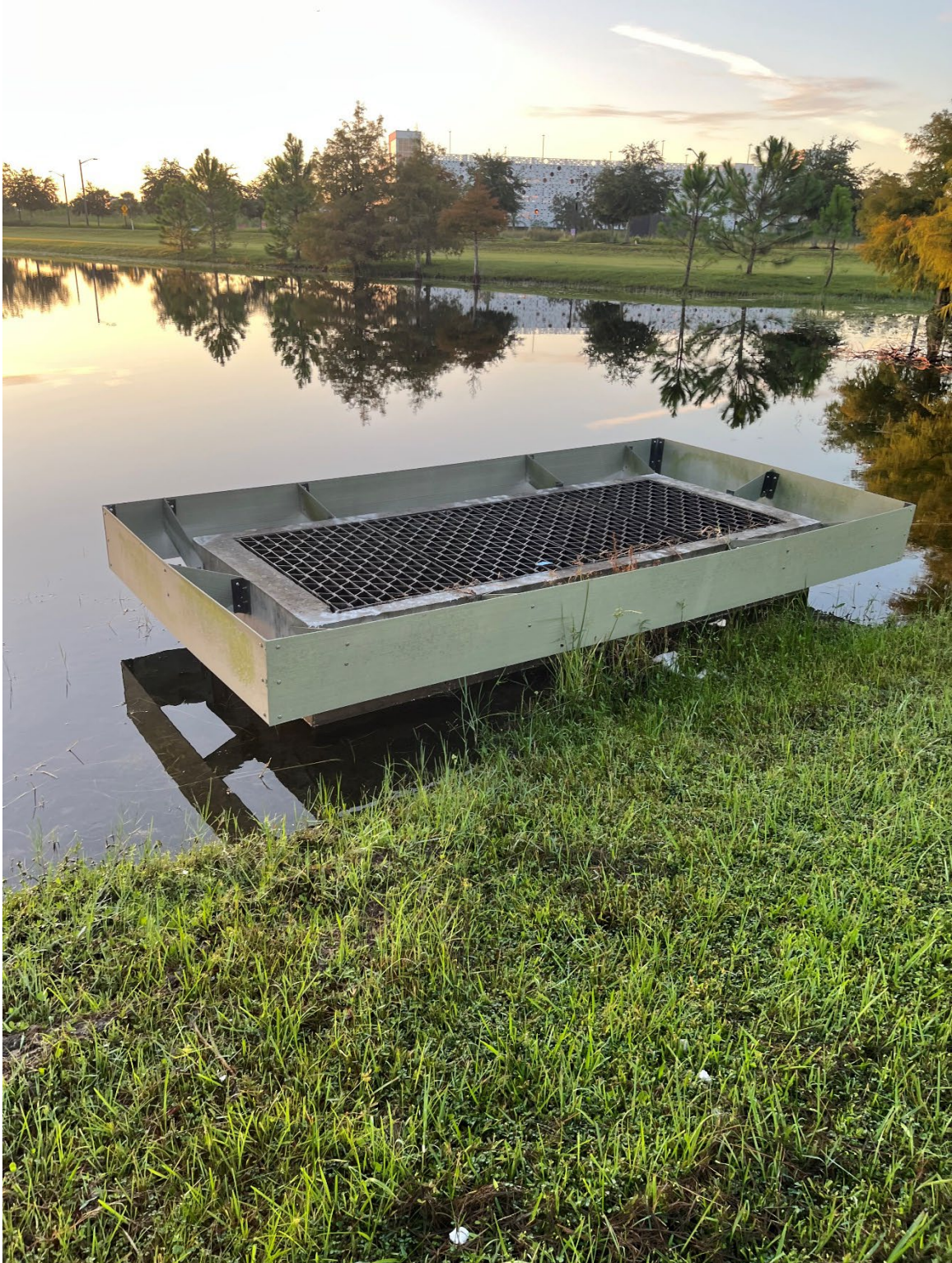
Photo 74 – Pond Outfall Structure in Good Condition
