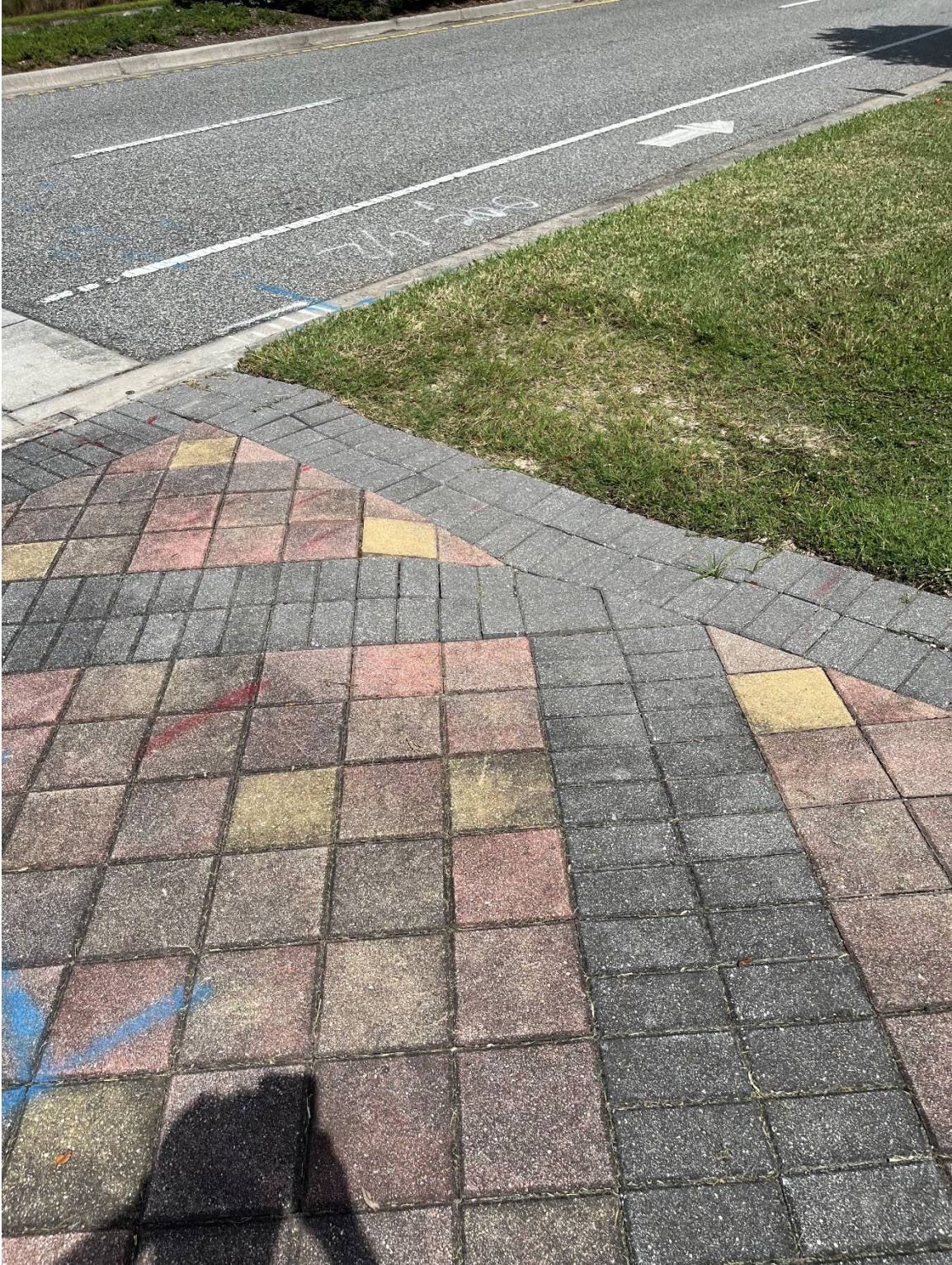
Photo 60 - Paver Base Failure
