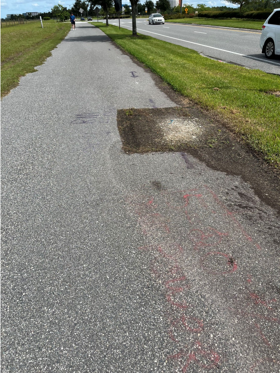
Photo 9 – Asphalt Cutout and Removed
