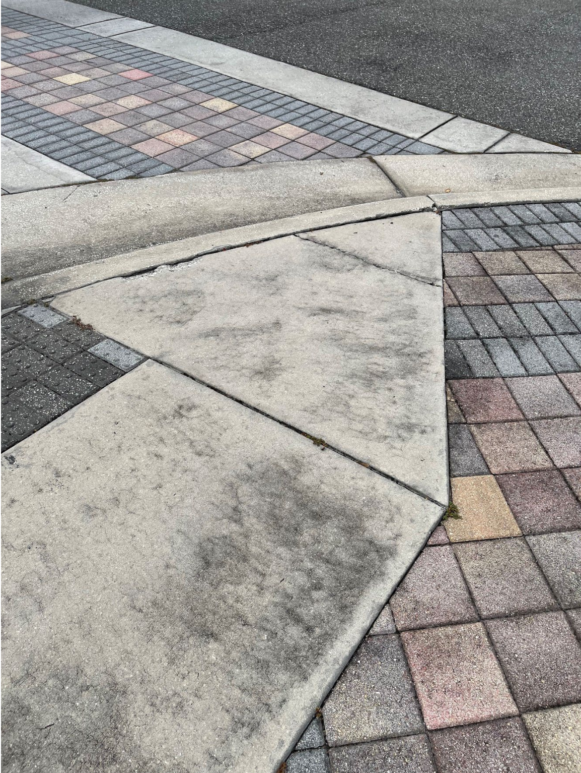
Photo 31 – Surficial Concrete Crack in Handicap Ramp
