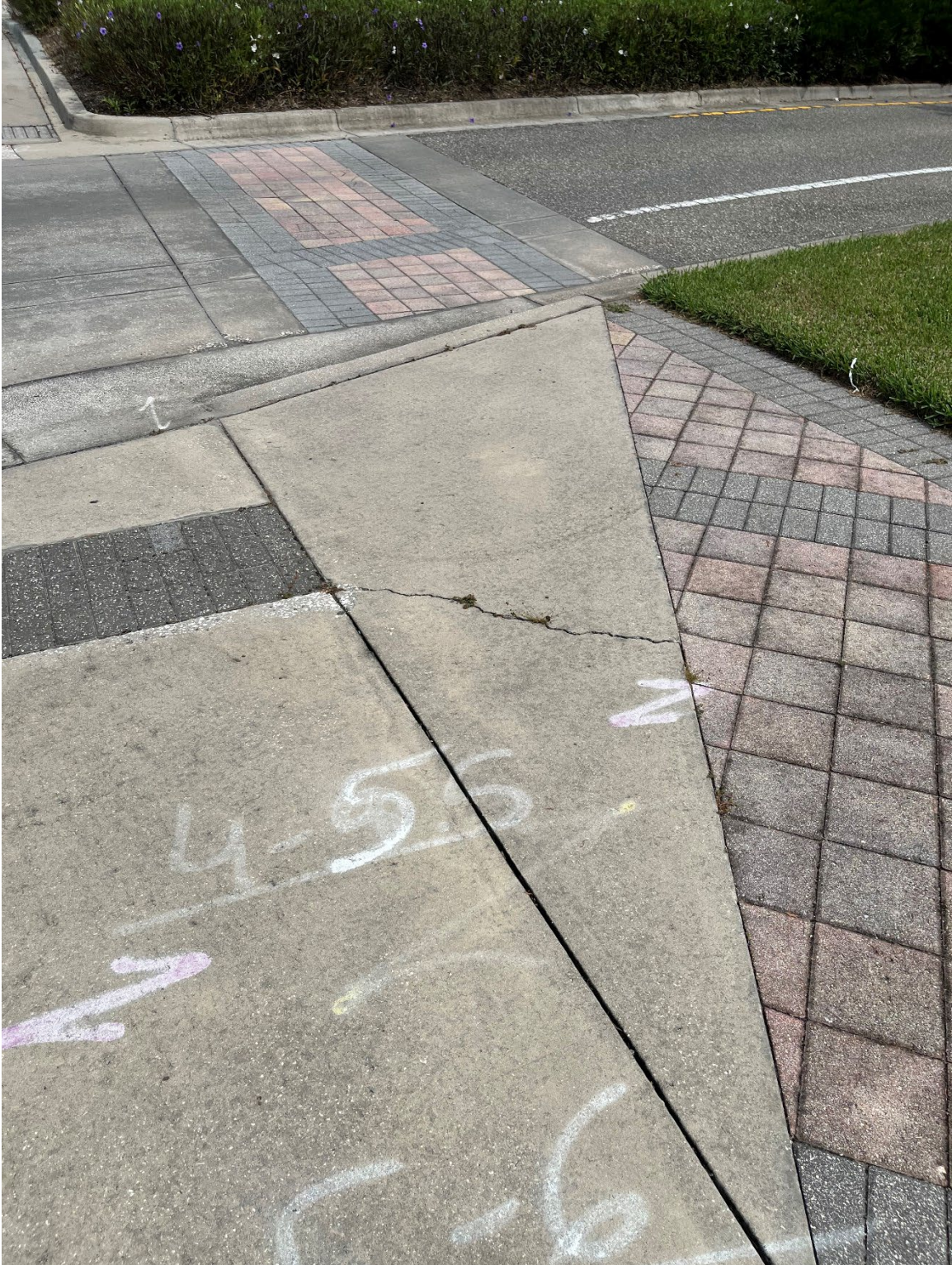
Photo 17 – Surficial Concrete Crack in Handicap Ramp
