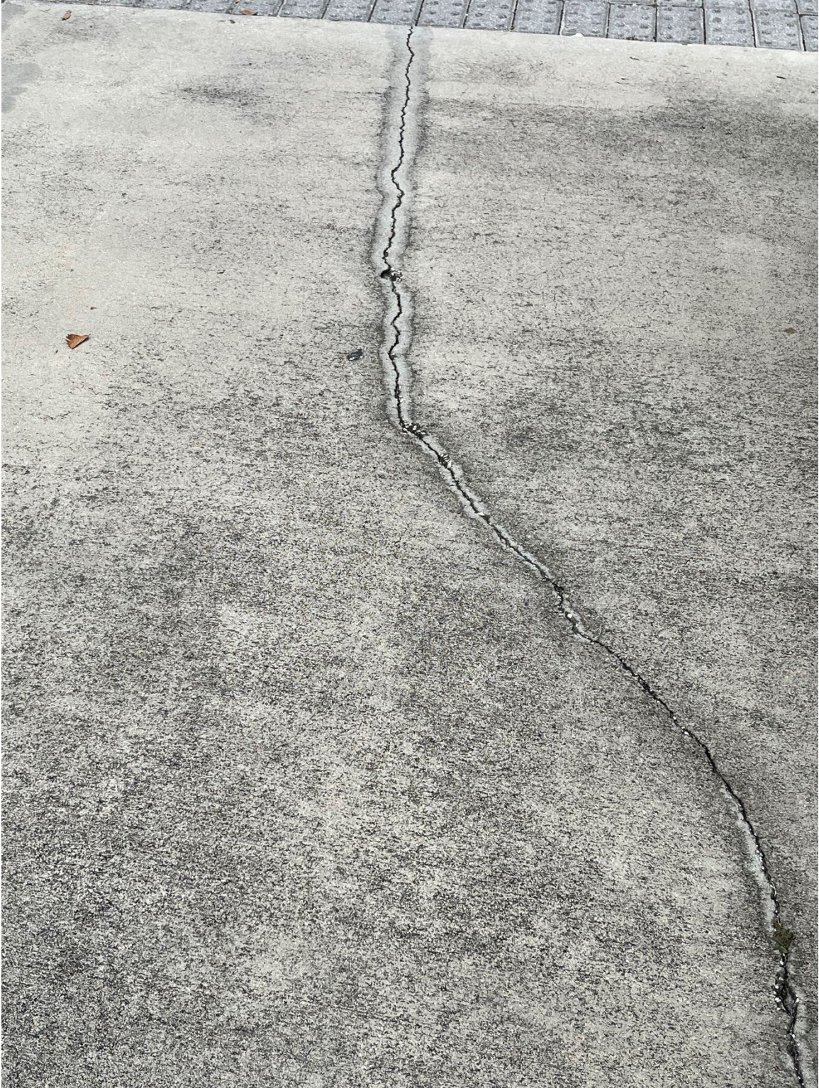
Photo 39 – Surficial Concrete Cracks in Median Strip
