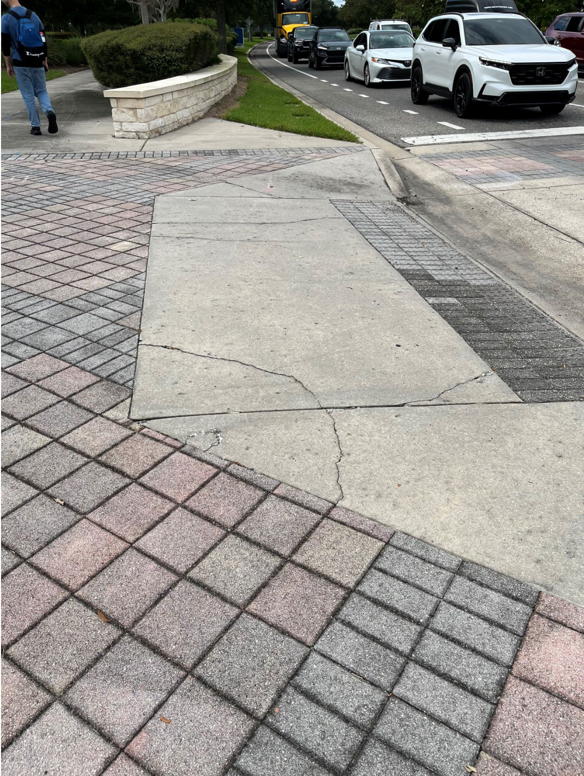
Photo 33 – Surficial Concrete Cracks in Handicap Ramp
