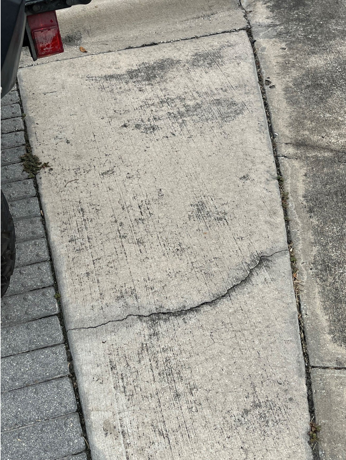
Photo 38 – Surficial Concrete Crack in Median Strip
