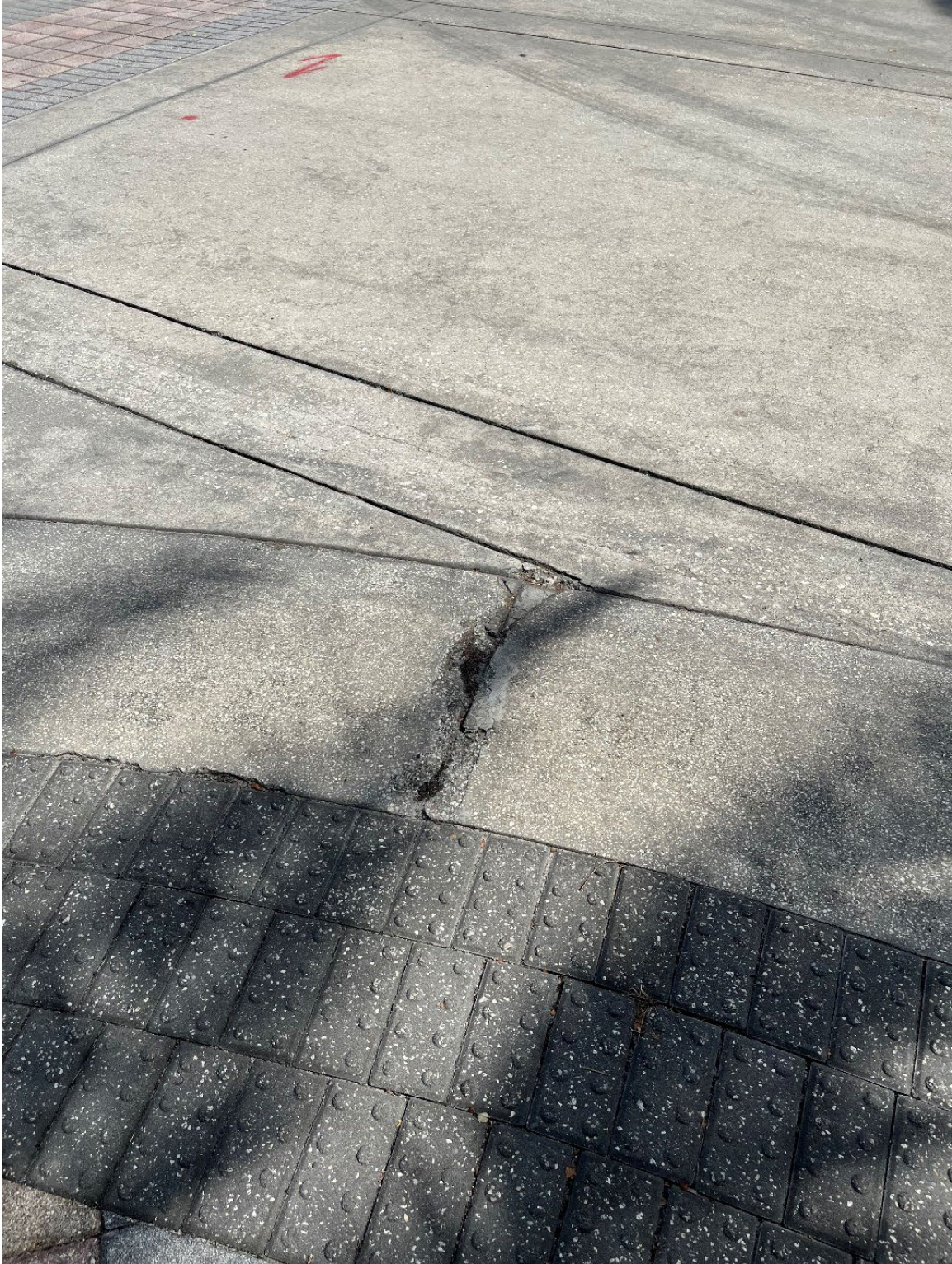
Photo 120 – Broken Concrete in Flush Curb
