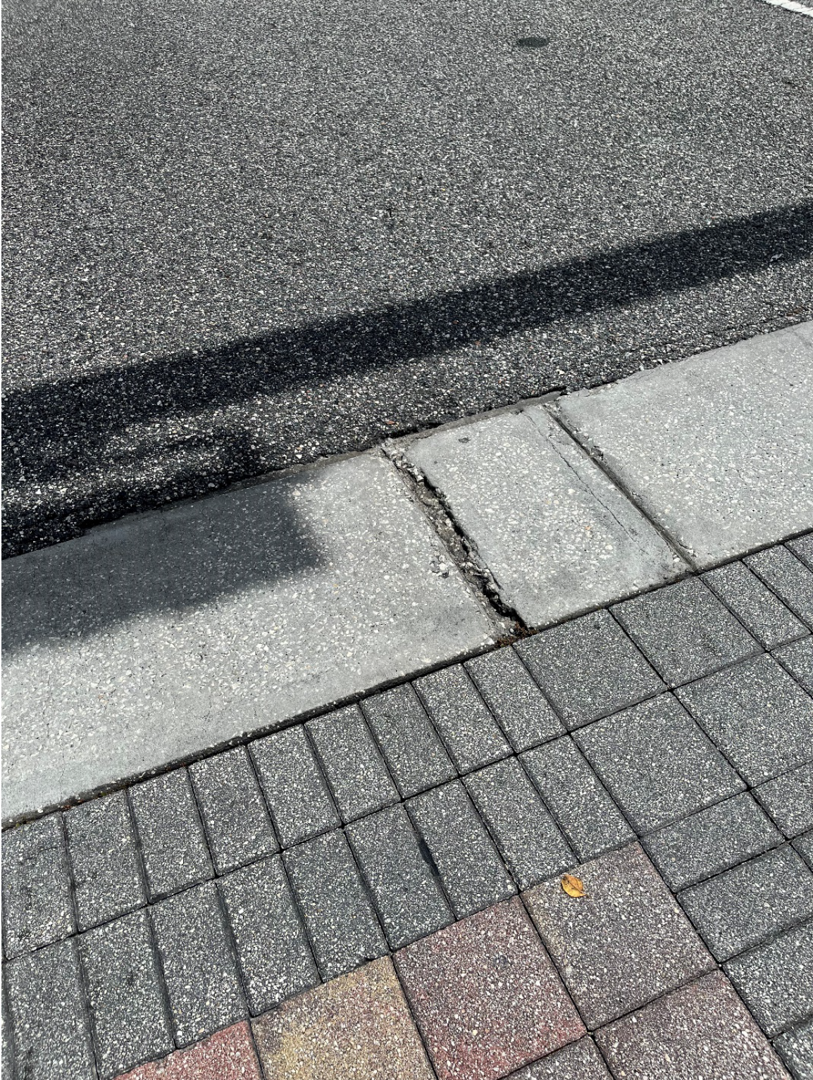
Photo 94 – Cracked Concrete - Minor Settling
