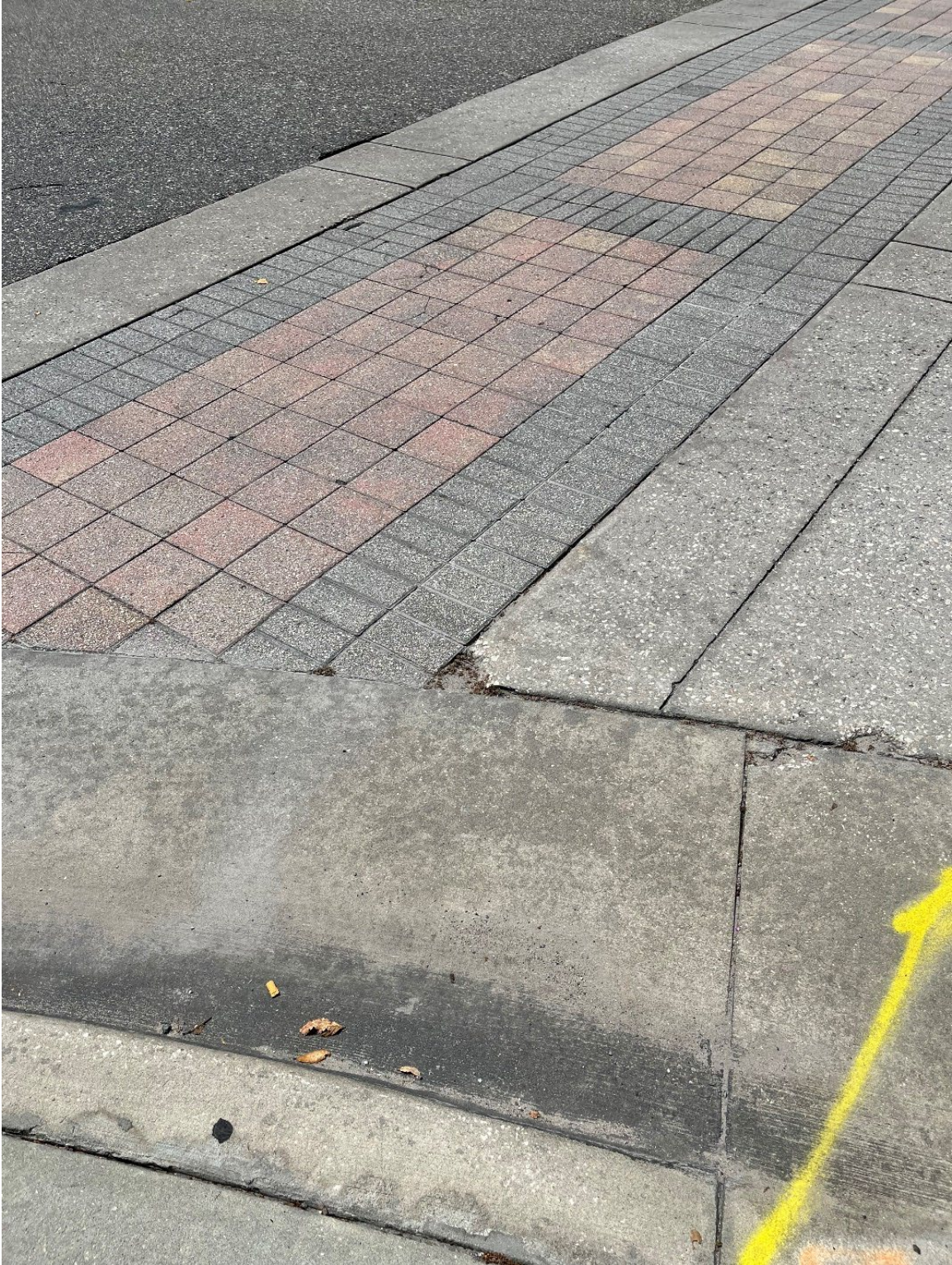
Photo 98 – Cracked Pavers – Broken Concrete
