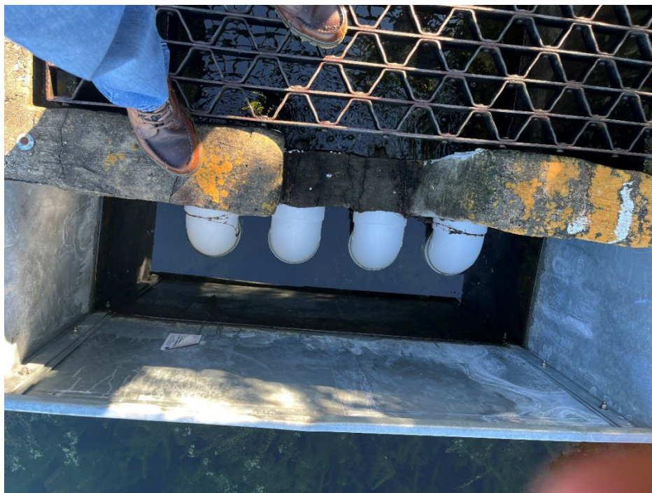
Photo 89 – Drawdown Pipe Inside of Outfall Structure
