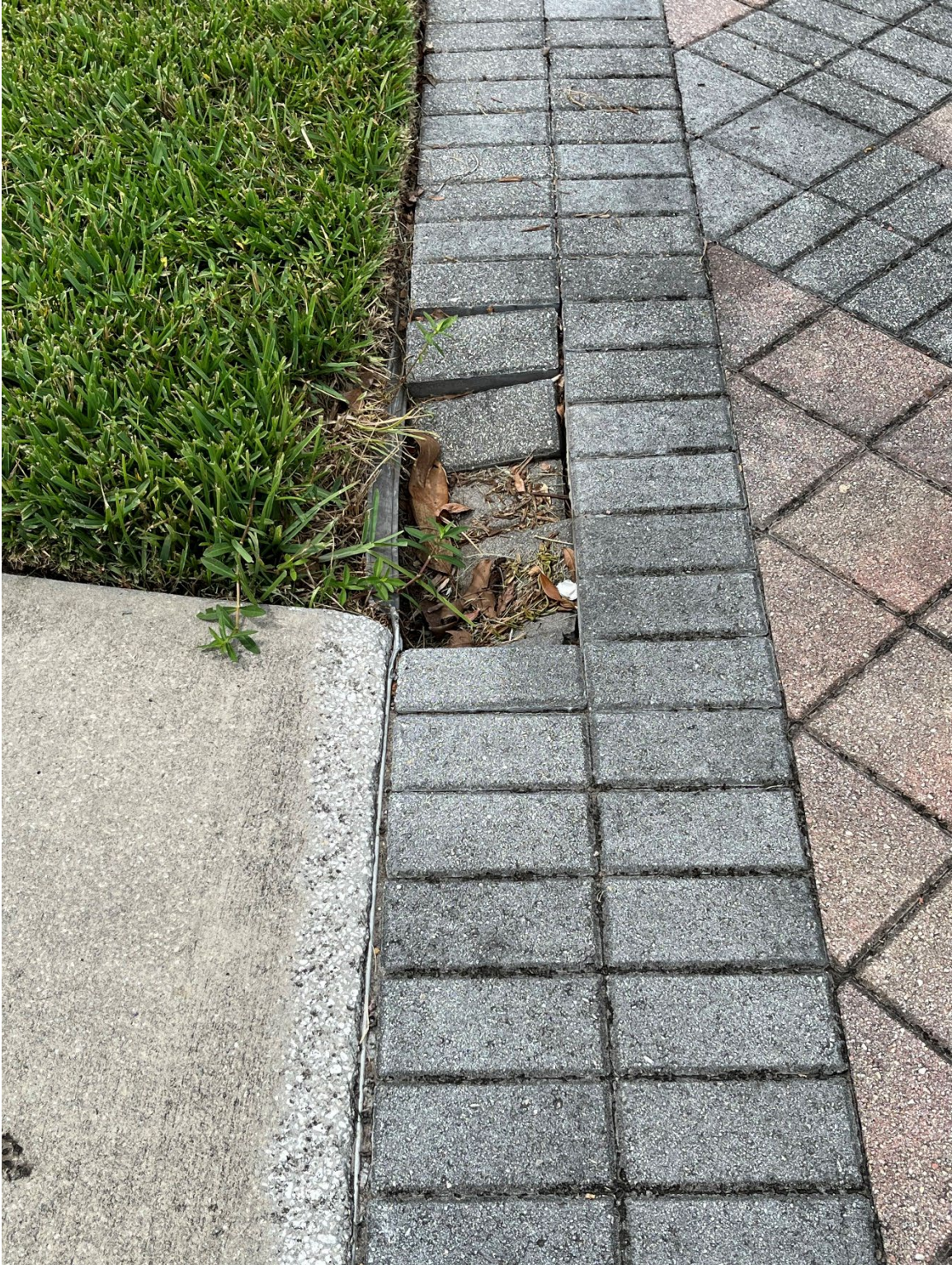
Photo 27 - Paver Base Failure
