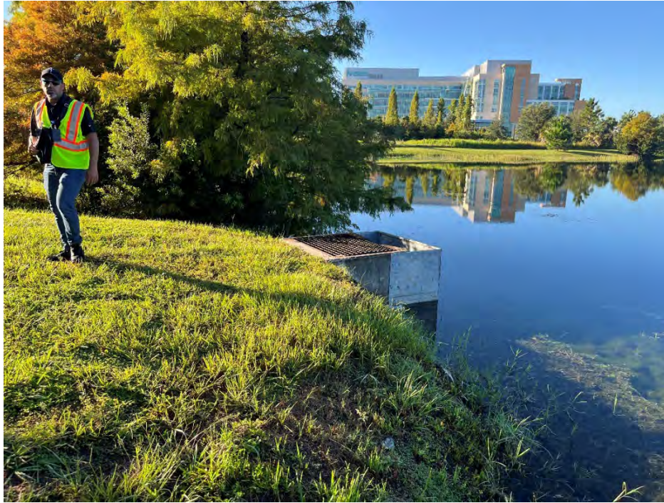
Photo 88 – Outfall Structure in Good Condition
