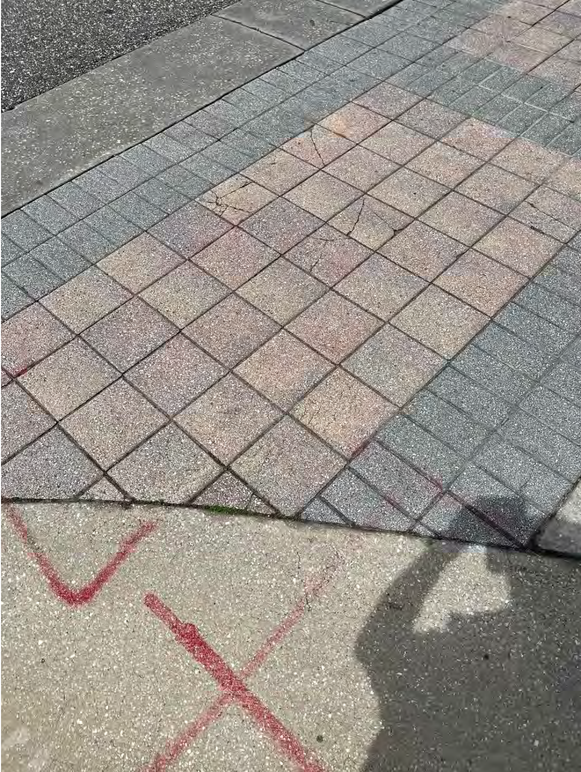
Photo 96 – Cracked Pavers
