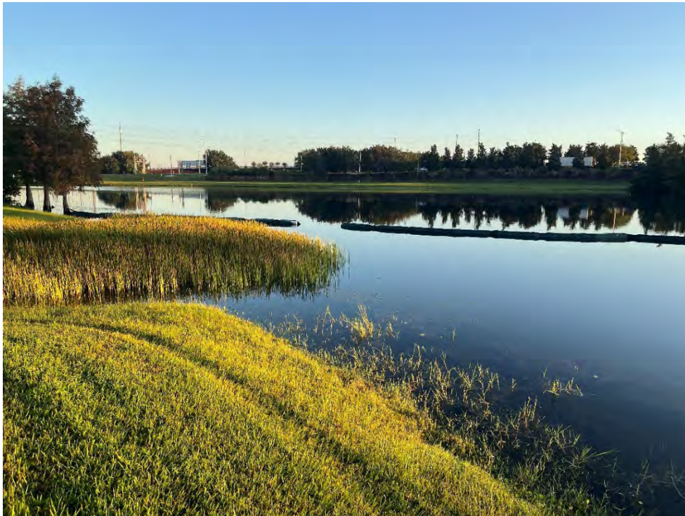
Photo 79 – Detached and Broken Floating Turbidity Barrier
