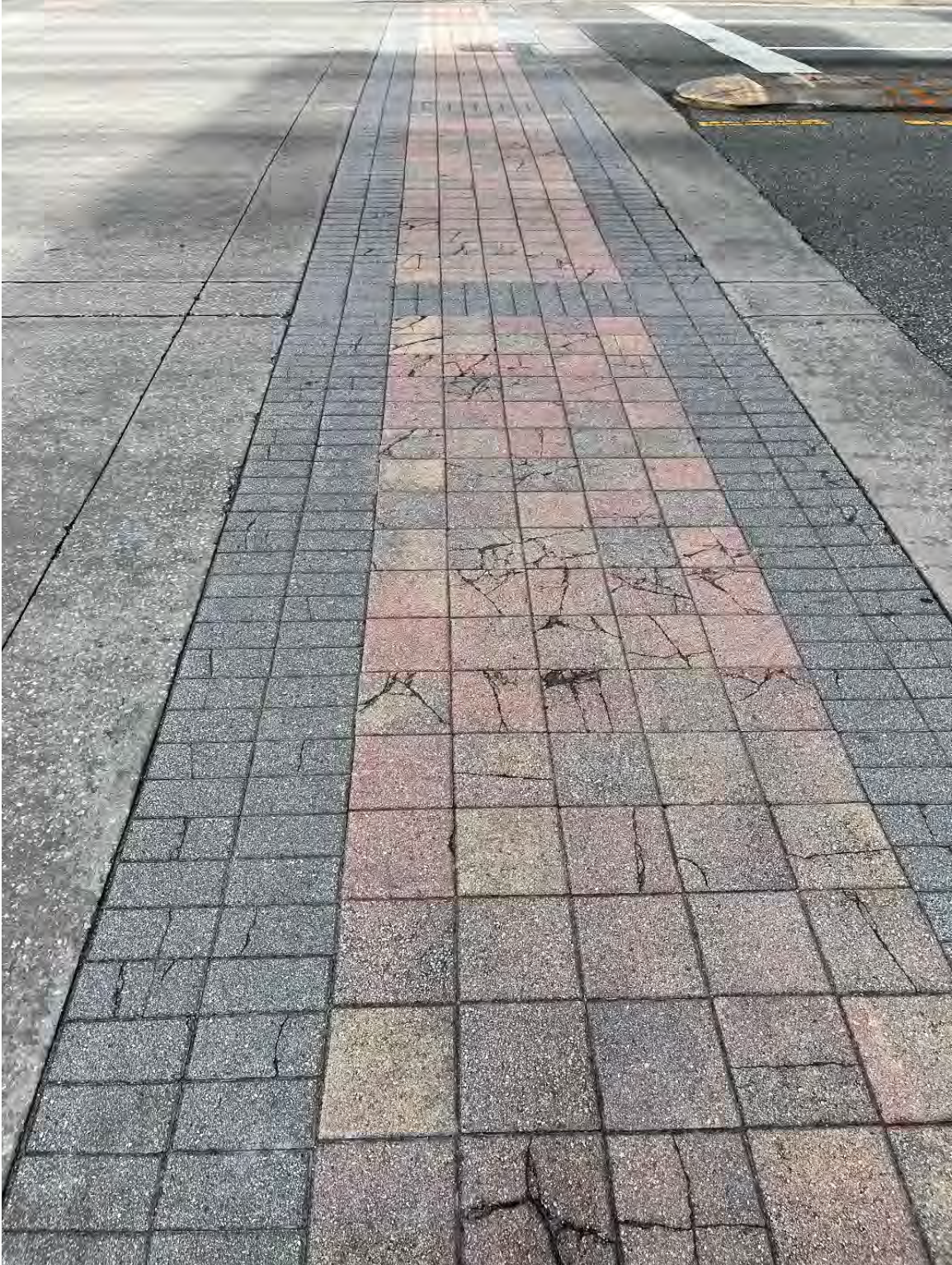
Photo 97 – Cracked Pavers
