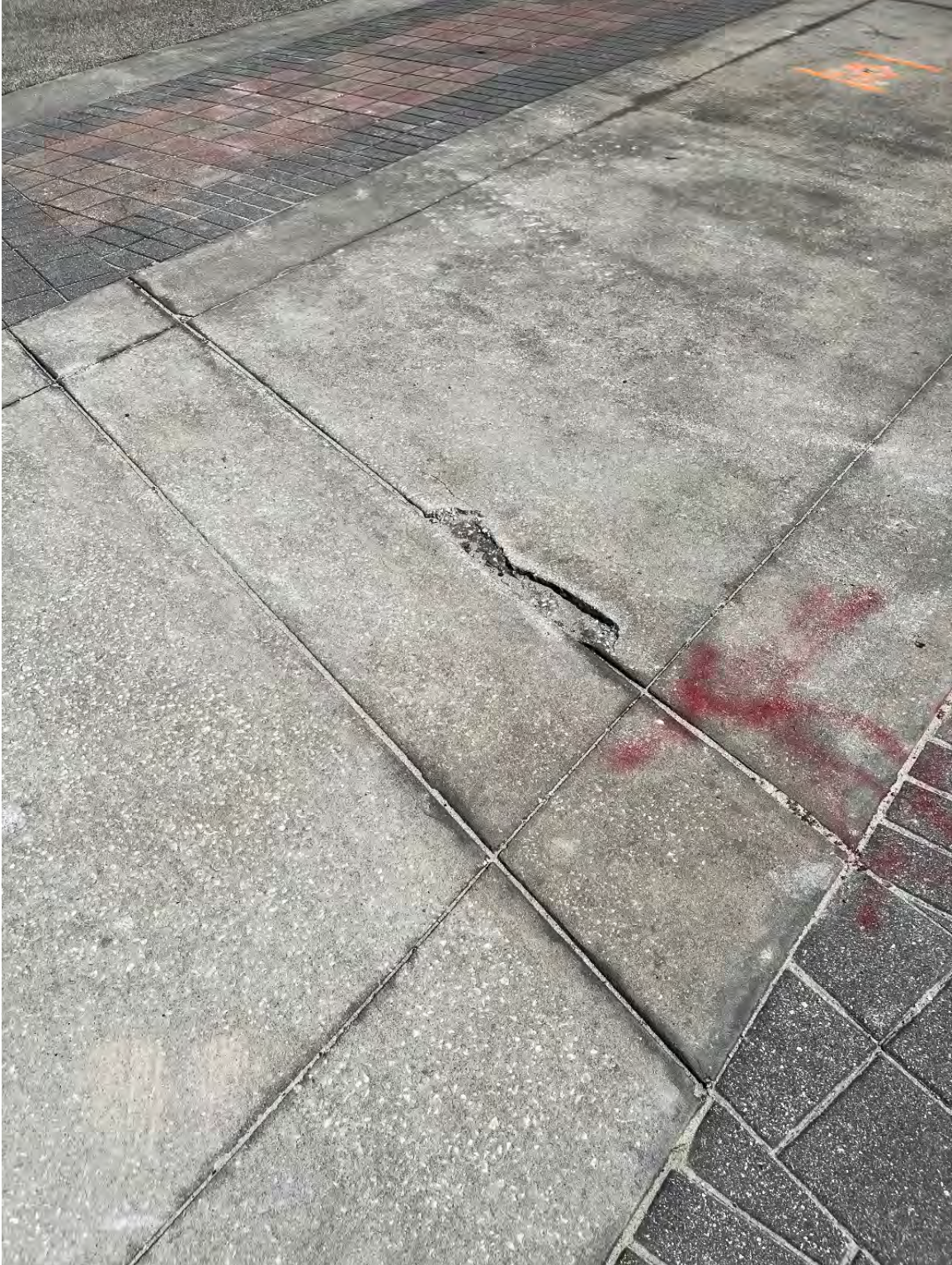
Photo 124 – Broken Concrete
