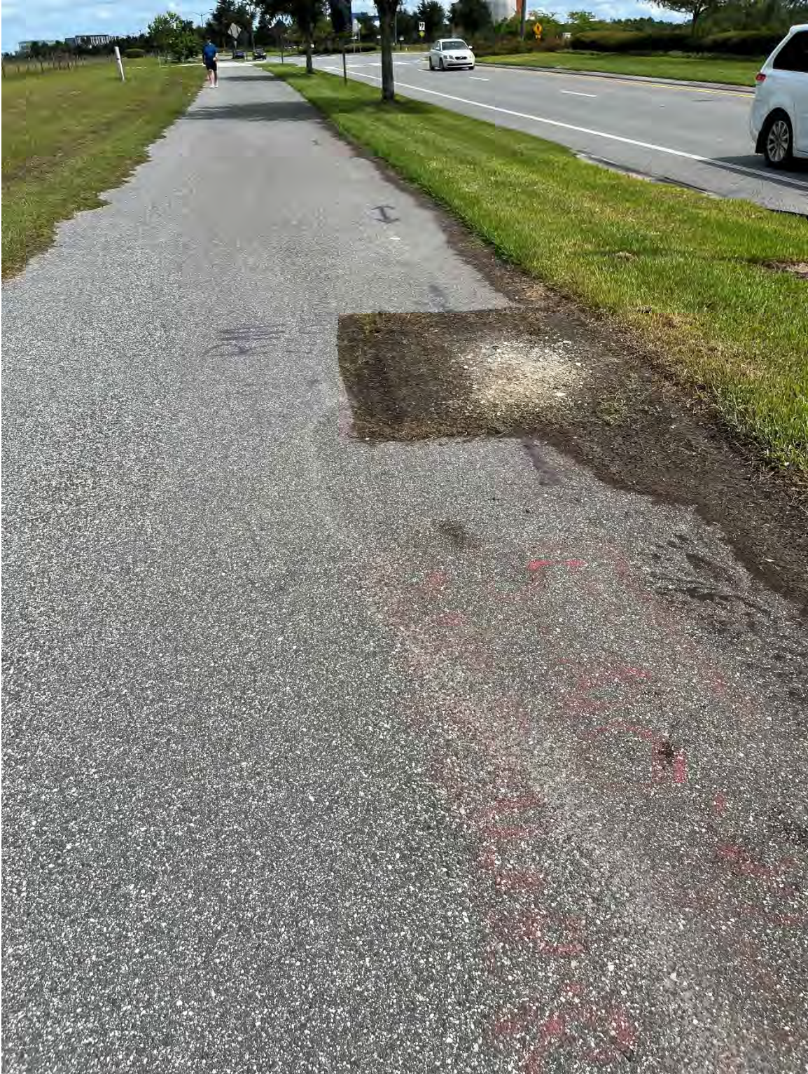
Photo 9 – Asphalt Cutout and Removed
