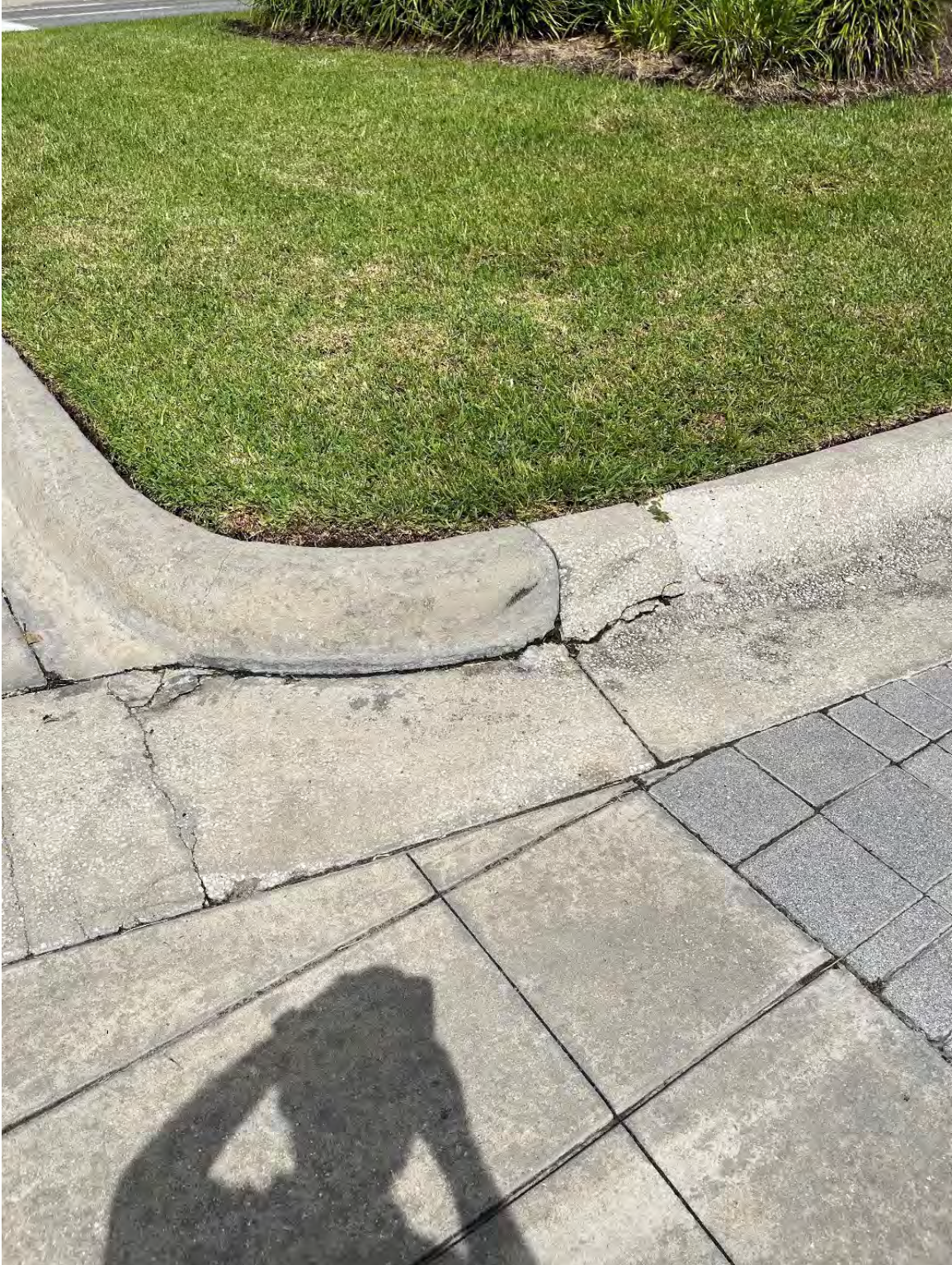
Photo 107 – Broken Curb
