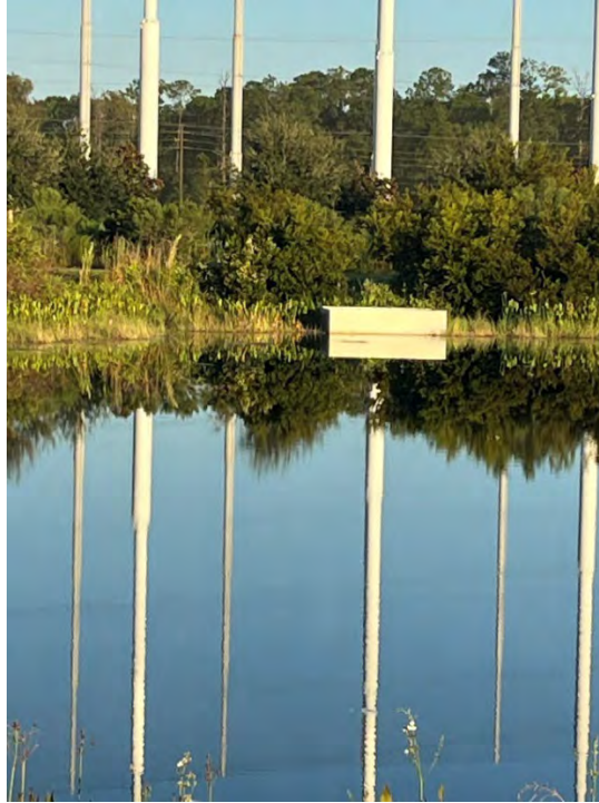
Photo 82 – Outfall Structure View from South Side of Pond Looking NW in Good Condition
