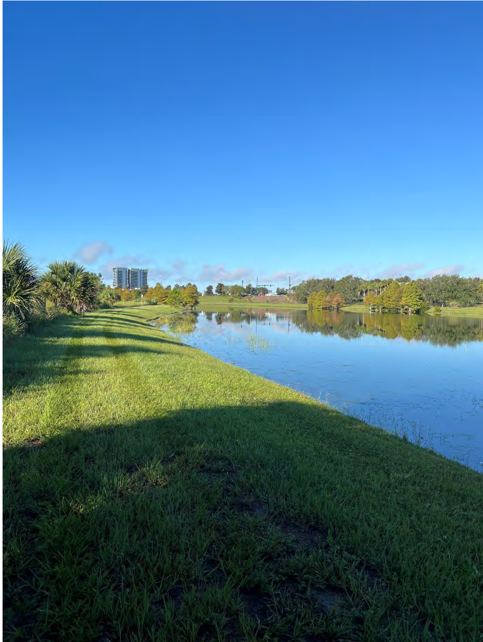
Photo 90 – South Berm Looking West in Good Condition
