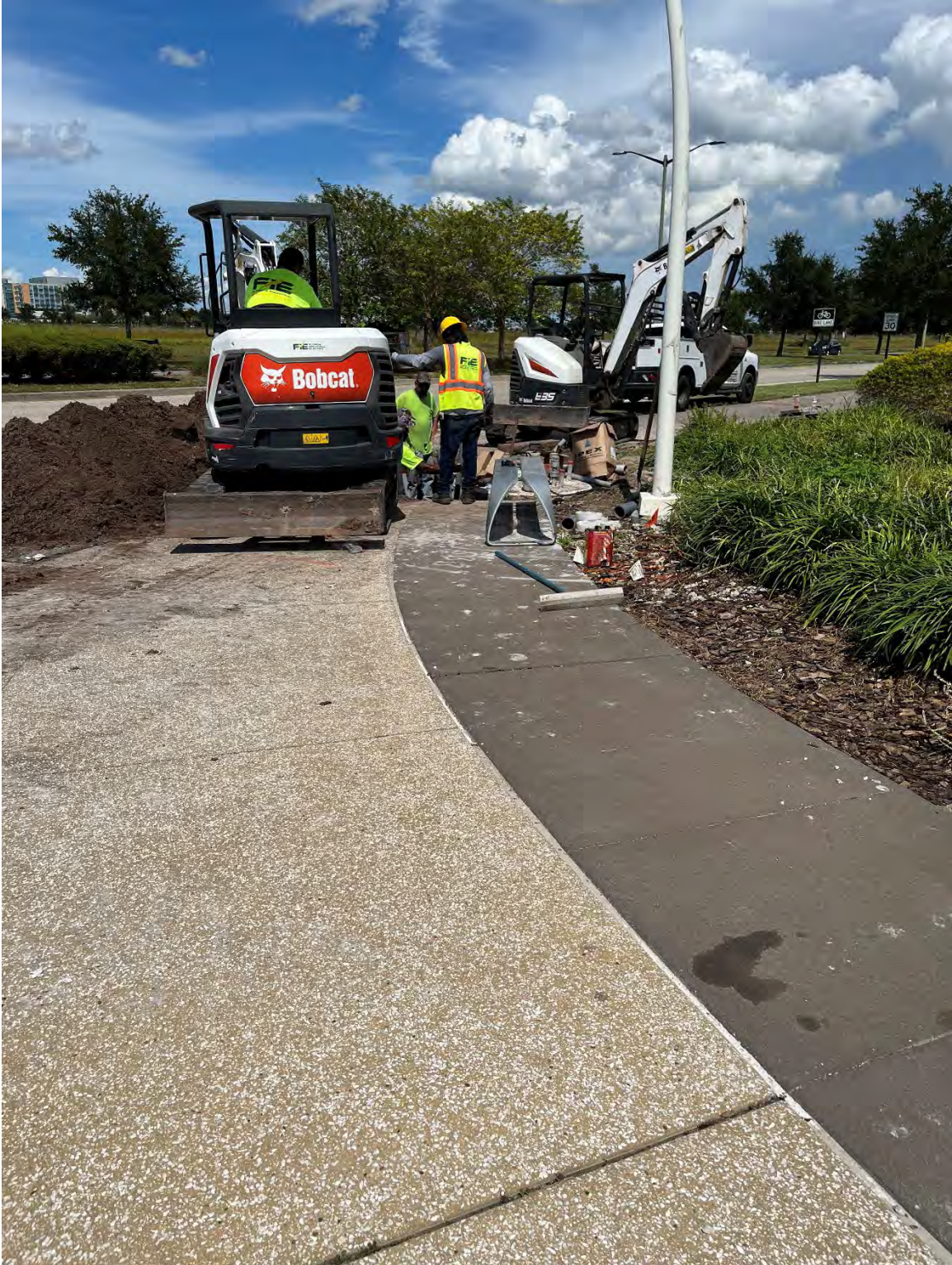
Photo 67 - Construction in Entrance at VA Hospital Intersection
