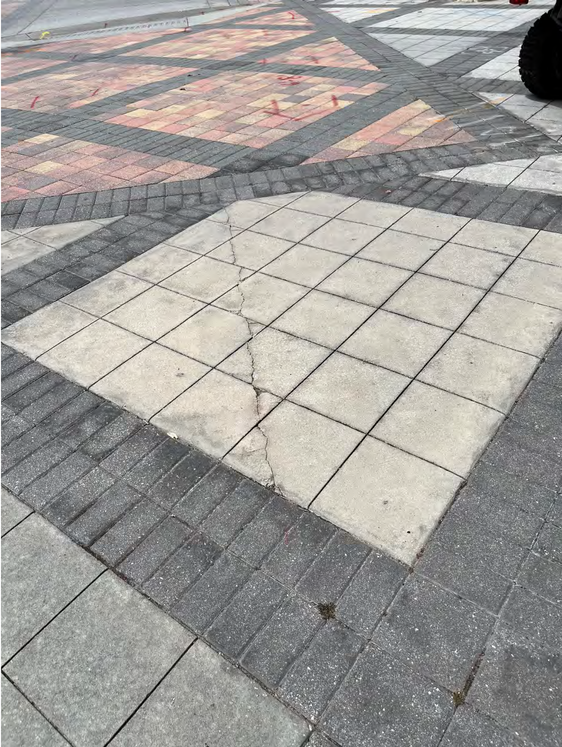
Photo 47 - Broken Pavers
