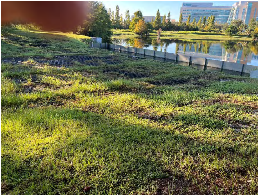
Photo 87 –Weir on NE Corner in Good Condition
