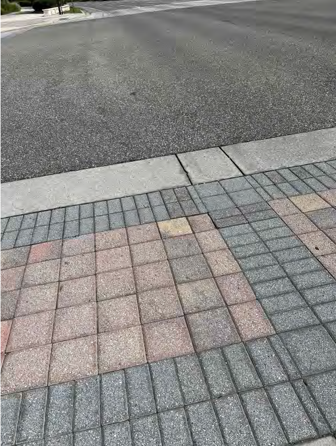
Photo 103 – Minor Settling
