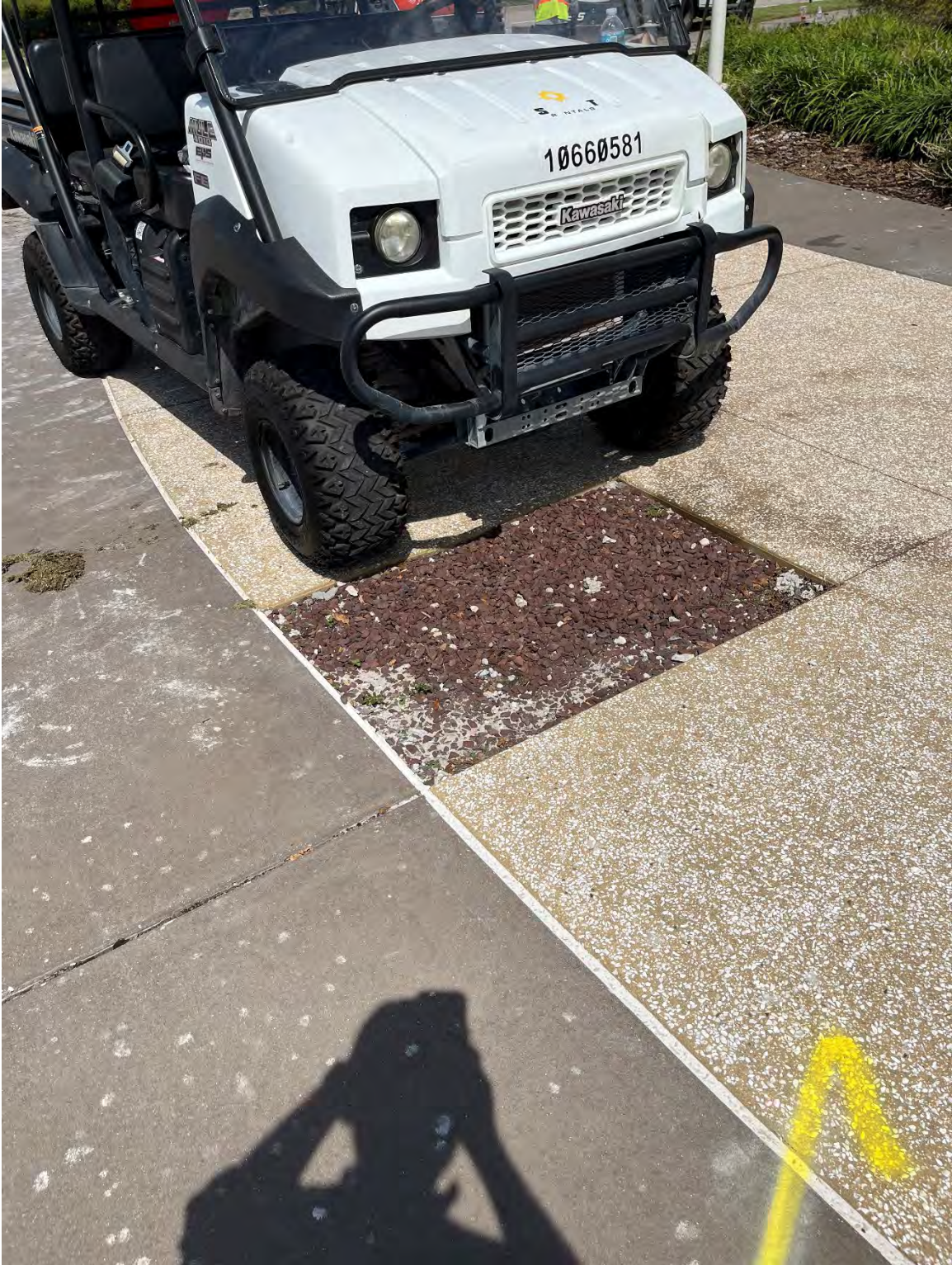
Photo 66 - Concrete Cutout - Construction at VA Hospital Intersection
