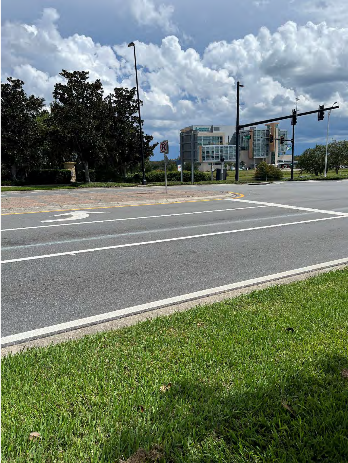
Photo 56 - Median Looking South onto SR 417
