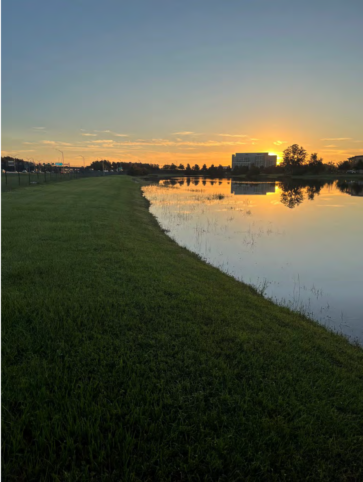
Photo 75 – Pond Berm Looking East in Good Condition
