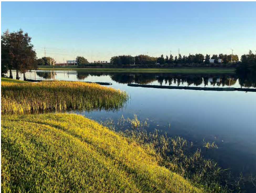
Photo 79 – Detached and Broken Floating Turbidity Barrier
