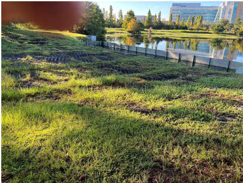
Photo 87 –Weir on NE Corner in Good Condition
