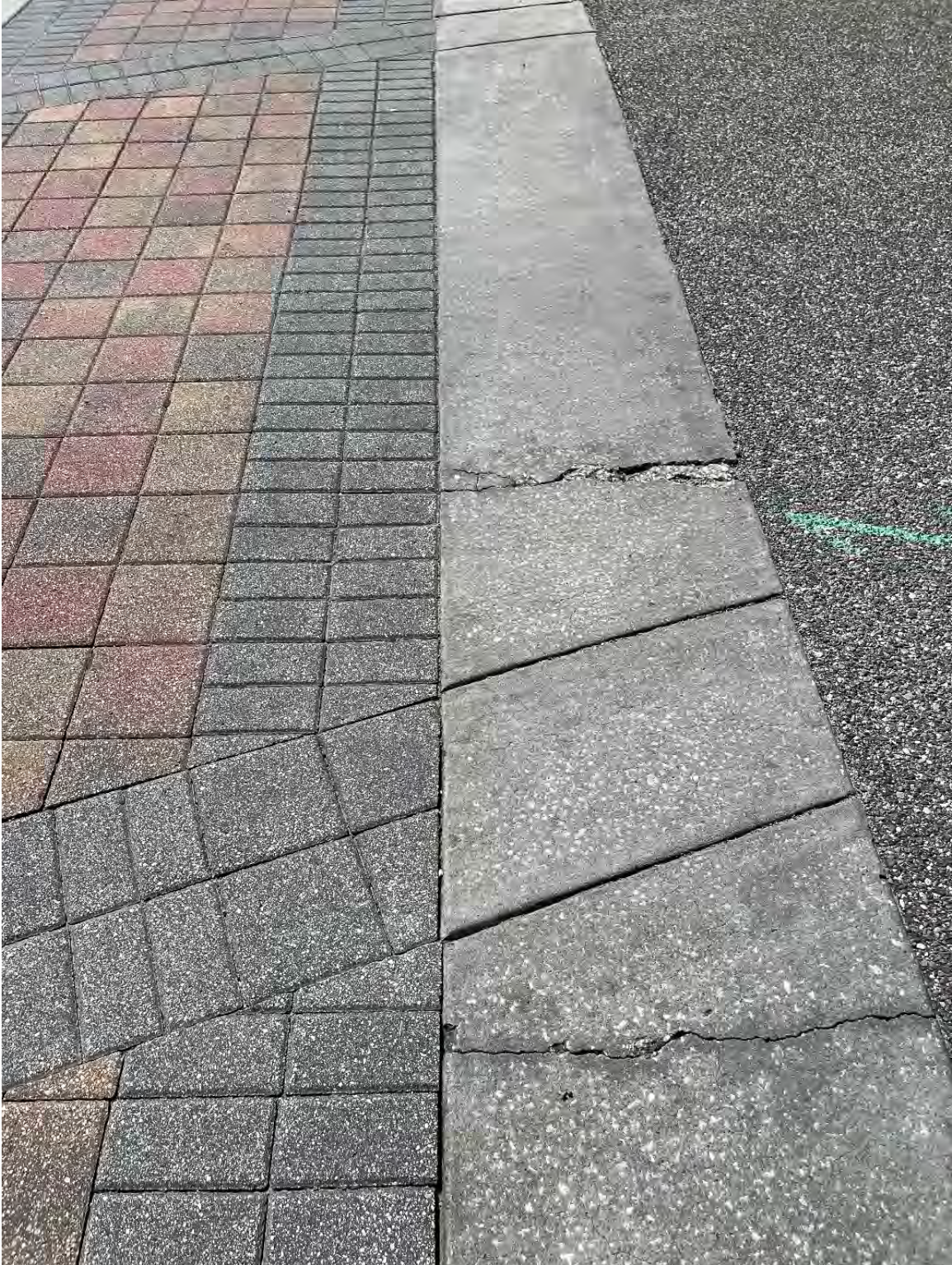
Photo 122 – Broken Concrete
