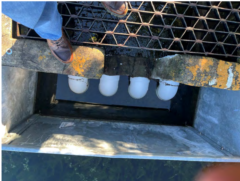
Photo 89 – Drawdown Pipe Inside of Outfall Structure
