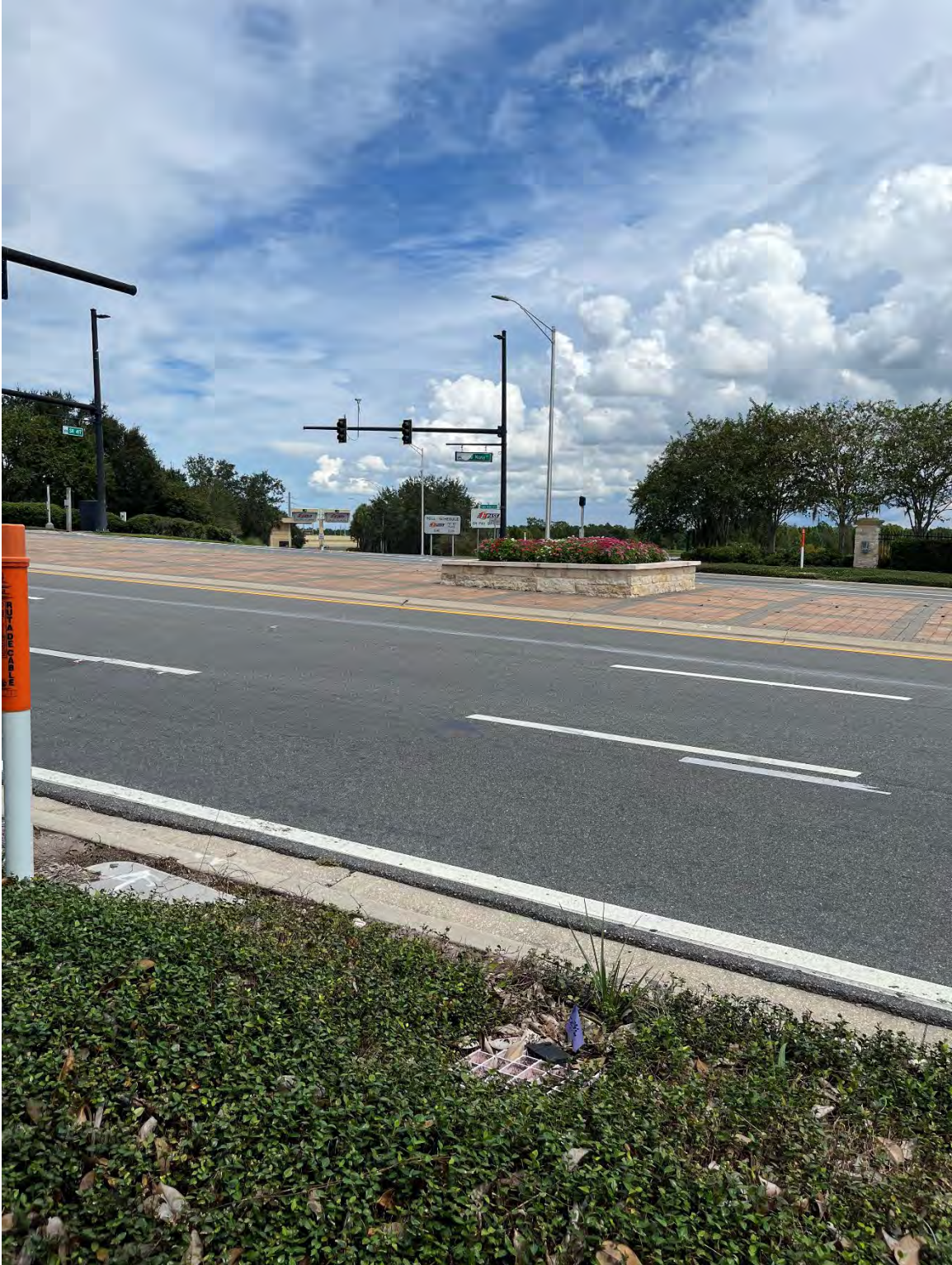
Photo 53 - East Entrance onto SR 417
