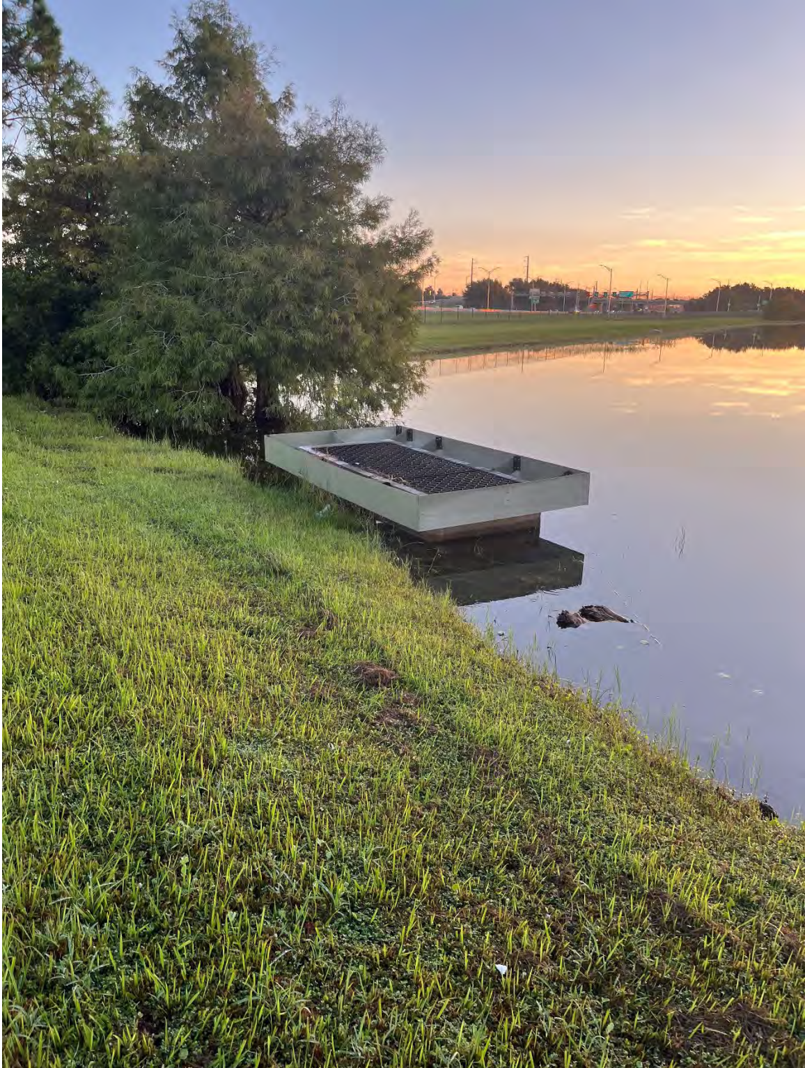
Photo 73 – Pond Outfall Structure in Good Condition
