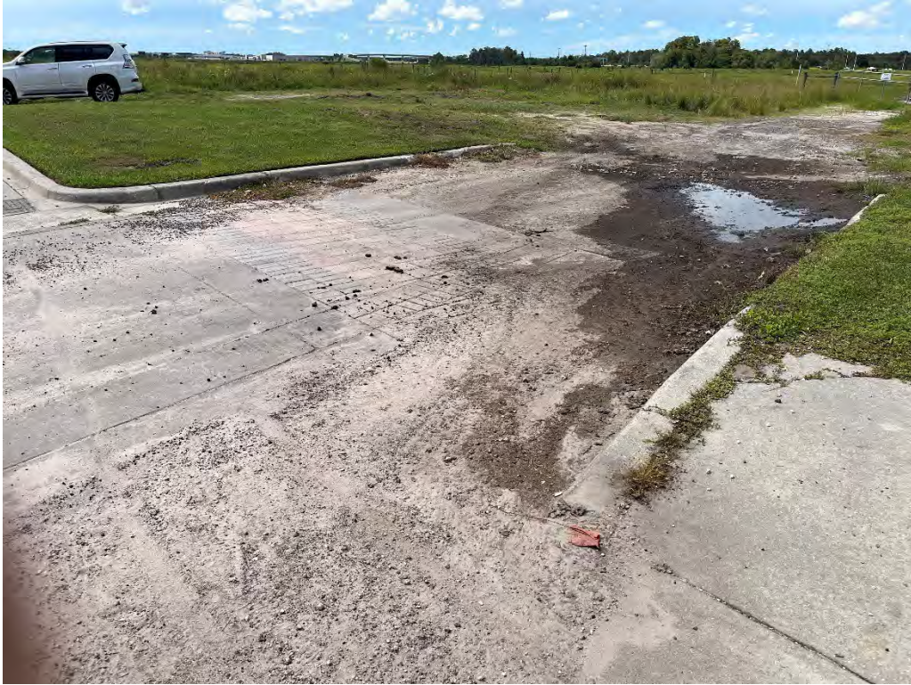
Photo 117 – Entrance to Construction Storage Area
