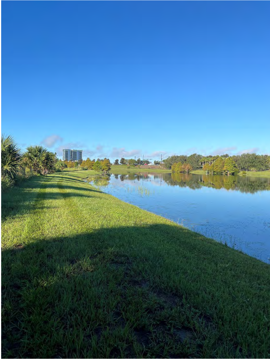
Photo 90 – South Berm Looking West in Good Condition
