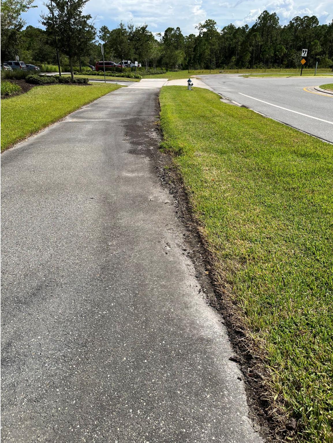
Photo 70 – Poor Drainage
