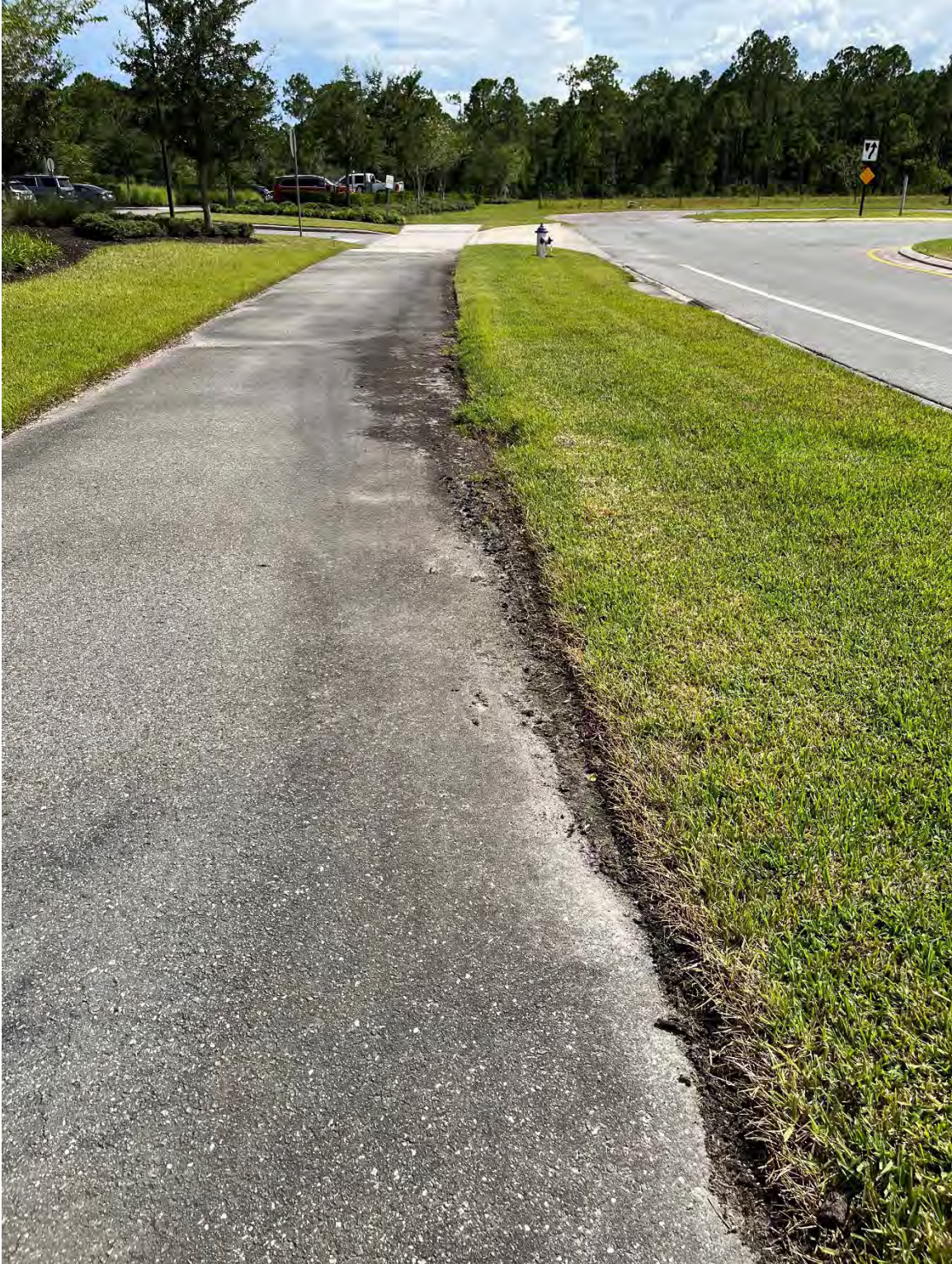
Photo 70 – Poor Drainage
