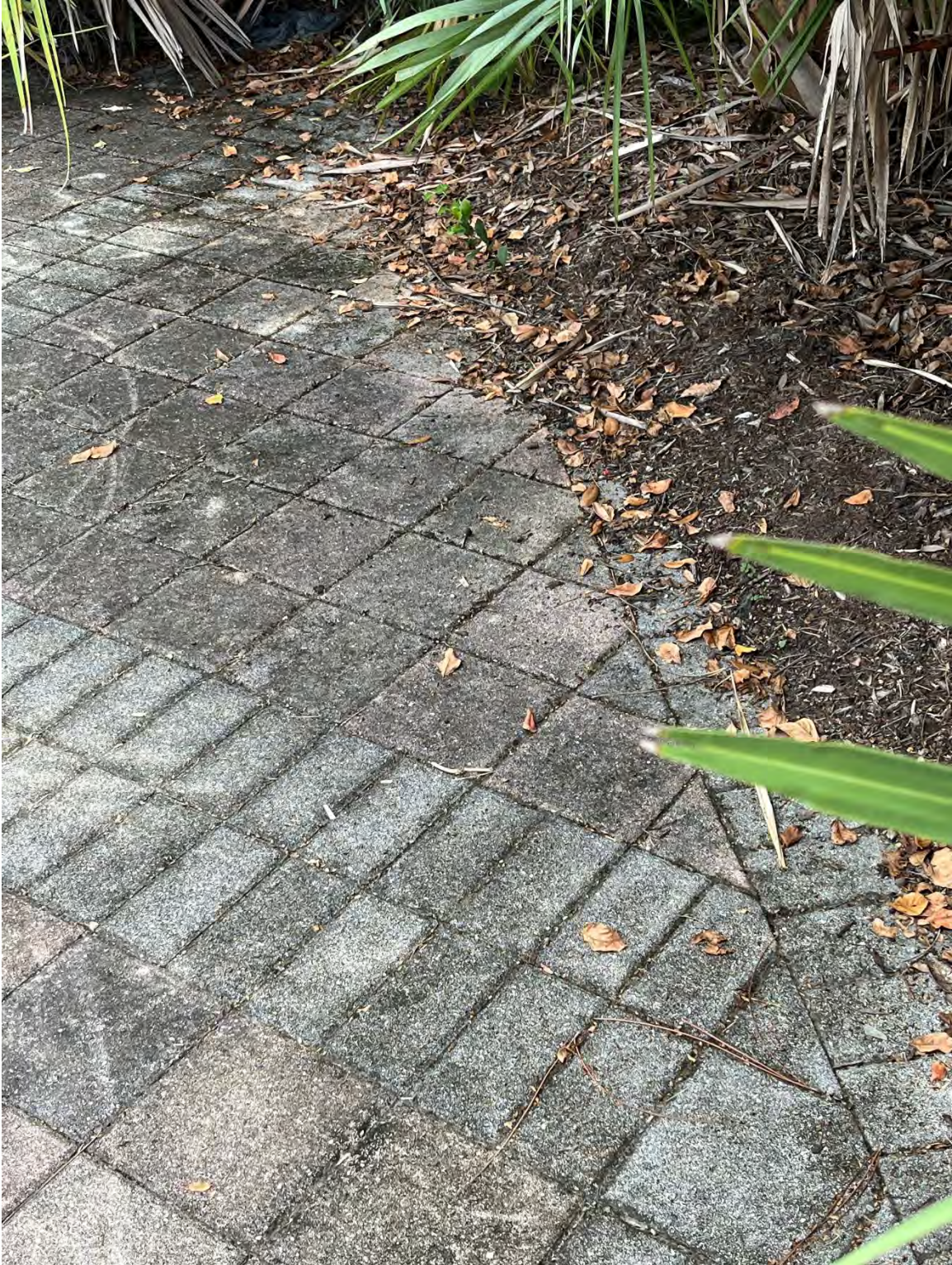
Photo 36 - Soil Covering Pavers
