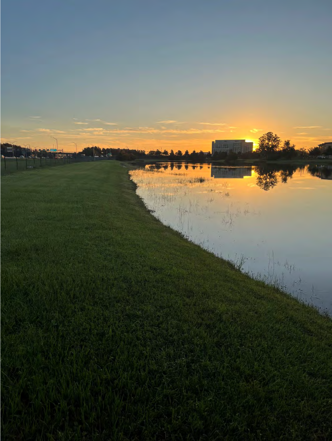
Photo 75 – Pond Berm Looking East in Good Condition
