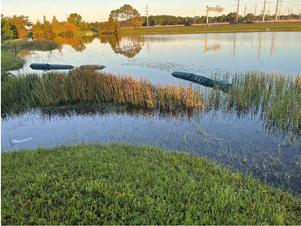
Photo 80 – Broken Floating Turbidity Barrier
