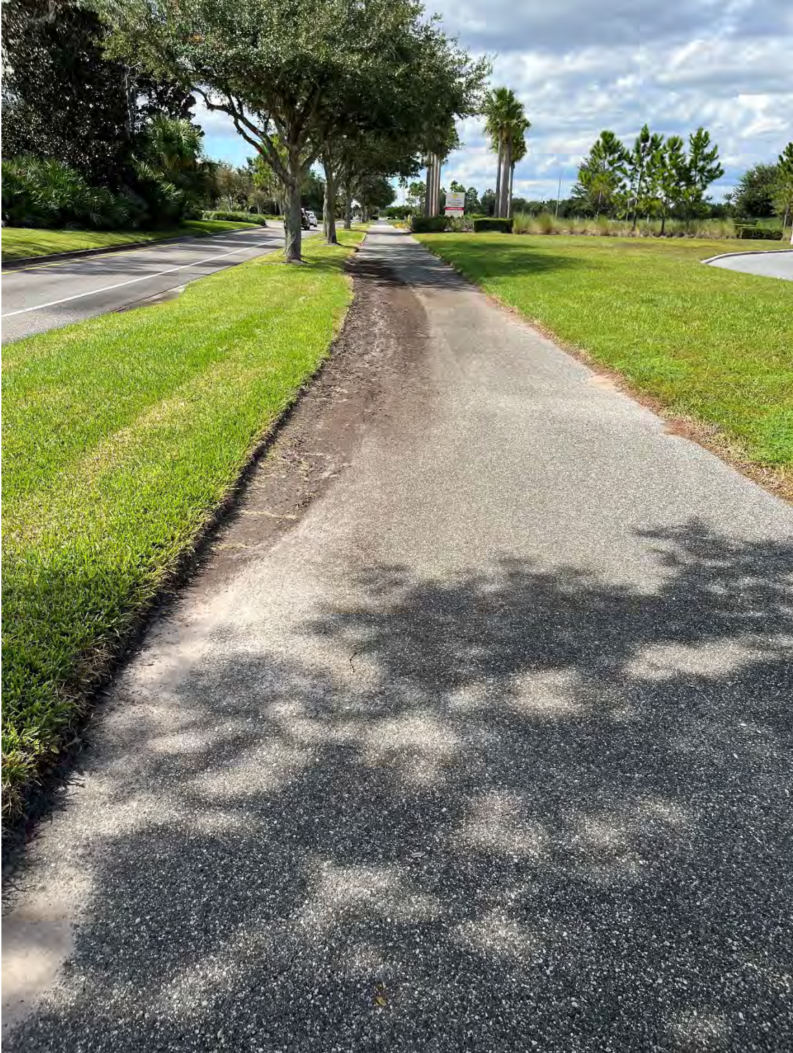
Photo 71 – Poor Drainage
