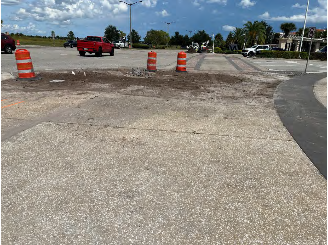
Photo 68 - Construction in All Quads at VA Hospital Intersection
