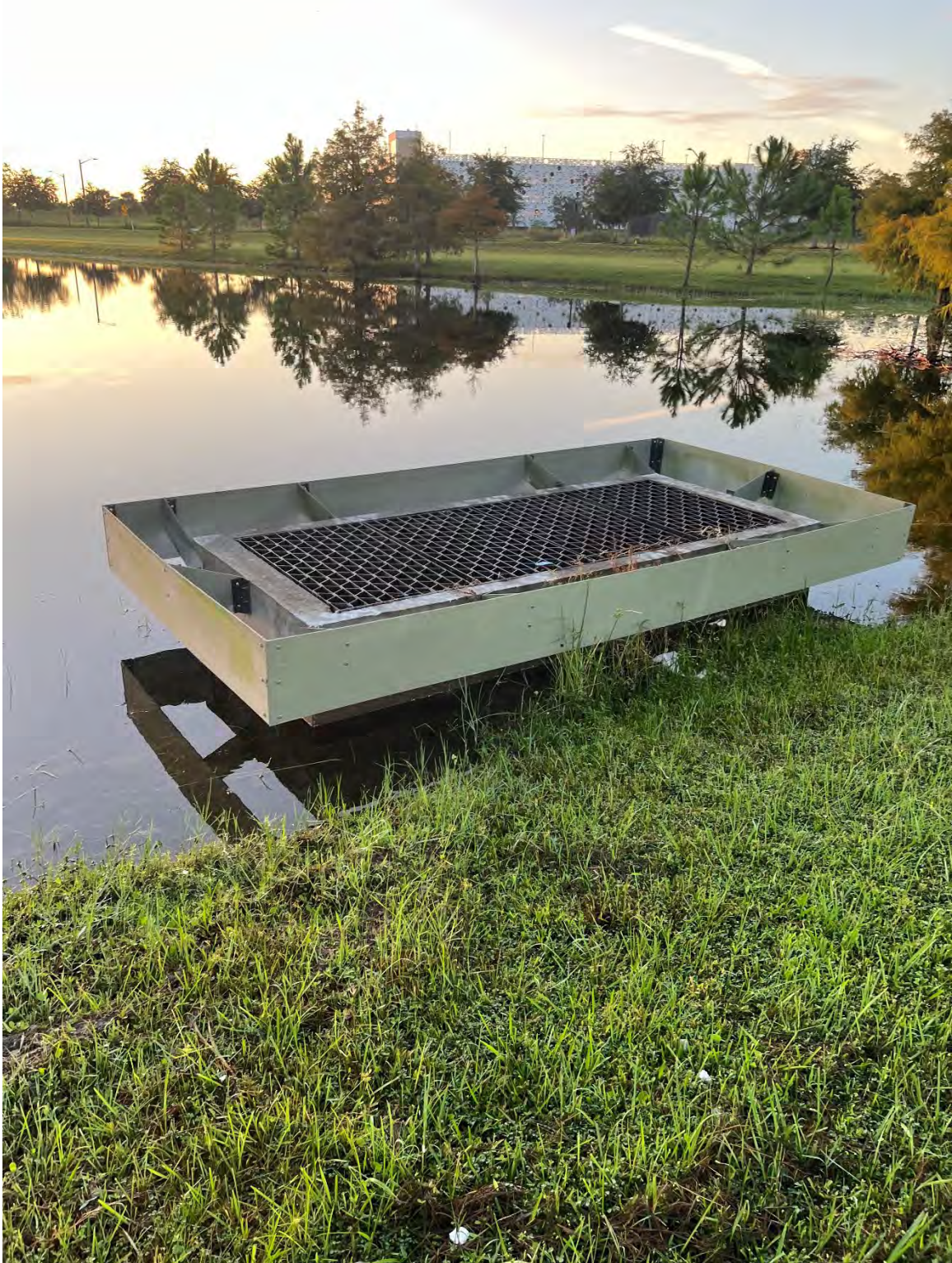
Photo 74 – Pond Outfall Structure in Good Condition
