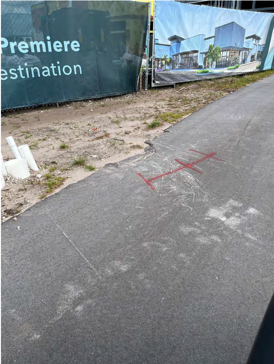
Photo 5 – Asphalt Damage (construction ongoing)
