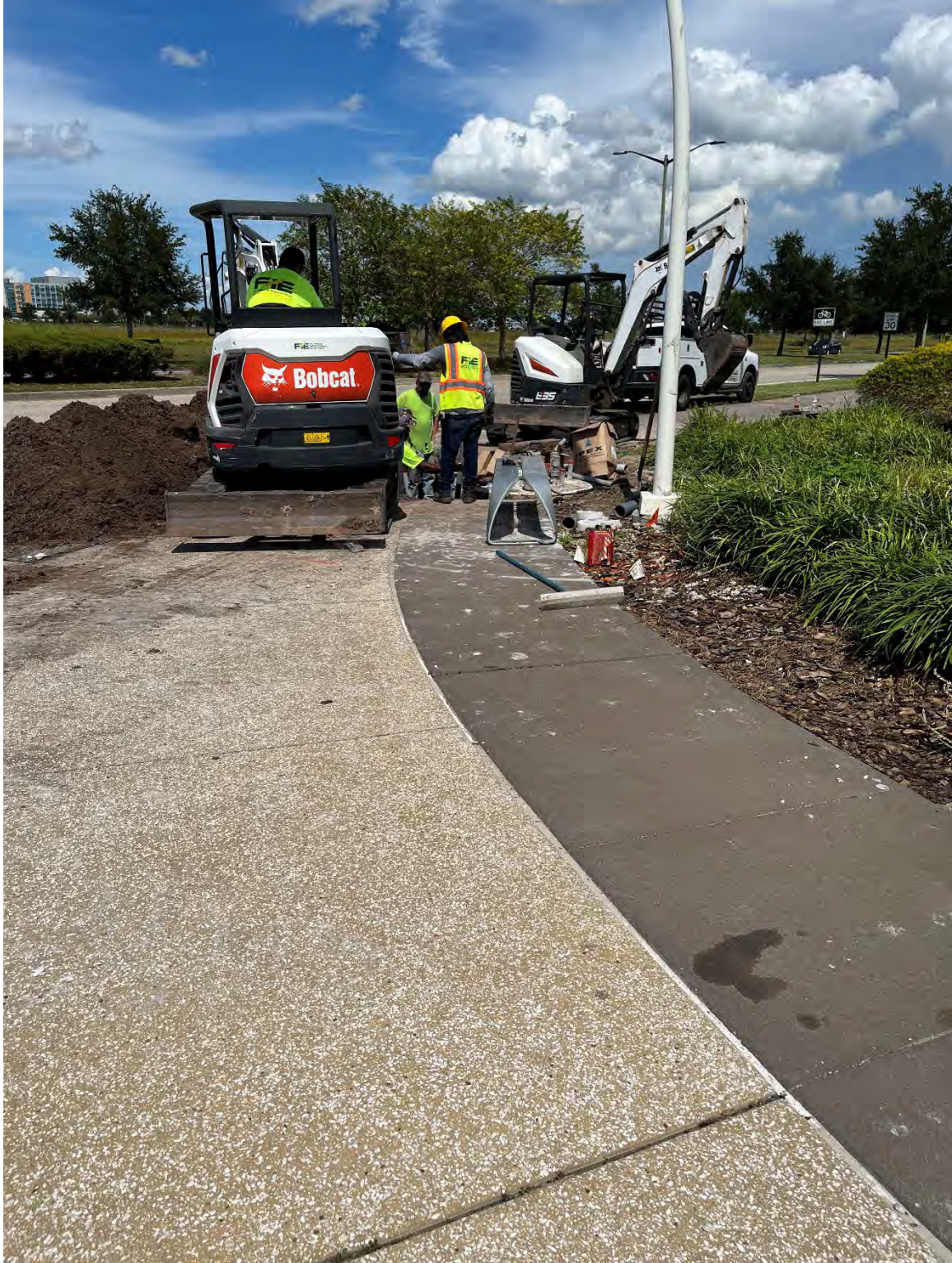
Photo 67 - Construction in Entrance at VA Hospital Intersection
