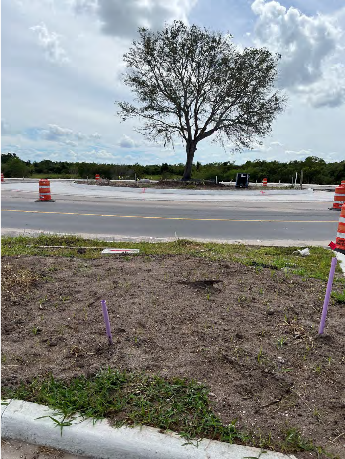
Photo 4 – Roundabout Under Construction
