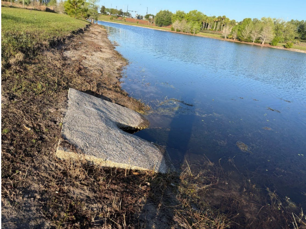
Photo 70.1 – Stormwater Inflow in Good Condition (New Photo – 2026 Assessment)
