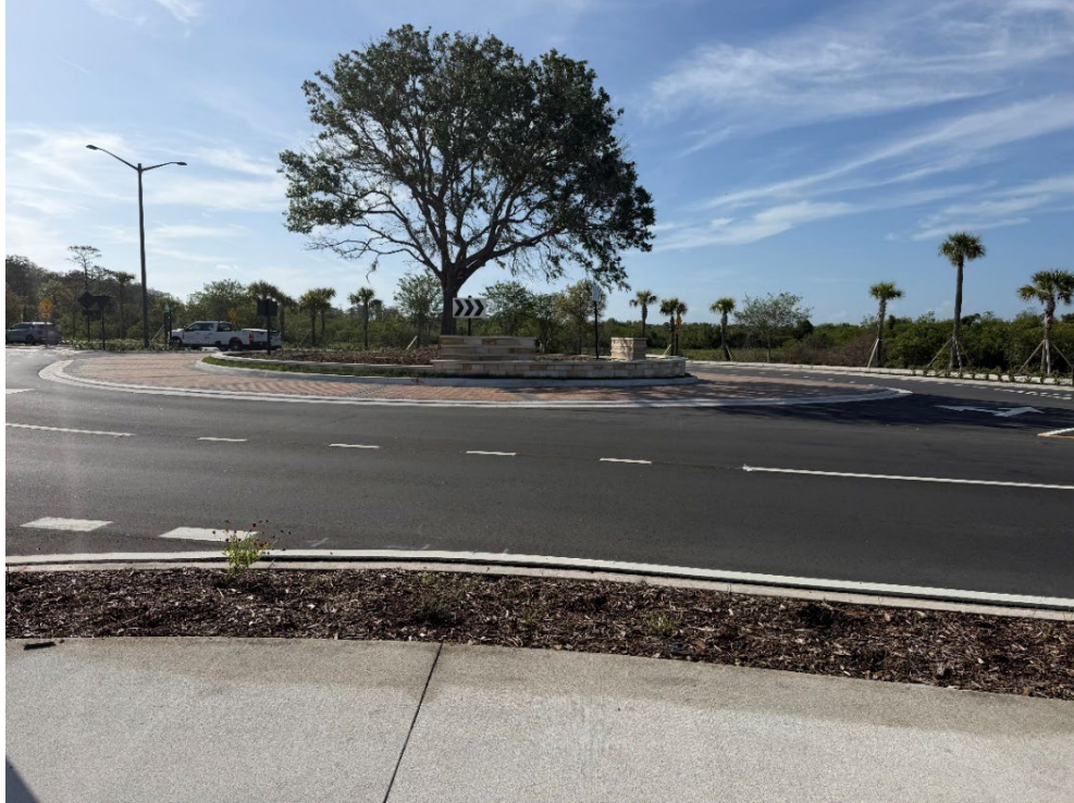
Photo 3 – Roundabout Under Construction (Roundabout Constructed) (Refer to Prior Photo 4- 2025 Assessment)
