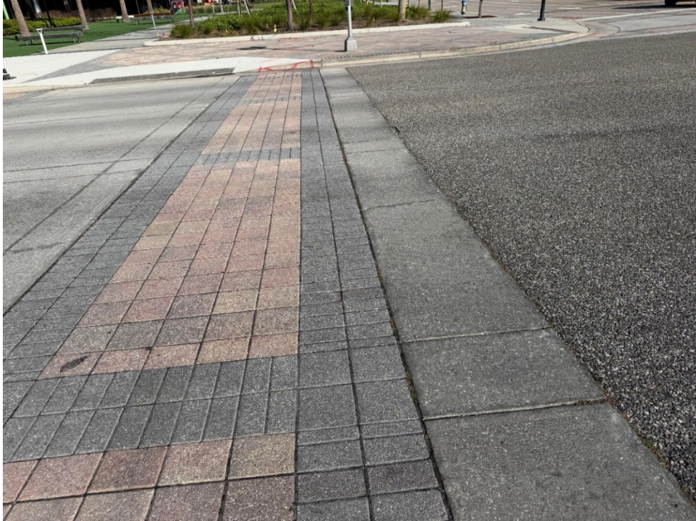
Photo 77 – Cracked Pavers, Minor Settling (No Observed Changes) (Refer to Prior Photo 101 - 2025 Assessment)
