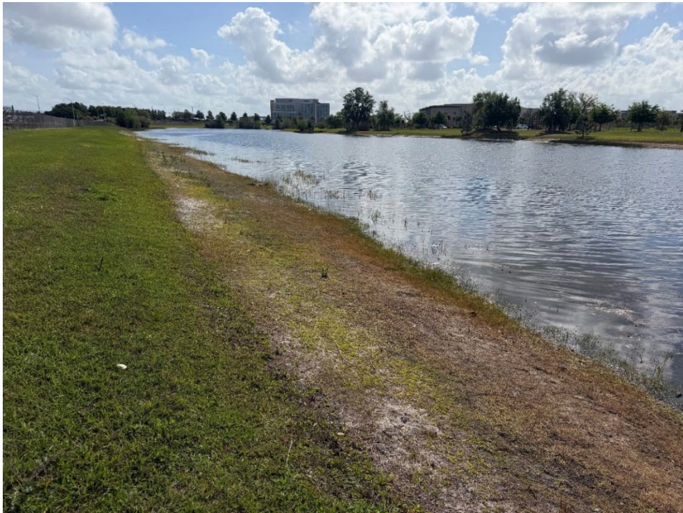
Photo 57 – Pond Berm Facing East in Good Condition (No Observed Changes) (Refer to Prior Photo 75- 2025 Assessment)
