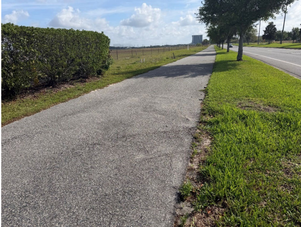
Photo 8 – Raveling Asphalt with Depression and Base Failure (No Observed Changes) (Refer to Prior Photo 11- 2025 Assessment)
