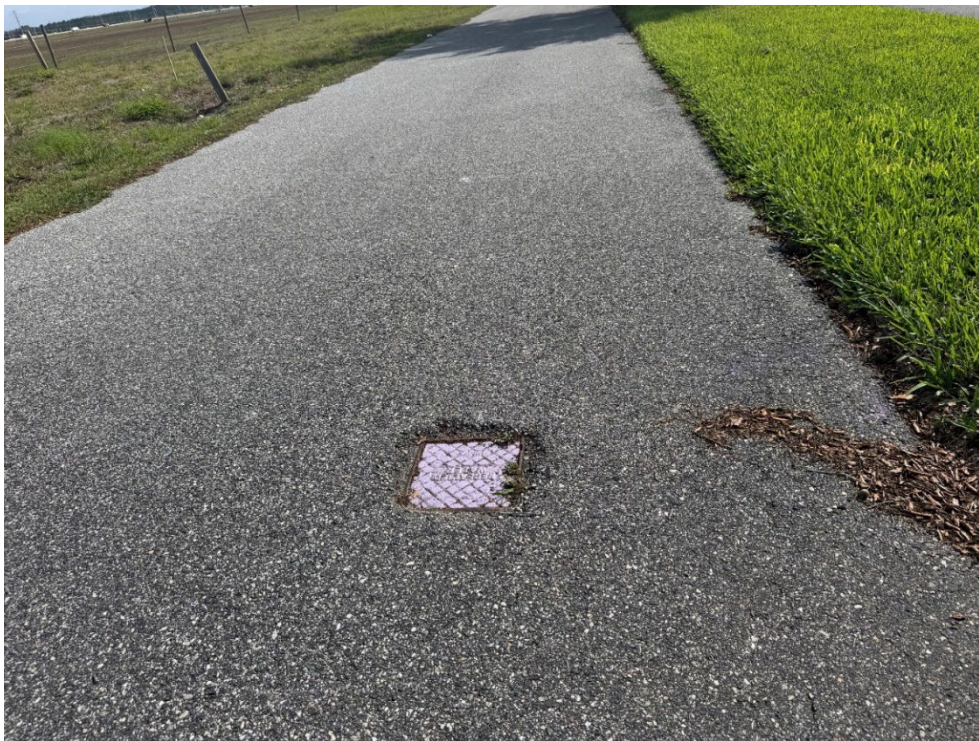
Photo 9 – Sunken Reclaim Water Meter (No Observed Changes) (Refer to Prior Photo 12- 2025 Assessment)
