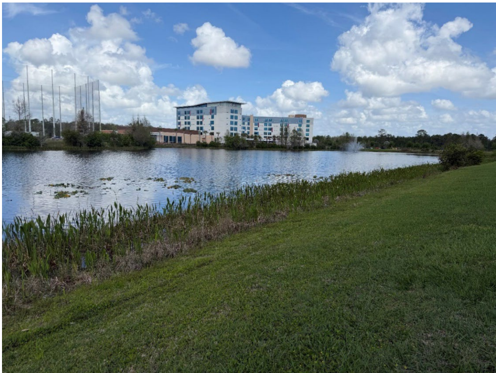
Photo 61.1 – Vegetation in Pond and Pond Berm in Good Condition (New Photo – 2026 Assessment)
