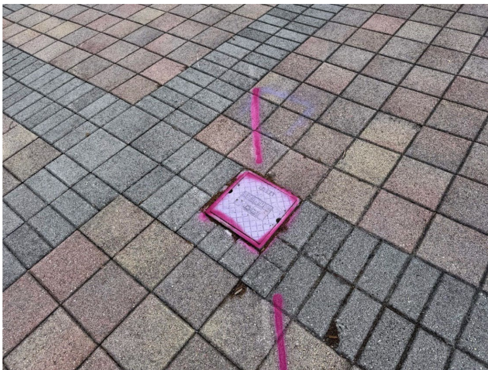
Photo 35 – Raised Reclaim Meter (Approximately ½ -inch) (No Observed Changes) (Refer to Prior Photo 42- 2025 Assessment)
