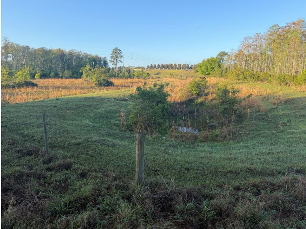
Photo 63 – Overgrown Inflow Ditch from Apartment Access Road into Pond (No Observed Changes) (Refer to Prior Photo 83- 2025 Assessment)
