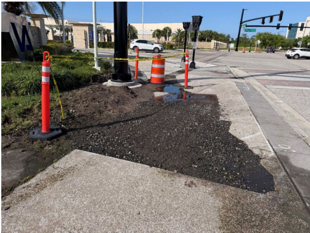
Photo 52 – Concrete Cut – Construction at VA Hospital Intersection (Construction More Extensive Than Previous Year) (Refer to Prior Photo 66 - 2025 Assessment)
