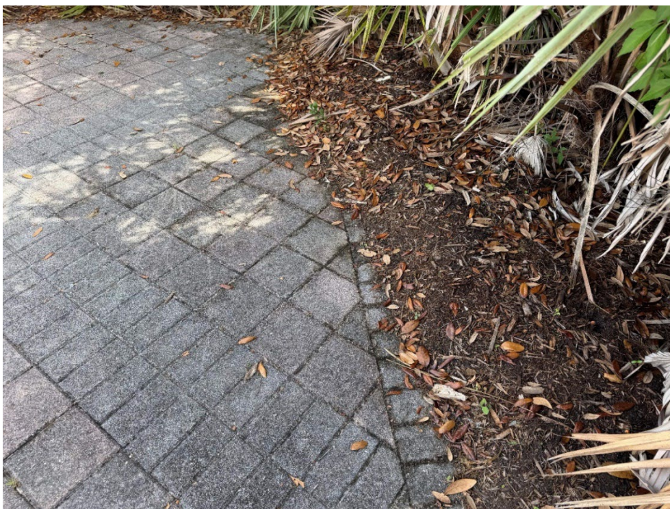
Photo 29 – Soil Covering Pavers (No Observed Changes) (Refer to Prior Photo 36- 2025 Assessment)
