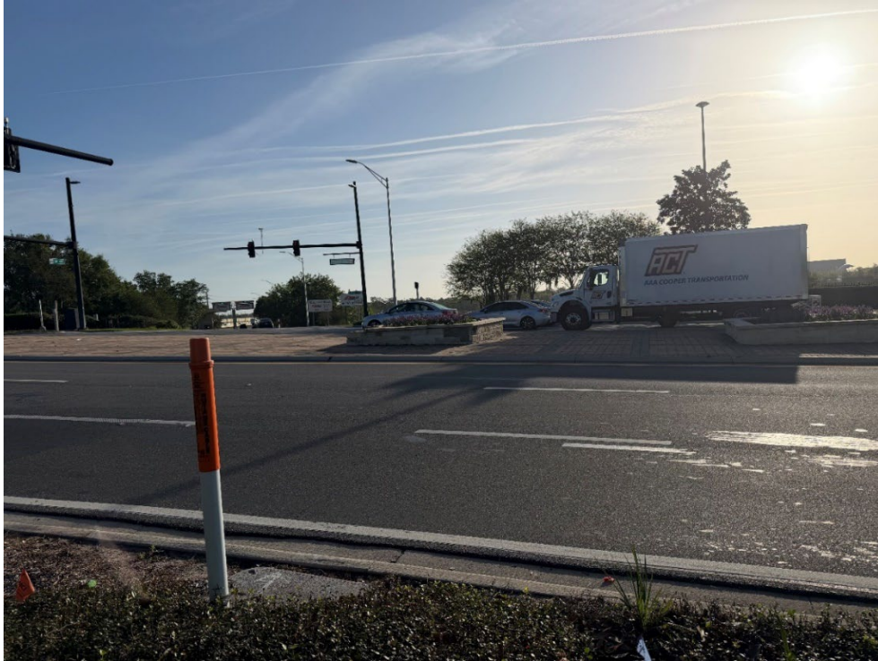
Photo 43 – East Entrance on to SR 417 (No Observed Changes) (Refer to Prior Photo 53- 2025 Assessment)
