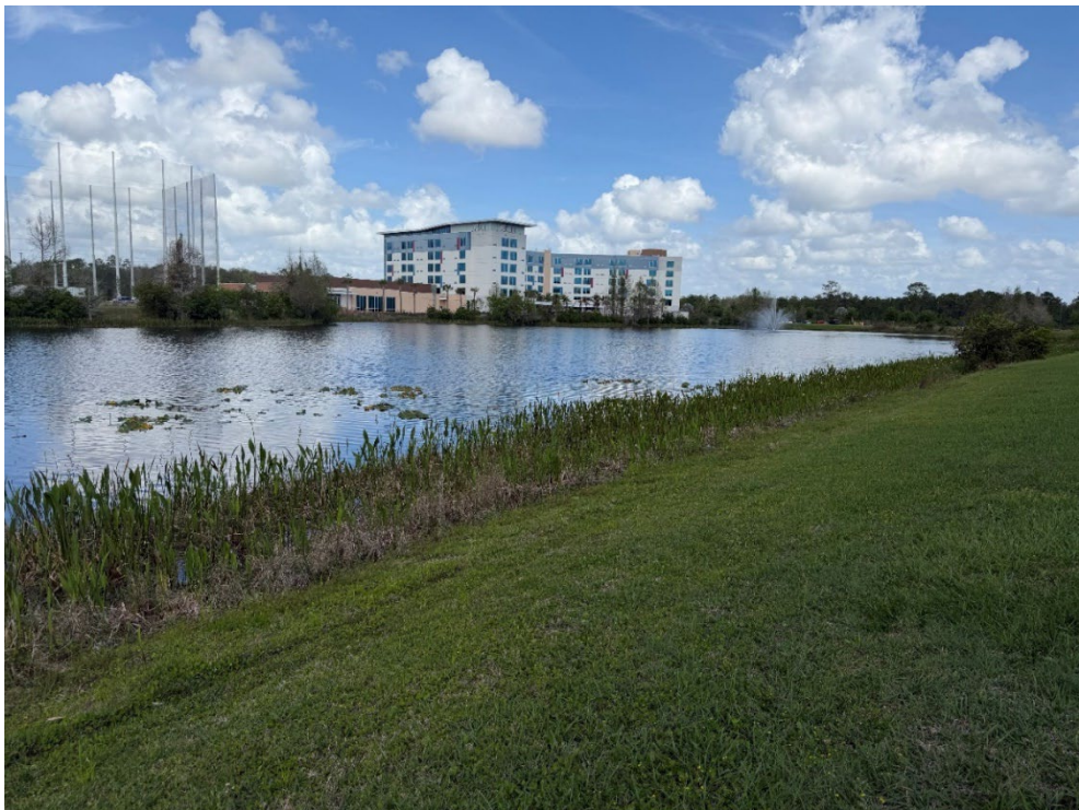
Photo 61.1 – Vegetation in Pond and Pond Berm in Good Condition (New Photo – 2026 Assessment)
