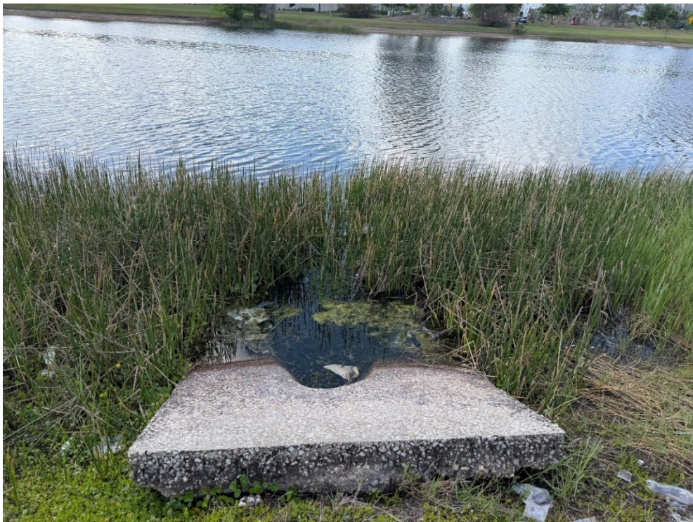
Photo 57.2 – Discharge Into Pond (New Photo – 2026 Assessment)
