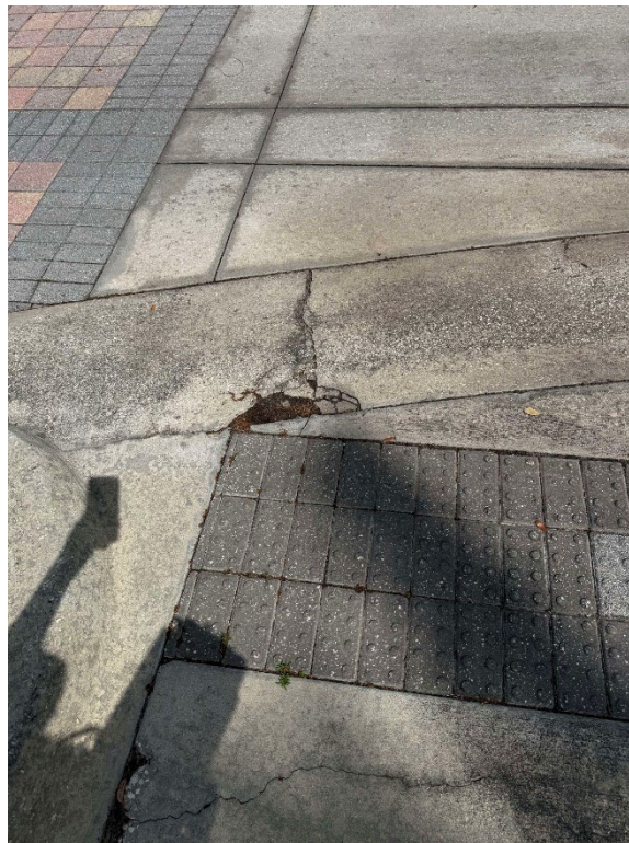
Photo 23 – Cracked Concrete in East Median (No Observed Changes) (Refer to Prior Photo 30- 2025 Assessment)
