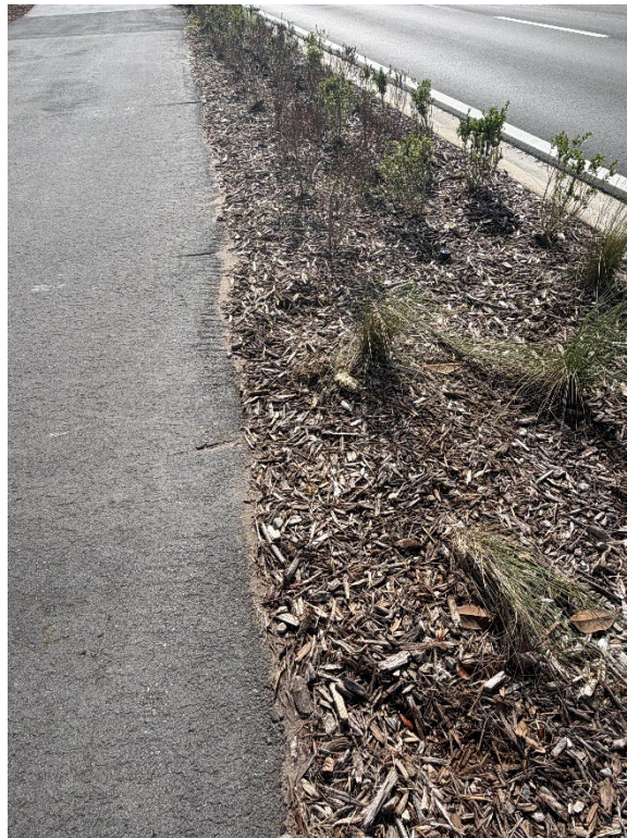
Photo 5.1 – Damaged Asphalt (New Photo – 2026 Assessment)
