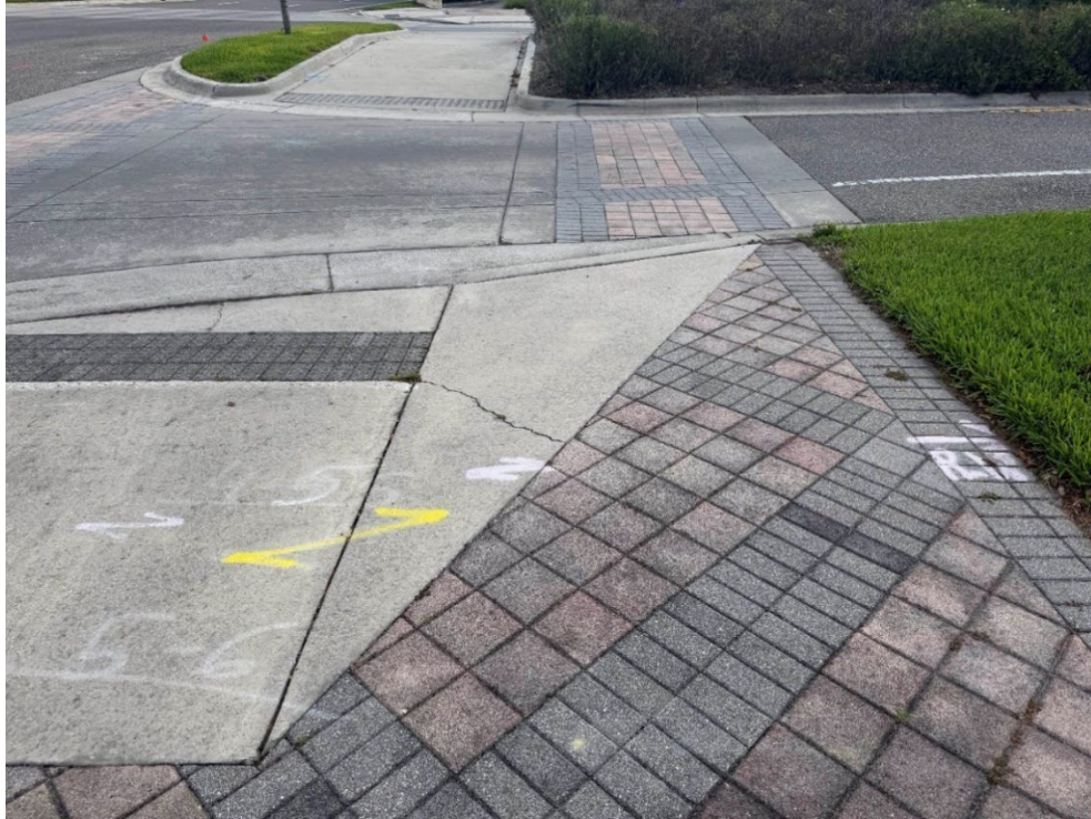
Photo 14 – Surficial Concrete Cracks in Handicap Ramp (No Observed Changes) (Refer to Prior Photo 17 - 2025 Assessment)
