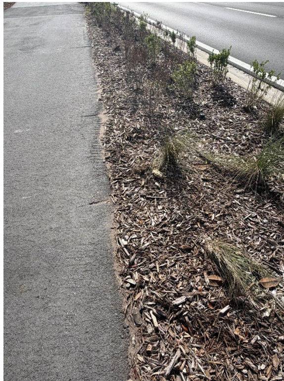
Photo 5.1 – Damaged Asphalt (New Photo – 2026 Assessment)
