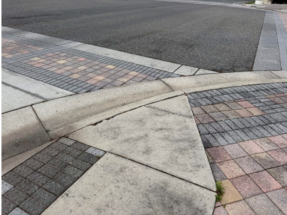
Photo 24 – Surficial Concrete Cracks in Handicap Ramp (No Observed Changes) (Refer to Prior Photo 31- 2025 Assessment)
