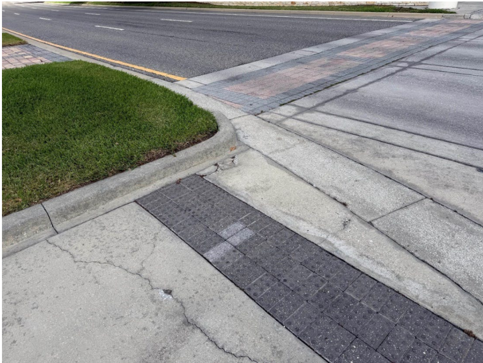
Photo 17 – Surficial Concrete Cracks in Handicap Ramp (No Observed Changes) (Refer to Prior Photo 21- 2025 Assessment)
