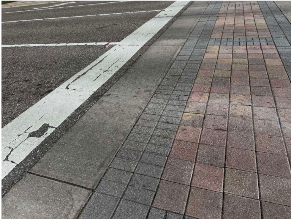
Photo 83 – Cracked Pavers, Some Settling (No Observed Changes) (Refer to Prior Photo 110 - 2025 Assessment)
