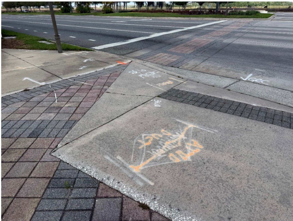
Photo 11 – Surficial Concrete Cracks in Handicap Ramp (No Observed Changes) (Refer to Prior Photo 14- 2025 Assessment)
