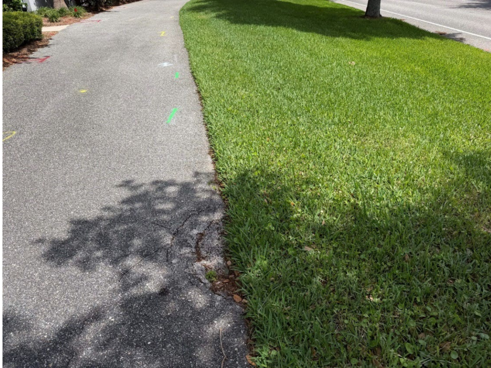
Photo 36 – Raveling Asphalt and Base Failure (No Observed Changes) (Refer to Prior Photo 43- 2025 Assessment)
