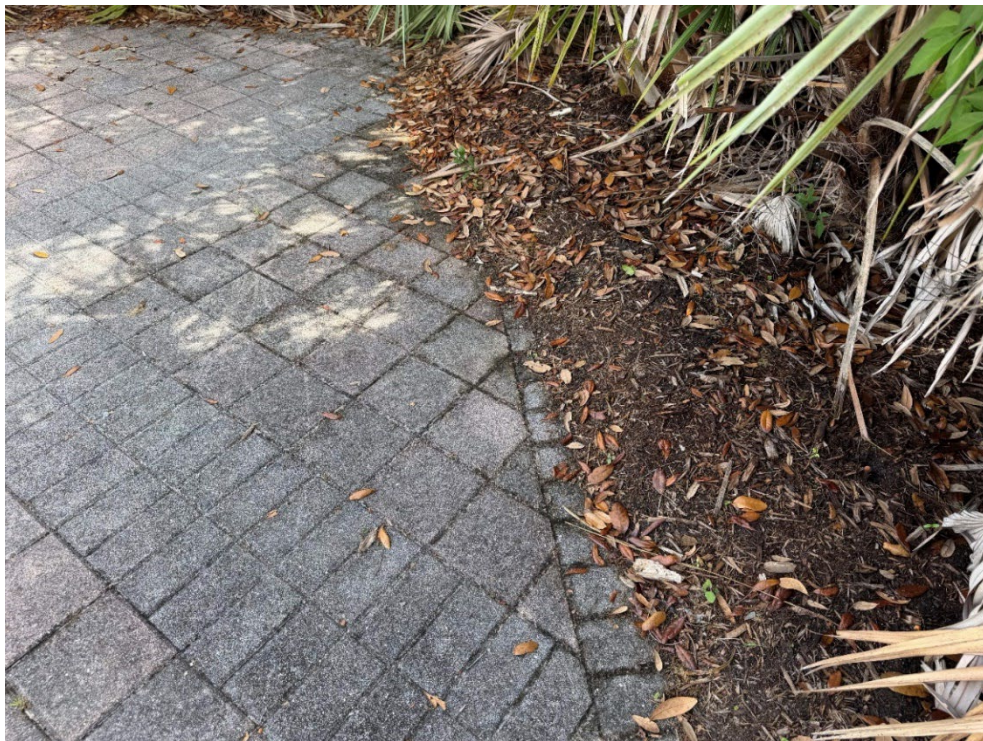
Photo 29 – Soil Covering Pavers (No Observed Changes) (Refer to Prior Photo 36- 2025 Assessment)
