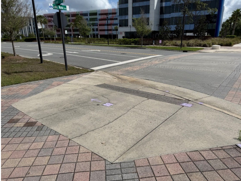
Photo 16 – Surficial Concrete Cracks in Handicap Ramp (No Observed Changes) (Refer to Prior Photo 20- 2025 Assessment)
