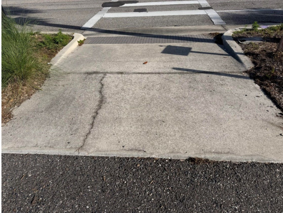
Photo 51 – Surficial Concrete Cracks in Handicap Ramp (No Observed Changes) (Refer to Prior Photo 63 - 2025 Assessment)
