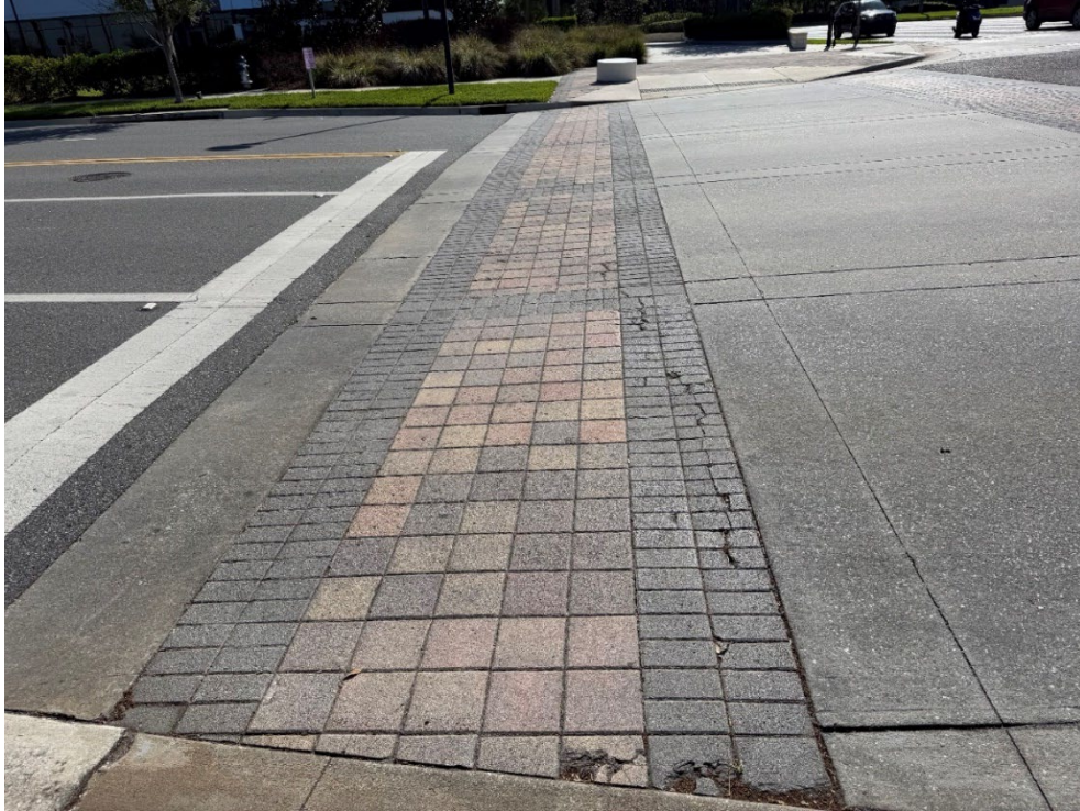
Photo 81 – Cracked and Broken Pavers, Some Settling (No Observed Changes) (Refer to Prior Photo 108 - 2025 Assessment)
