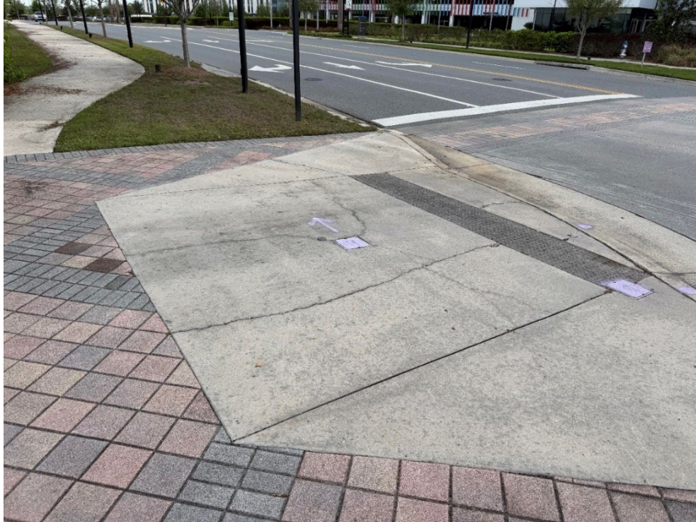
Photo 18 – Surficial Concrete Cracks in Handicap Ramp (No Observed Changes) (Refer to Prior Photo 22- 2025 Assessment)
