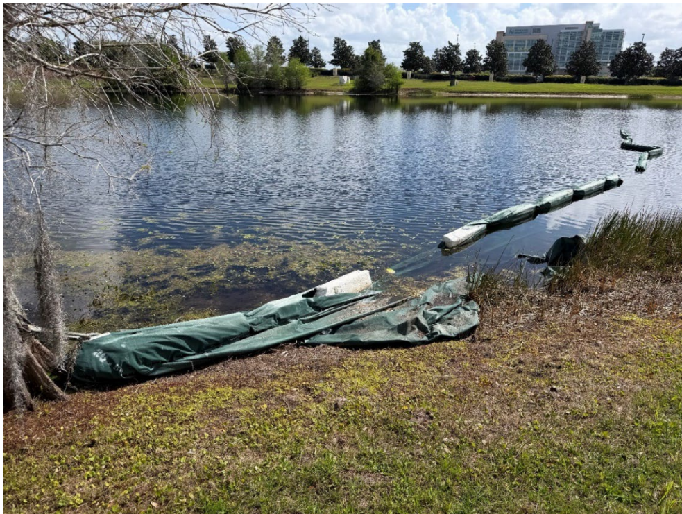
Photo 60 – Detached and Broken Floating Turbidity Barrier (No Observed Changes) (Refer to Prior Photo 79- 2025 Assessment)
