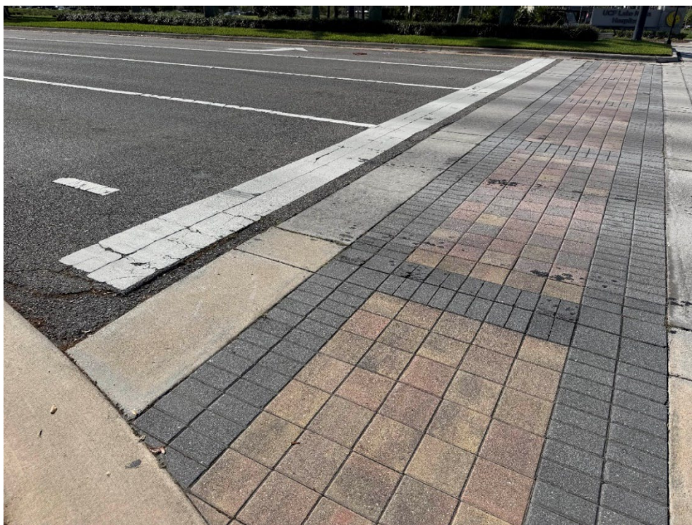
Photo 84 – Broken Concrete Flush Curb (No Observed Changes) (Refer to Prior Photo 111 - 2025 Assessment)
