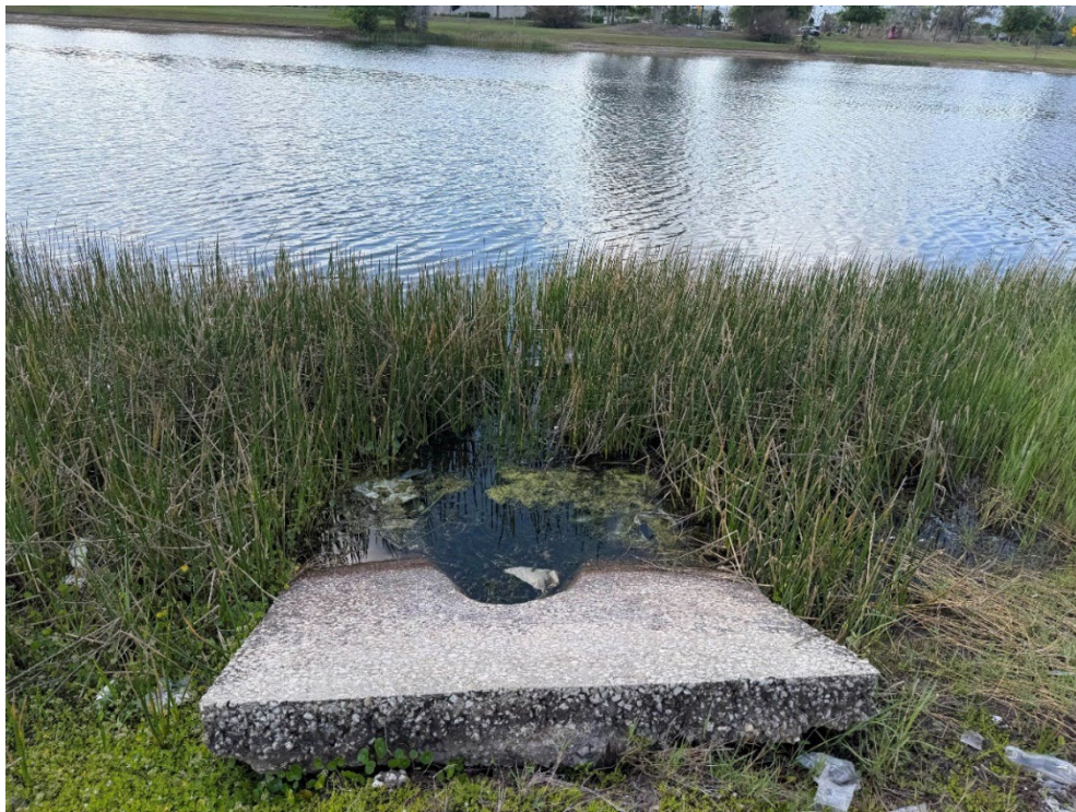
Photo 57.2 – Discharge Into Pond (New Photo – 2026 Assessment)
