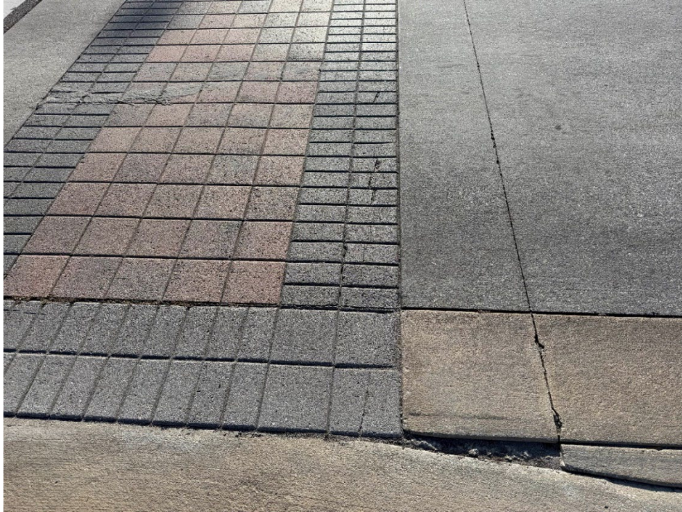
Photo 71 – Cracked Pavers, Minor Settling (No Observed Changes) (Refer to Prior Photo 91- 2025 Assessment)
