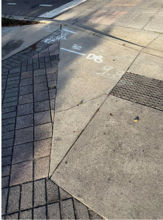
Photo 41 – Surficial Concrete Cracks in Handicap Ramp (No Observed Changes) (Refer to Prior Photo 49- 2025 Assessment)
