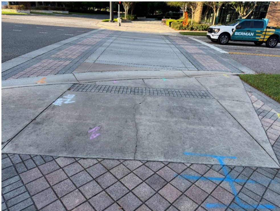
Photo 40 – Surficial Concrete Cracks in Handicap Ramp (No Observed Changes) (Refer to Prior Photo 48- 2025 Assessment)
