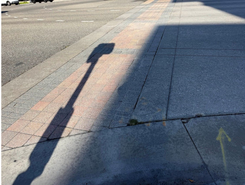
Photo 76 – Cracked Pavers, Broken Concrete (No Observed Changes) (Refer to Prior Photo 98 - 2025 Assessment)
