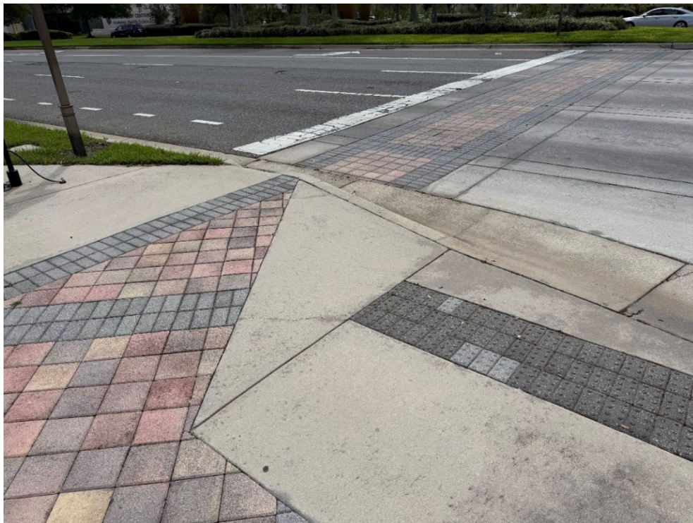
Photo 25 – Surficial Concrete Cracks in Handicap Ramp (No Observed Changes) (Refer to Prior Photo 32- 2025 Assessment)
