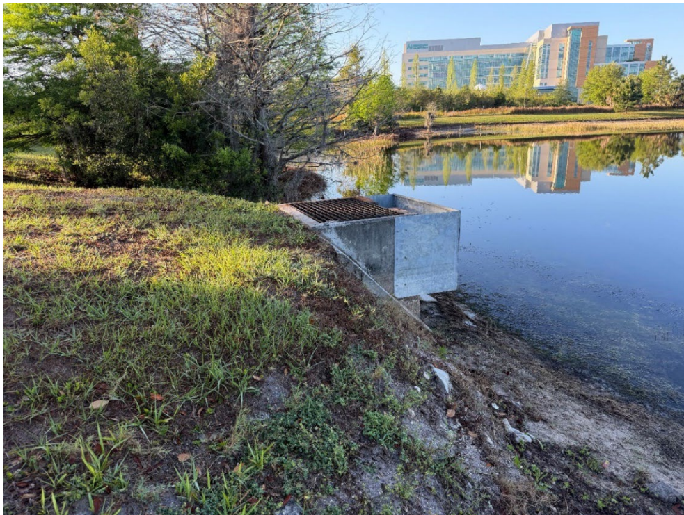
Photo 68 – Outfall Structure in Good Condition (No Observed Changes) (Refer to Prior Photo 88 - 2025 Assessment)
