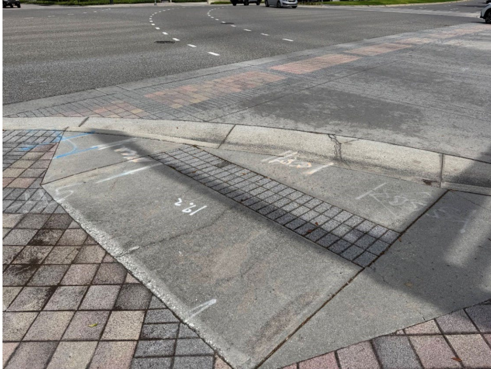
Photo 28 – Surficial Concrete Cracks in Handicap Ramp (No Observed Changes) (Refer to Prior Photo 35- 2025 Assessment)
