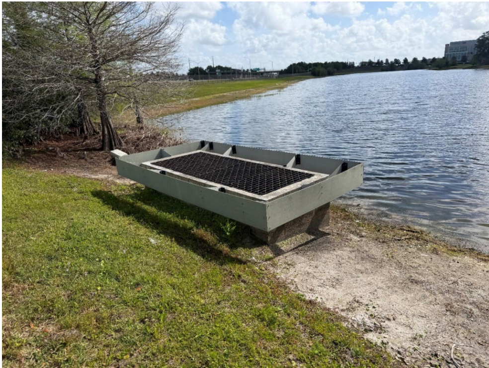
Photo 55 – Pond Outfall Structure in Good Condition (No Observed Changes) (Refer to Prior Photo 73- 2025 Assessment)
