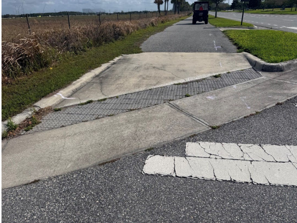
Photo 10 – Surficial Concrete Cracks in Handicap Ramp (No Observed Changes) (Refer to Prior Photo 13- 2025 Assessment)
