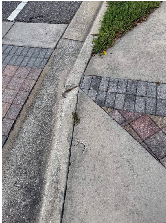
Photo 19 – Cracked and Spalling Concrete in Handicap Ramp (No Observed Changes) (Refer to Prior Photo 23- 2025 Assessment)
