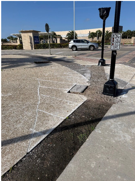
Photo 52.2 – Concrete Work Unfinished (New Photo – 2026 Assessment)
