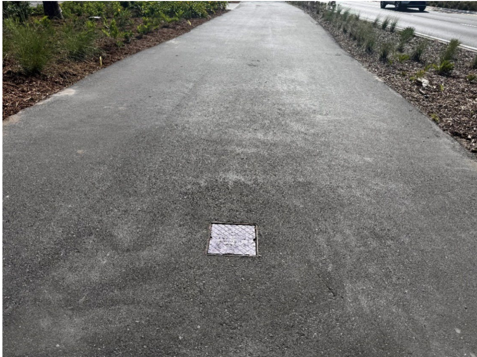
Photo 5 – Sunken Reclaim Water Meter (No Observed Changes) (Refer to Prior Photo 6- 2025 Assessment)
