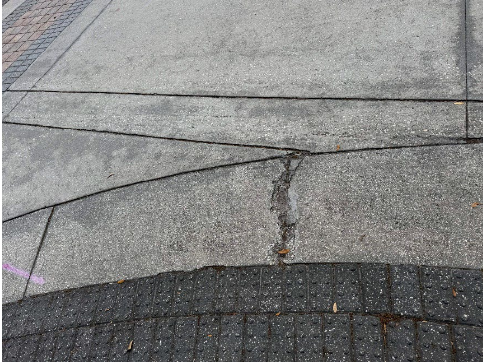
Photo 89 – Construction Entrance – Broken Concrete in Flush Curb (No Observed Changes) (Refer to Prior Photo 120 - 2025 Assessment)
