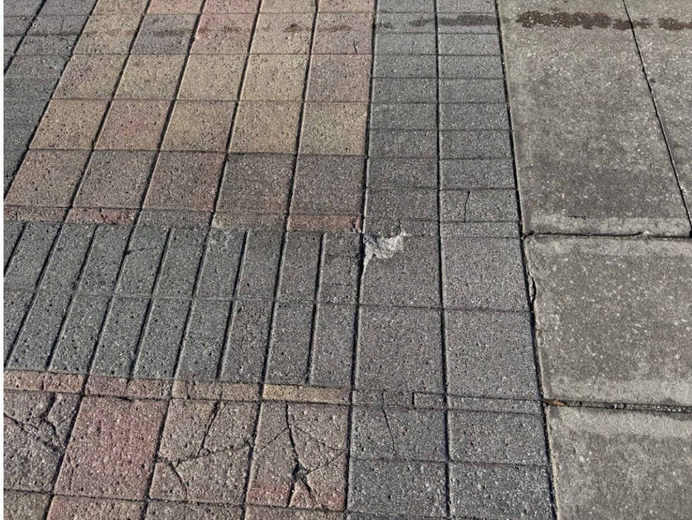
Photo 73 – Cracked Pavers, Minor Settling (No Observed Changes) (Refer to Prior Photo 95 - 2025 Assessment)
