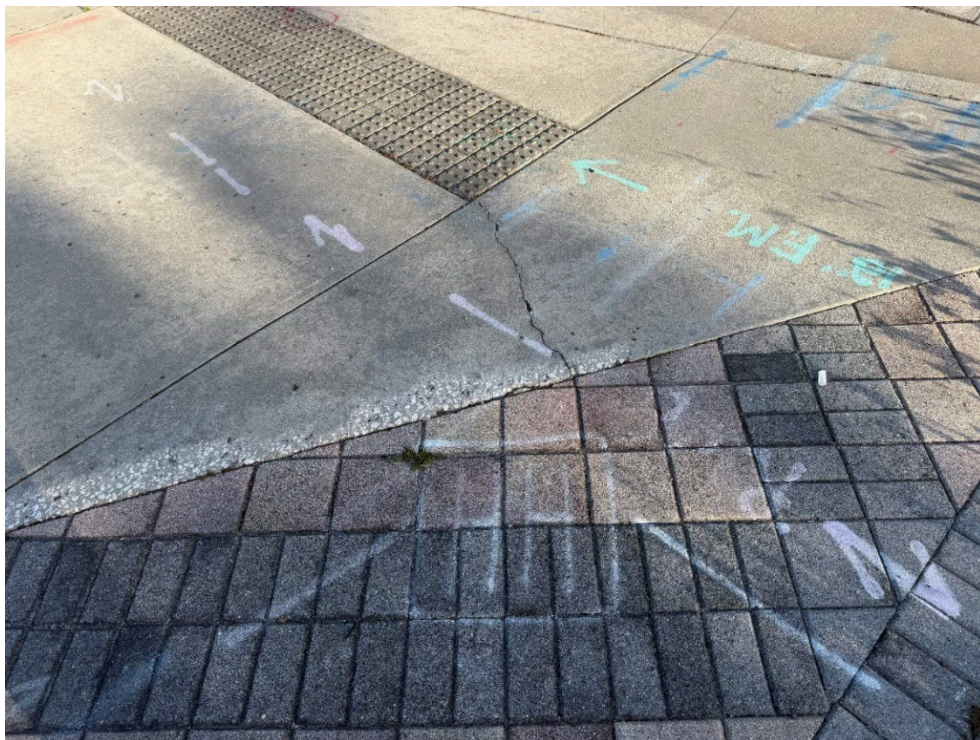
Photo 42 – Surficial Concrete Cracks in Handicap Ramp (No Observed Changes) (Refer to Prior Photo 51- 2025 Assessment)
