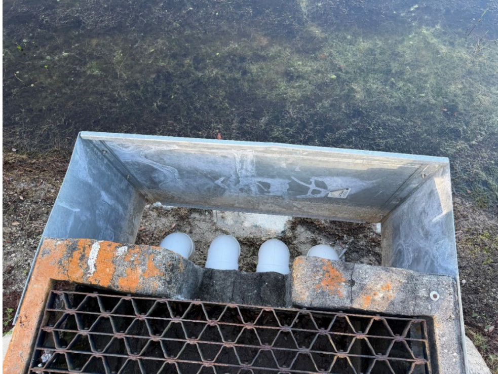
Photo 69 – Drawdown Pipe Inside of Outfall Structure (No Observed Changes) (Refer to Prior Photo 89- 2025 Assessment)
