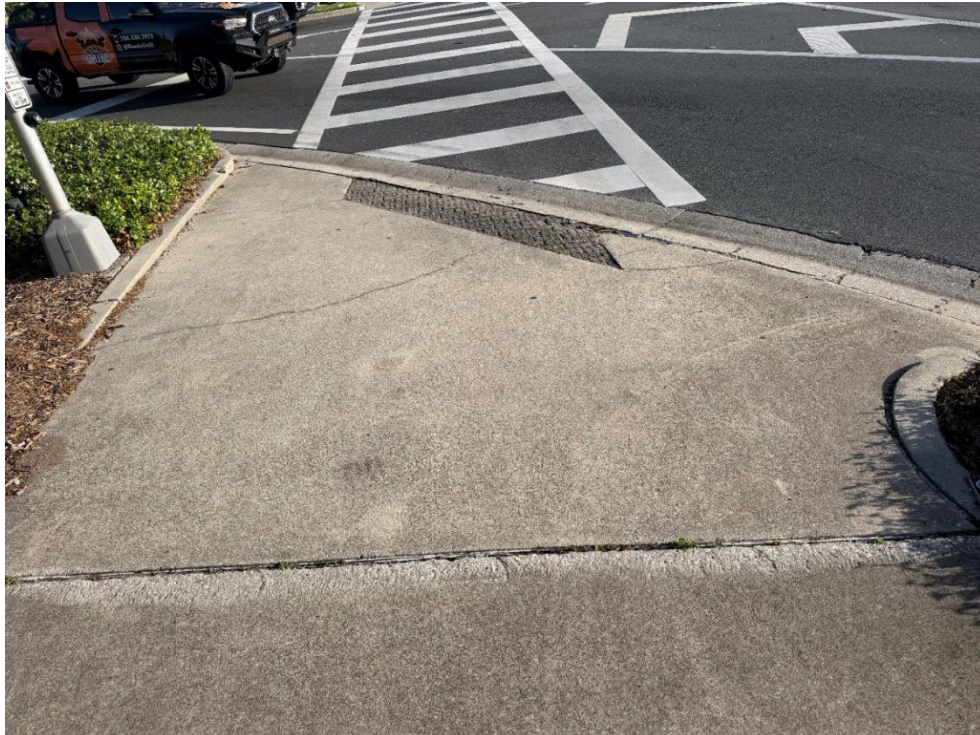
Photo 45 – Surficial Concrete Cracks in Handicap Ramp in Median (No Observed Changes) (Refer to Prior Photo 55- 2025 Assessment)
