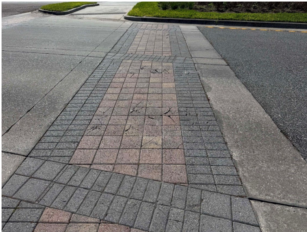
Photo 85 – Multiple Cracked Concrete, Pavers Settling, Broken Flush Curb (No Observed Changes) (Refer to Prior Photo 113 - 2025 Assessment)
